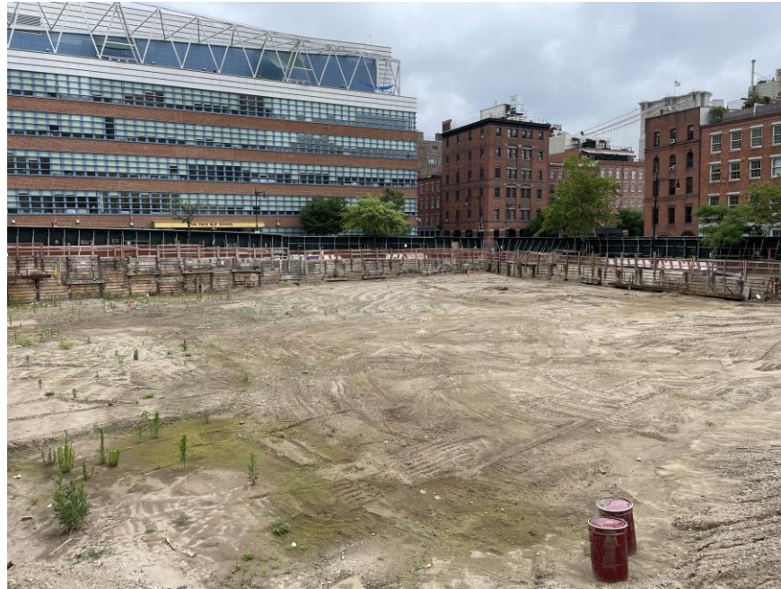
Photo 1: General view of the site (facing east)
