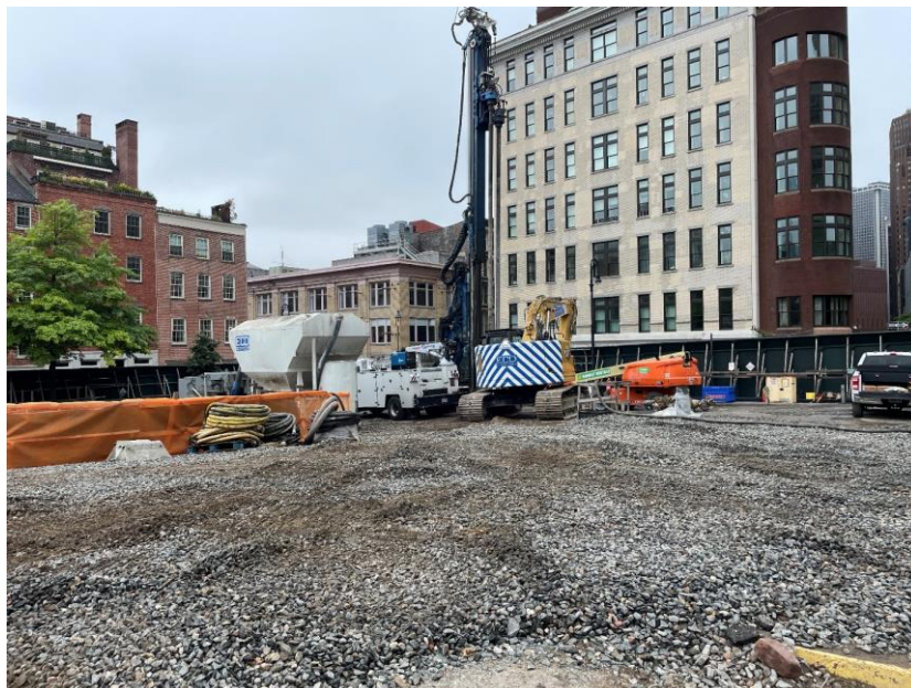
Photo 2: ECD mobilizing equipment to the site (facing southwest)
