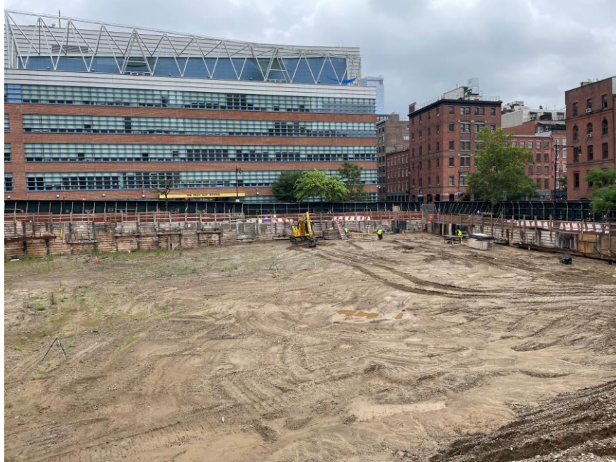
Photo 1: General view of the site (facing east)
