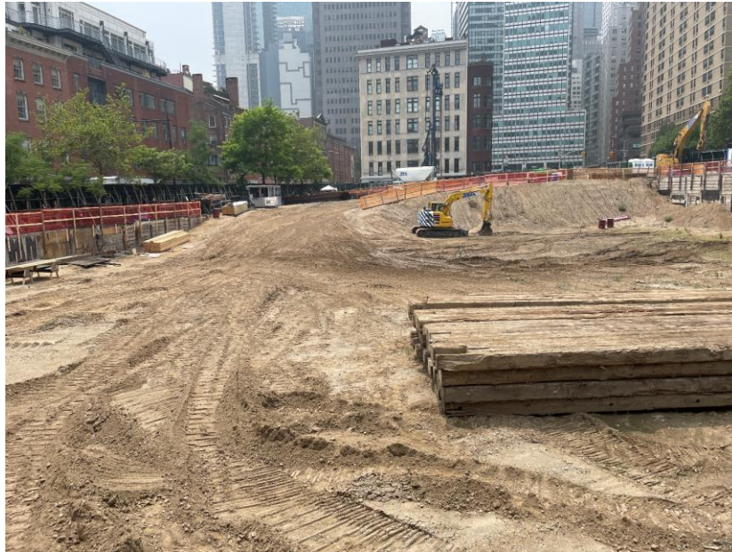
Photo 1: General view of the site (facing west)
