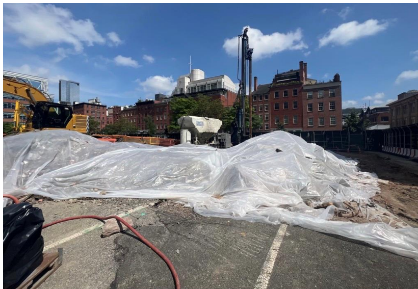
Photo 2: Soil/fill stockpile on and covered with polyethylene sheeting in the northwestern part of the site (facing south)
