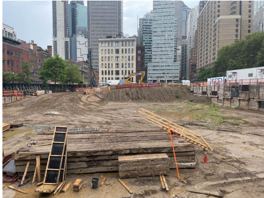
Photo 1: General view of the site (facing west)
