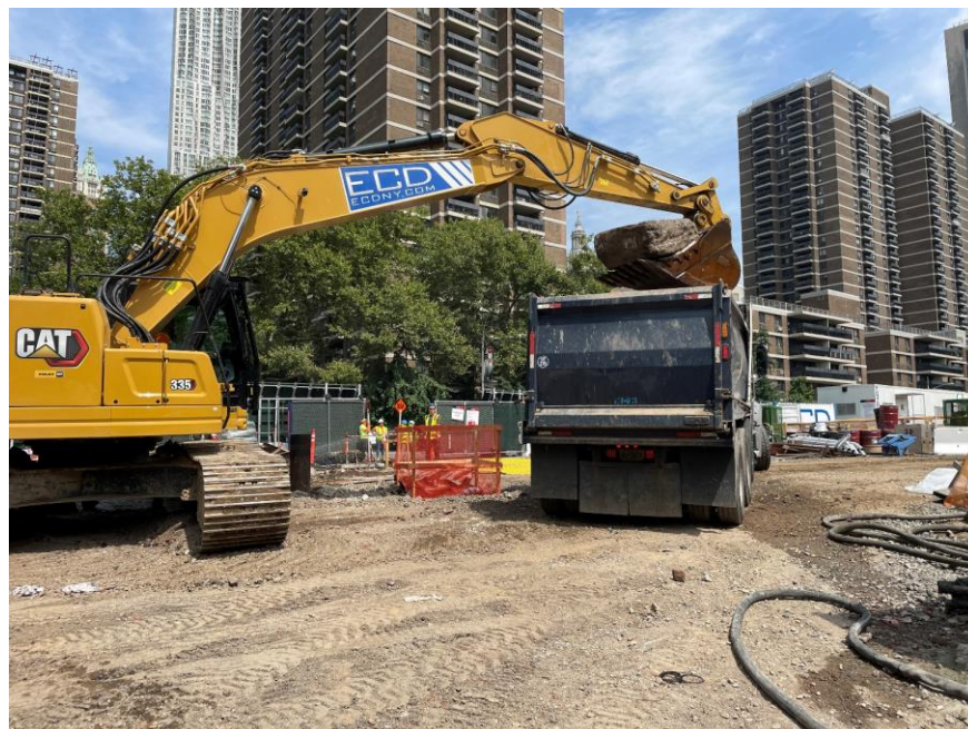
Photo 2: ECD exporting C&D debris from the western part of the site for off-site disposal (facing northeast)
