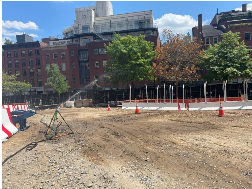
Photo 2: Dust suppression in the central part of the site (facing south)
