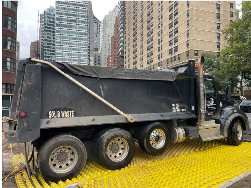
Photo 1: Securely covered dump truck prior to exiting the site (facing northwest)
