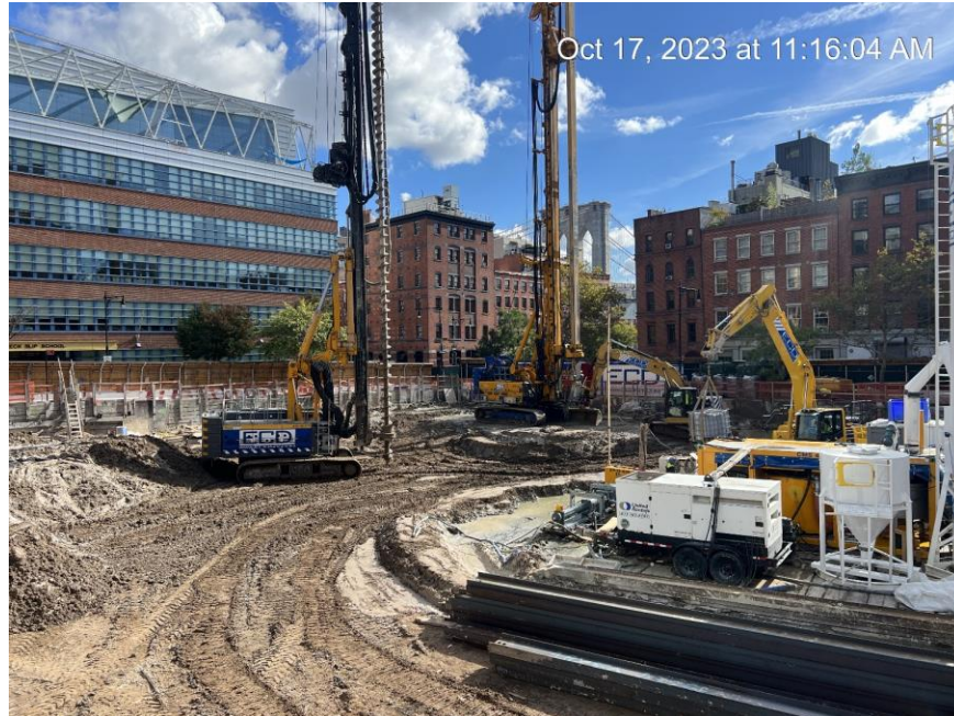
Photo 1: General view of the site (facing east)
