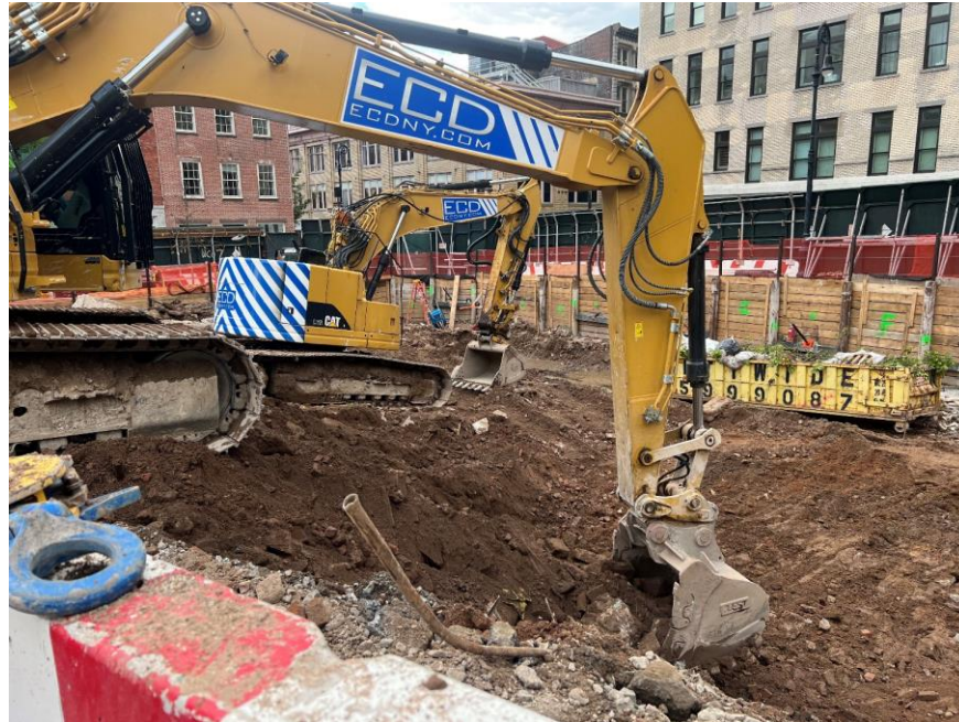
Photo 1: ECD excavating soil/fill in the western part of the site (facing southeast)
