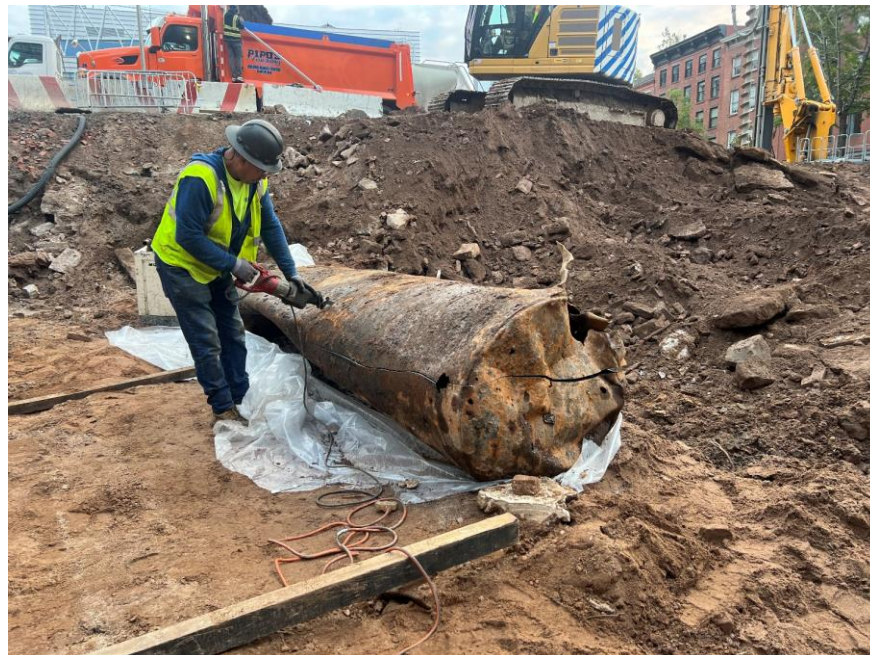
Photo 2: IRT decommissioning a UST prior to off-site disposal (facing southeast)
