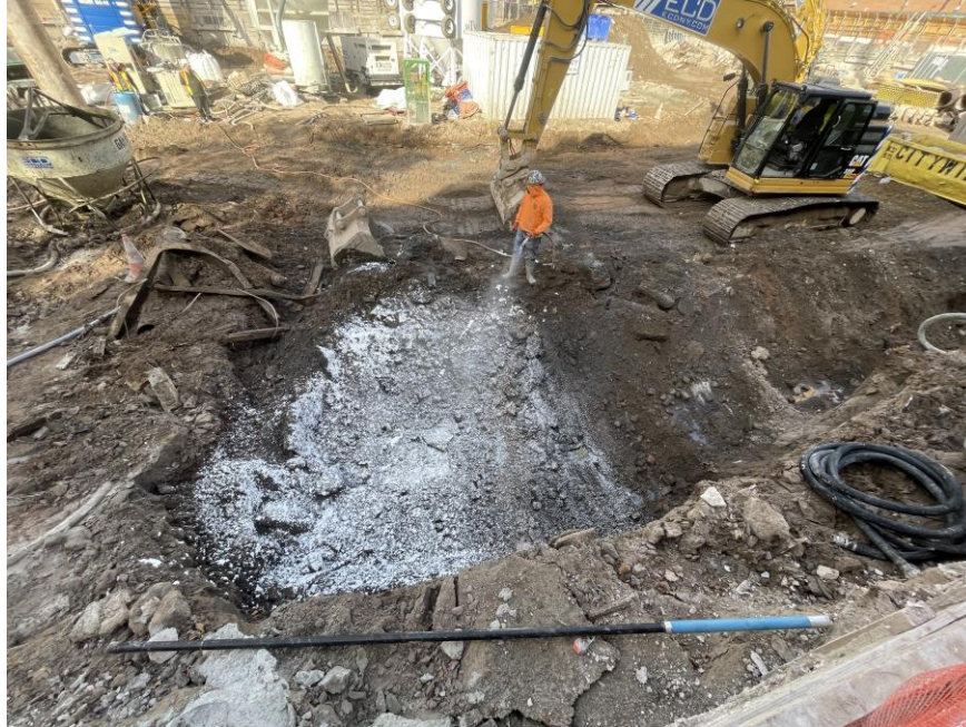
Photo 1: ECD applying Atmos AC-645 odor/vapot suppressing foam to soil/fill in the southern part of the site (facing northwest).
