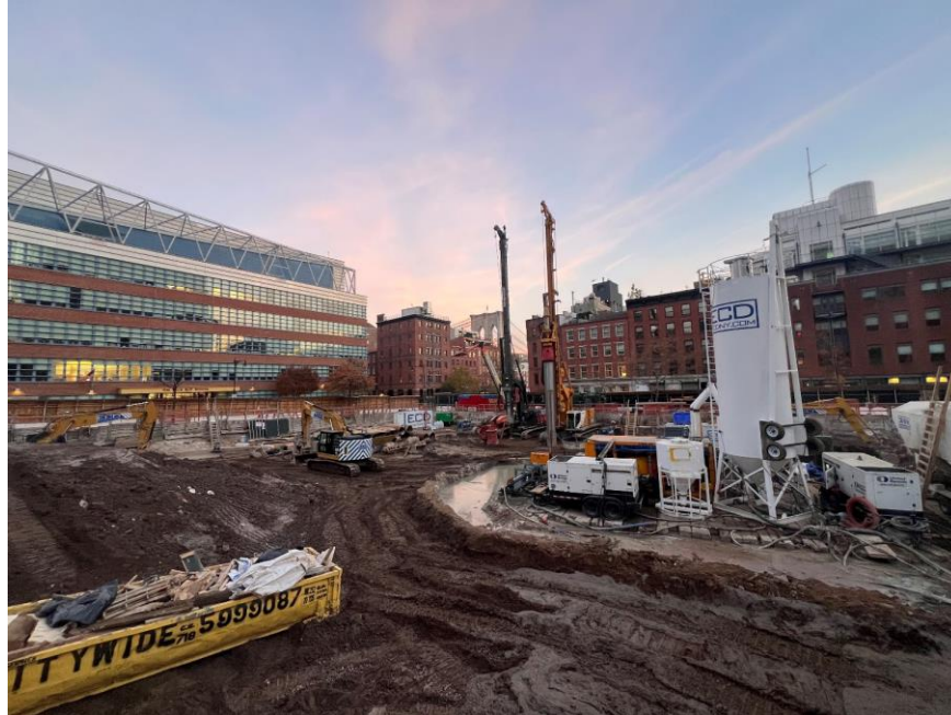
Photo 1: General view of the eastern part of site (facing southeast)
