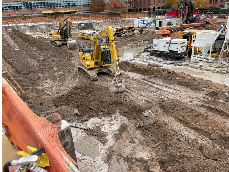
Photo 1: ECD grading soil/fill in the northeast part of site (facing southeast)
