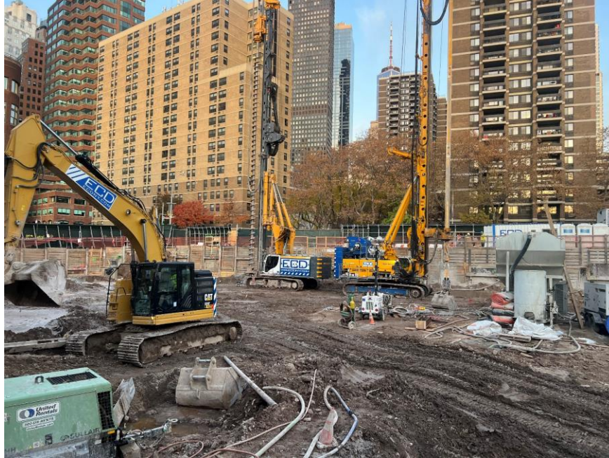
Photo 1: General view of the western part of site (facing north)
