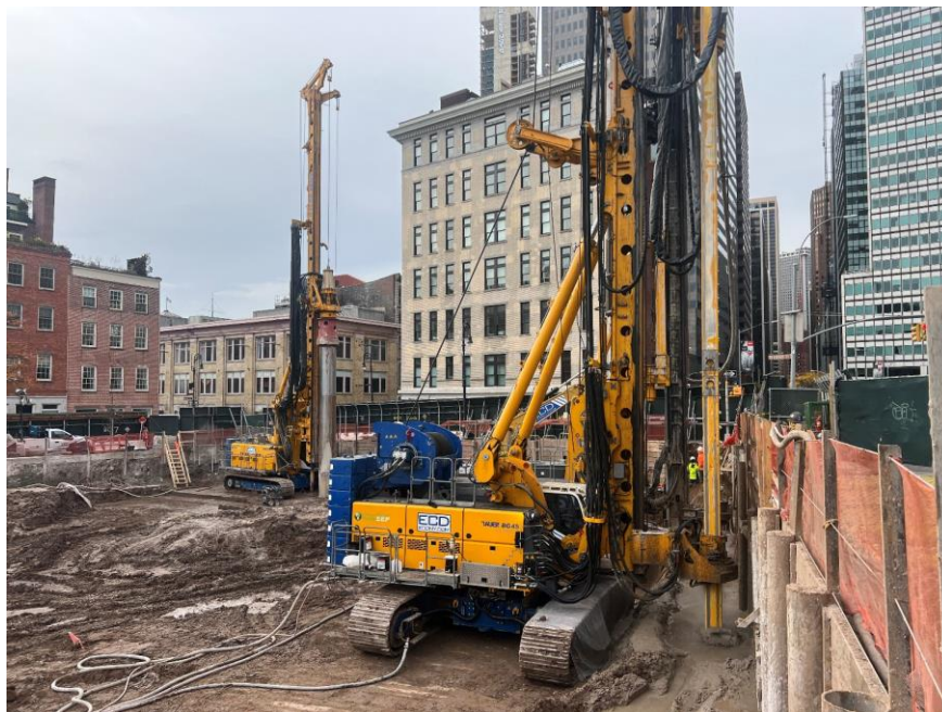
Photo 2: ECD installing a soil mix column in the northern part of site (facing west)
