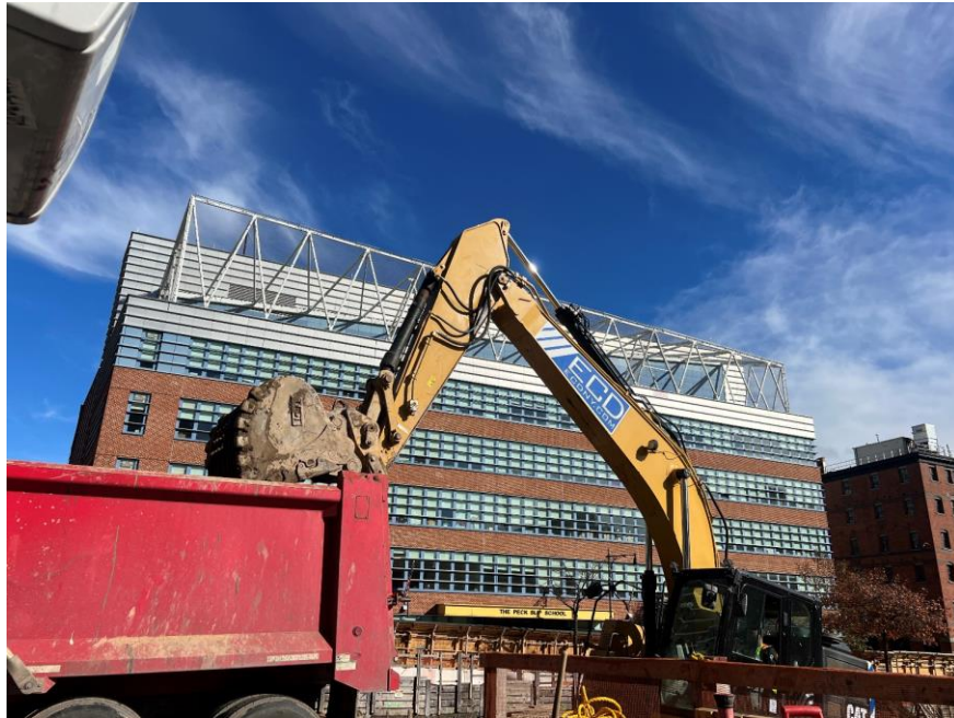
Photo 1: ECD loading a truck with C&D debris for off-site disposal (facing east)
