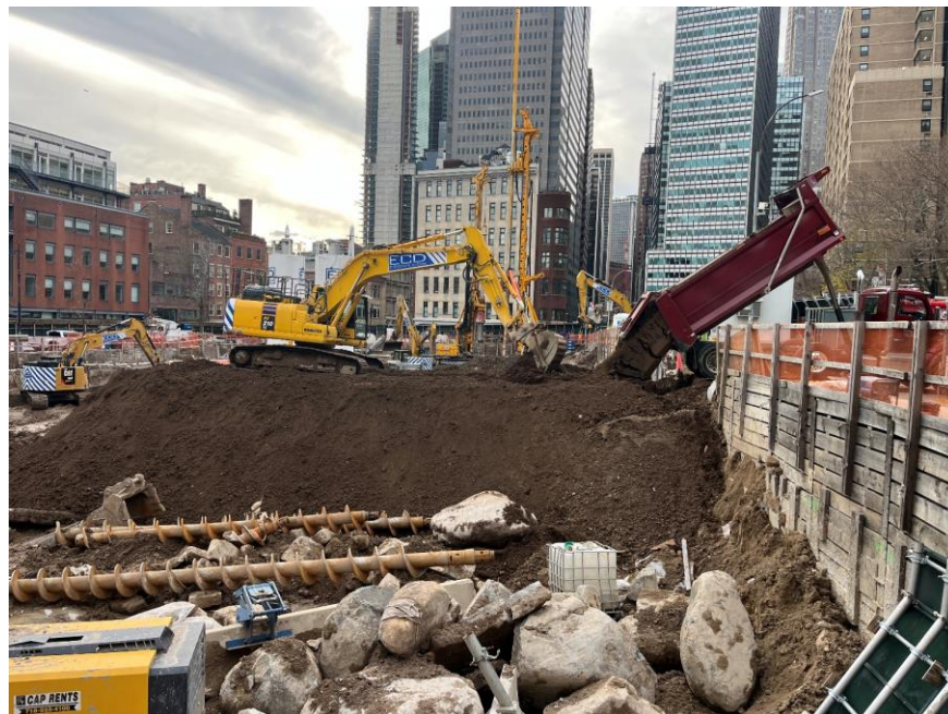
Photo 2: ECD importing screened fill (facing southwest)
