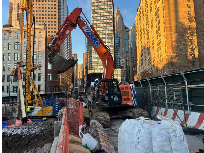
Photo 1: ECD loading a truck with soil/fill for off-site disposal (facing west)
