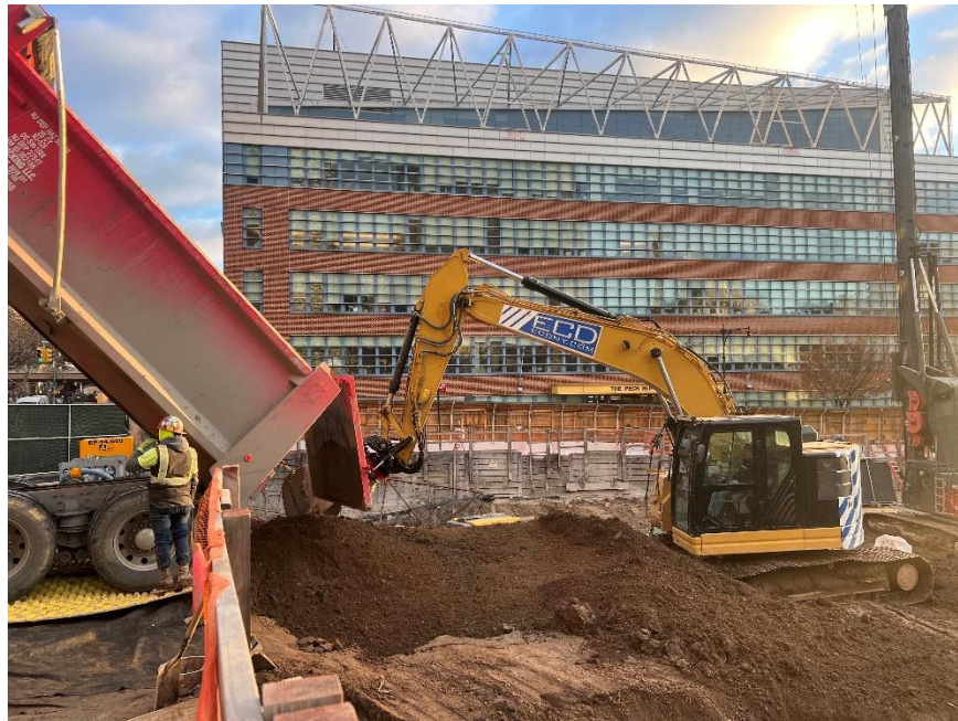
Photo 2: ECD importing screened fill to the site (facing east)
