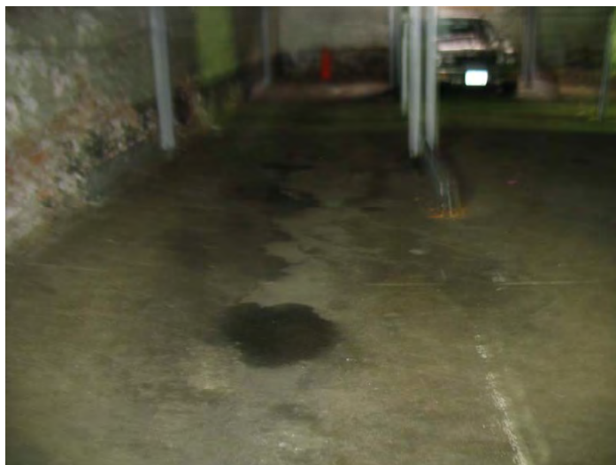
Photograph 5: Staining inside parking garage.
