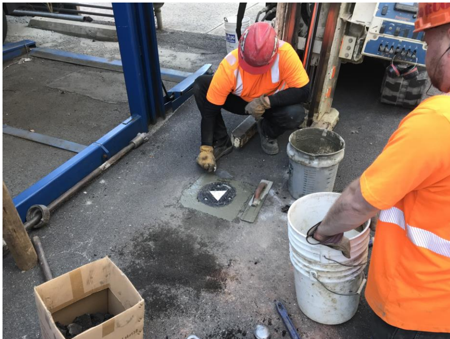
Photo 4, 4/23/2018: View of AARCO installing a monitoring well (facing northwest).
