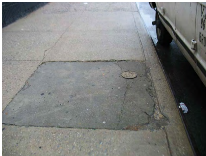
Photograph 7: Potential fill port for historical underground storage tanks.
