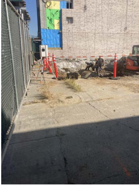
5. Excavation area overview, begin cutting, entering, and cleaning USTs.
