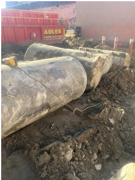
11. Final set of USTs located, contents removed, and staged for recycling.
