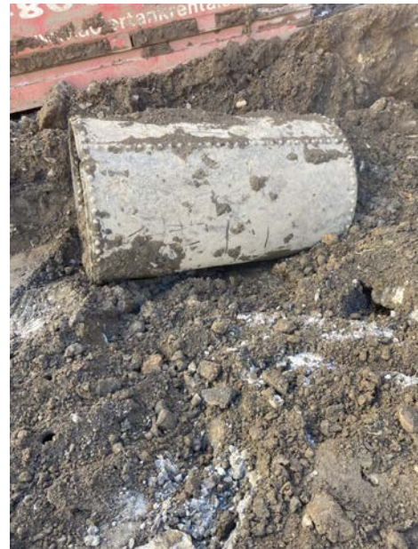
12. Example of riveted UST encountered.
