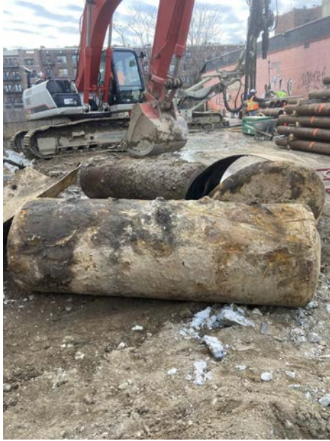
9. Additional USTs staged for future recycling.
