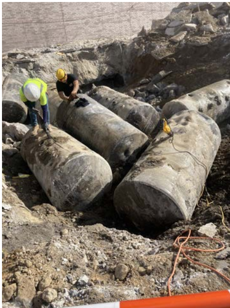
7. USTs staged, cut open, and contents emptied.
