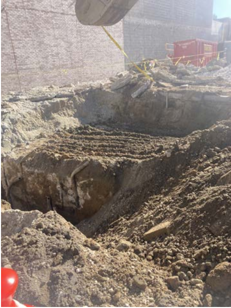
1. Begin removing concrete and overburden soils above USTs
