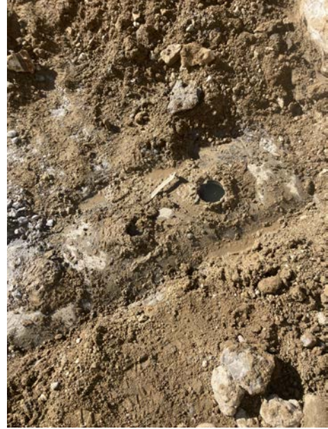
2. UST bung and top of UST exposed
