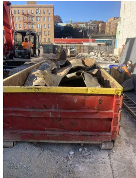
8. Cleaned UST shells recycled as scrap emptied.
