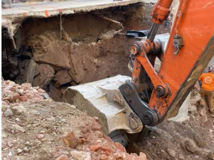
Photo 1: Mayrich excavating non-hazardous historic fill and native soil in the northern part of the site for SOE installation (facing north).
