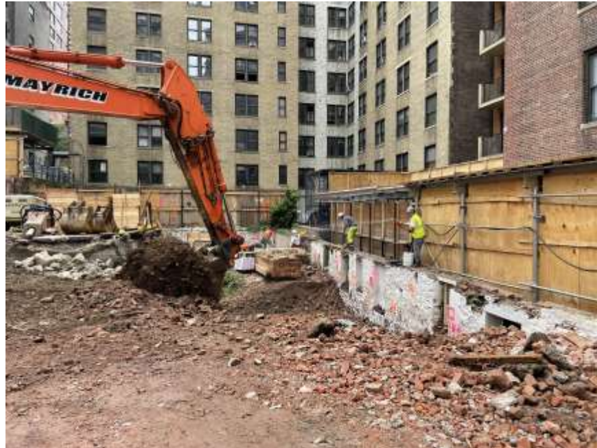
Photo 1: Mayrich using dust suppression during removal of C&D debris in the southwestern part of the site (facing south).
