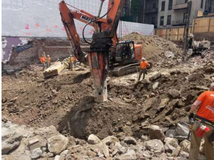
Photo 1: Mayrich applying dust suppression while breaking concrete in the northern part of the site (facing southeast).
