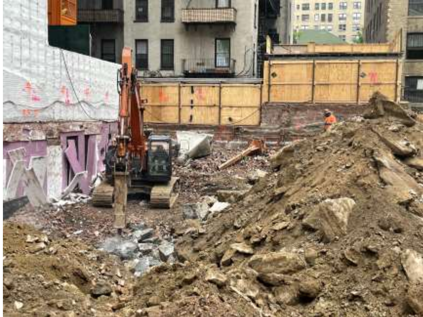
Photo 1: Mayrich using dust suppression while breaking concrete slab in the southeastern part of the site (facing south).
