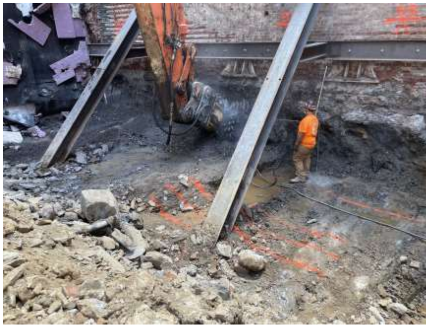
Photo 2: Mayrich using dust suppression while chipping bedrock in the southeastern part of the site (facing southeast)
