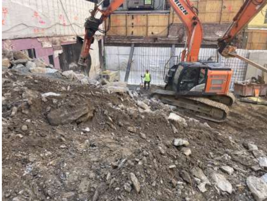
Photo 2: Mayrich using dust suppression while breaking concrete in the southeastern part of the site (facing south).
