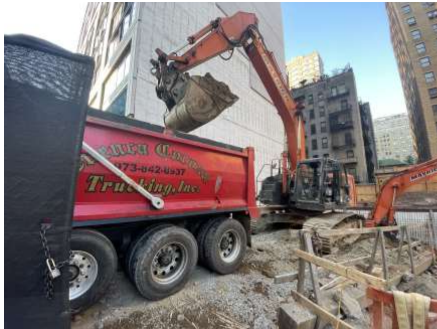
Photo 1: Mayrich exporting non-hazardous fill and native soil for off-site disposal (facing south)
