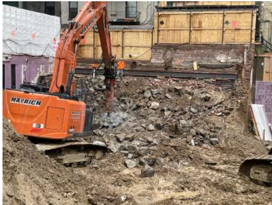
Photo 1: Mayrich applying dust suppression while breaking concrete in the southeastern part of the site (facing south)
