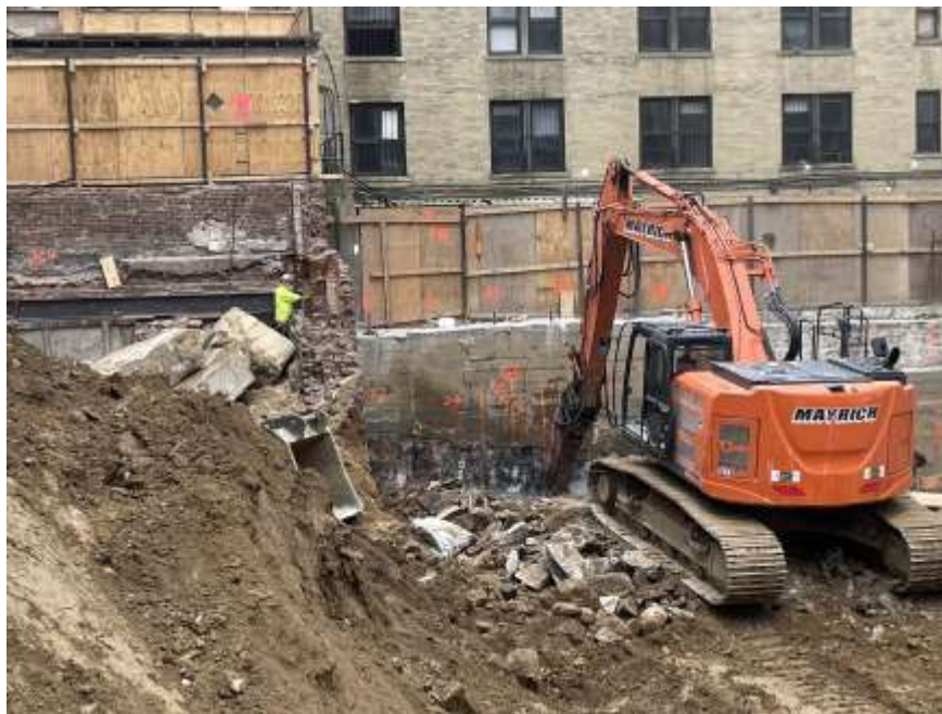
Photo 2: Mayrich applying dust suppression during bedrock chipping in the southwest part of the site (facing west).
