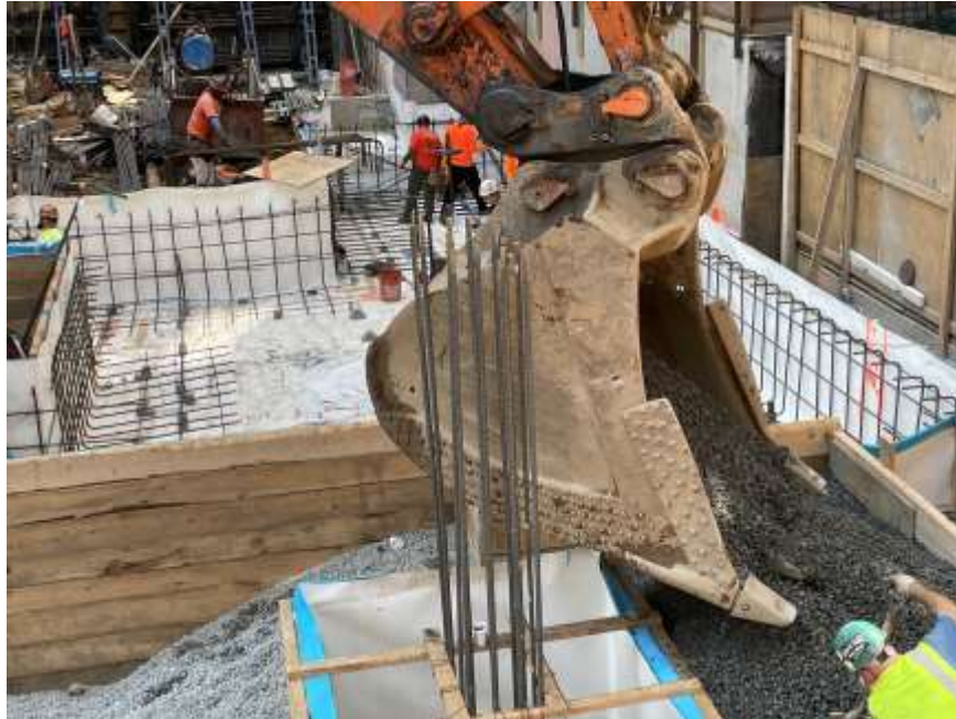
Photo 1: View of Mayrich temporarily backfilling around foundation elements with 0.75-inch stone in the northwestern part of the site, facing south.
