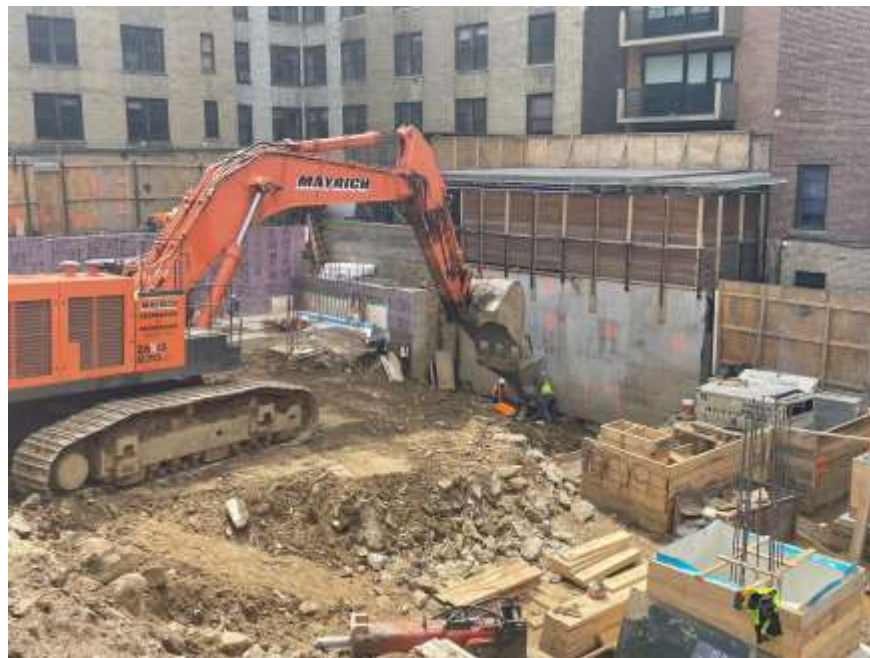
Photo 2: Mayrich excavating native soil along the western site boundary of the site for underpinning installation (facing southwest).
