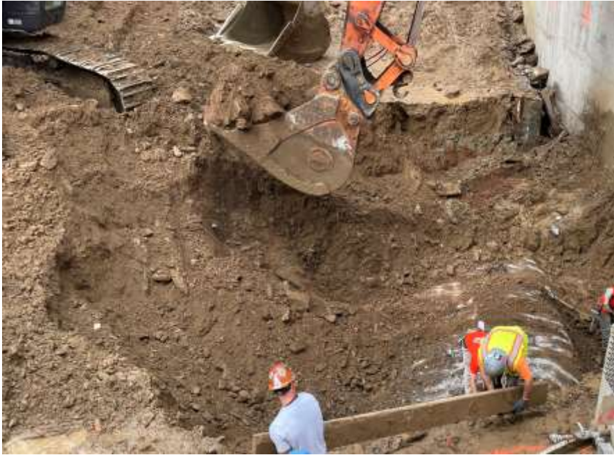
Photo 1: Mayrich excavated non-hazardous historic fill and native soil to bedrock in the northwestern part of the site (facing southwest).
