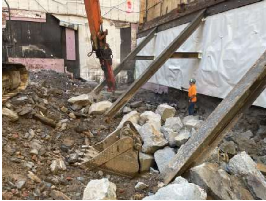
Photo 1: Mayrich using dust suppression while breaking concrete in the southeastern part of the site (facing east).
