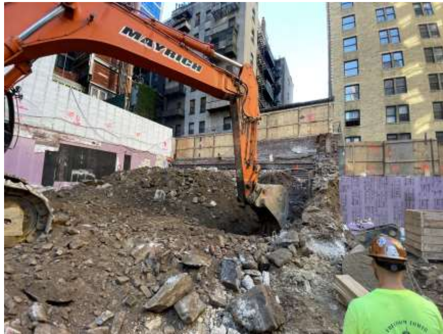
Photo 1: Mayrich excavating non-hazardous historic fill and C&D debris in the southeastern part of the site (facing southeast)
