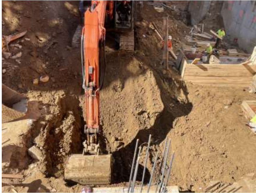
Photo 1: Mayrich excavating non-hazardous historic fill and native soil in the northwestern part of the site (facing south).
