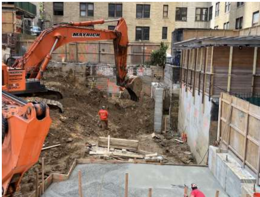
Photo 2: Mayrich excavating non-hazardous historic fill and native soil in the southwestern part of the site (facing south).
