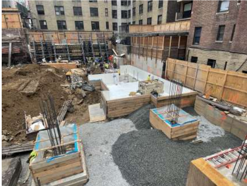
Photo 1: View of the area Mayrich backfilled with 0.75-inch stone in the northwestern part of the site, facing south.
