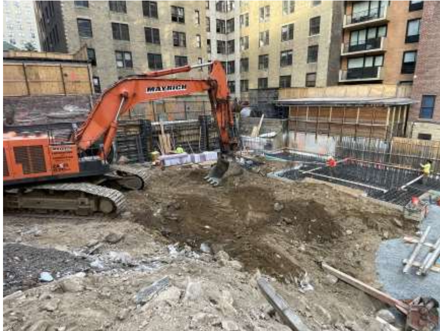
Photo 1: Mayrich grading non-hazardous historic fill in the northcentral part of the site (facing southwest).
