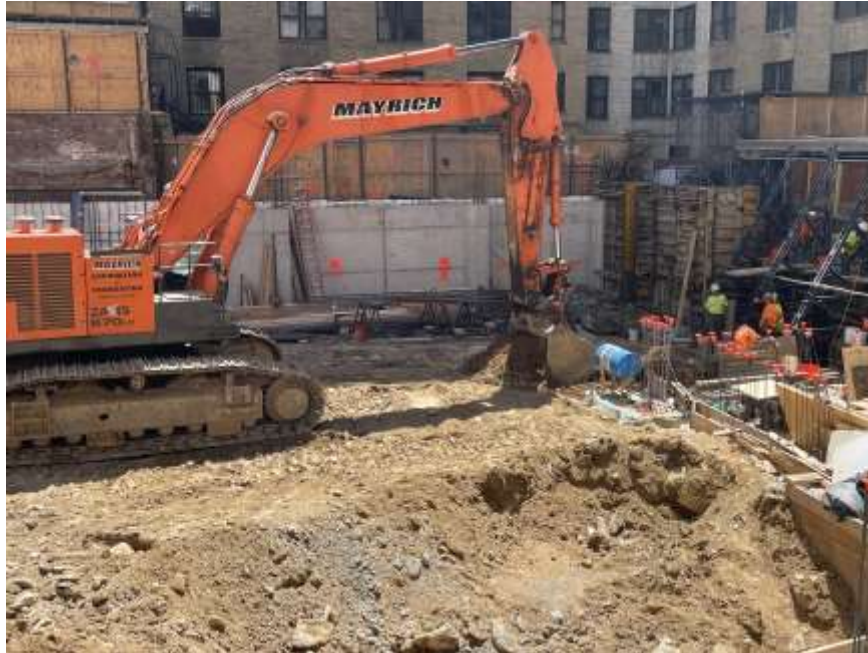
Photo 1: Mayrich excavating non-hazardous fill and native soil from the southwestern part of the site (facing south)
