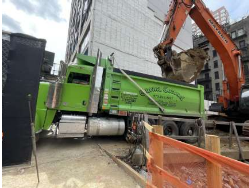
Photo 1: Mayrich exporting non-hazardous historic fill and native soil for off-site disposal (facing east).
