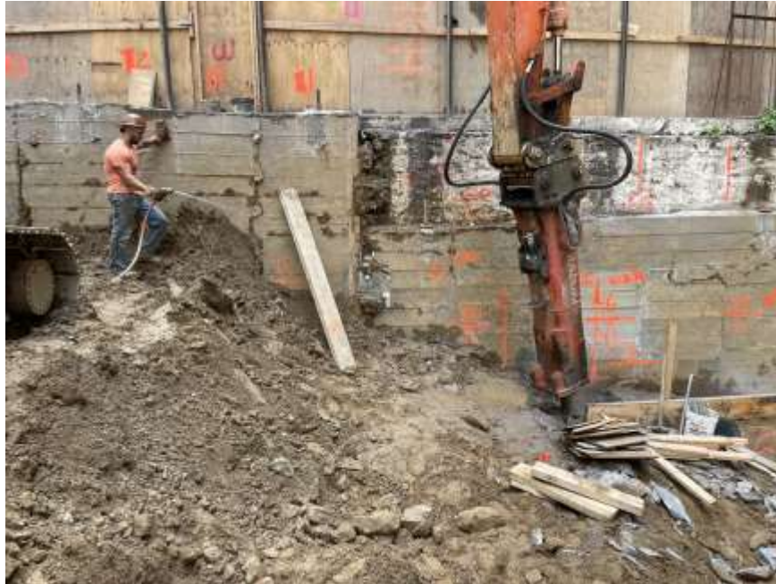
Photo 1: Mayrich applying dust suppression during bedrock chipping on the southwest part of the site (facing south)
