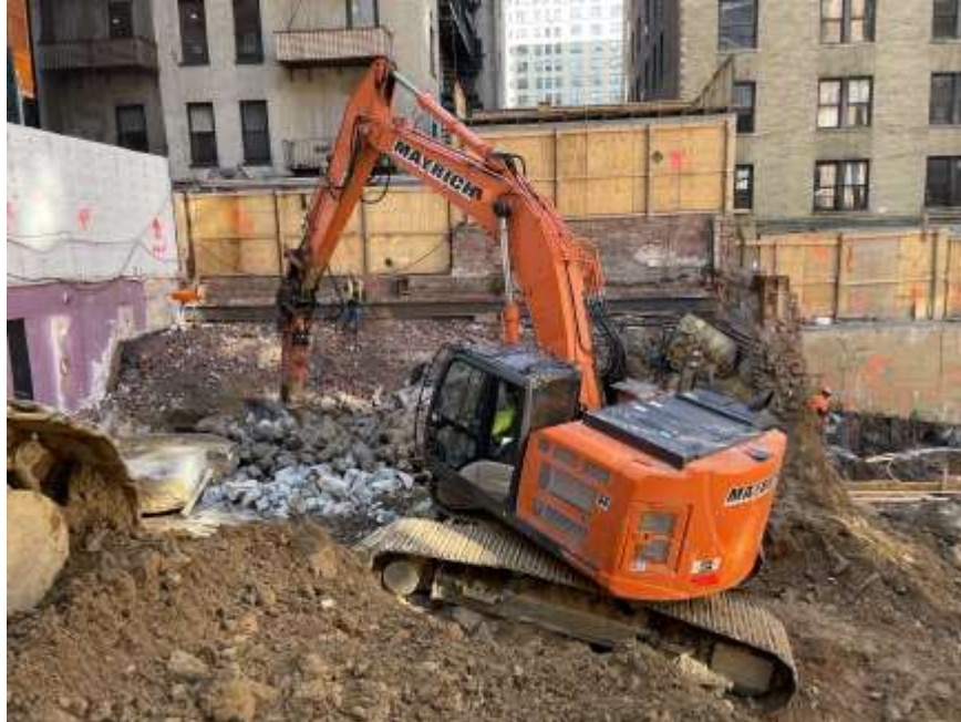
Photo 2: Mayrich applying dust suppression while breaking concrete in the southeastern part of the site (facing south).
