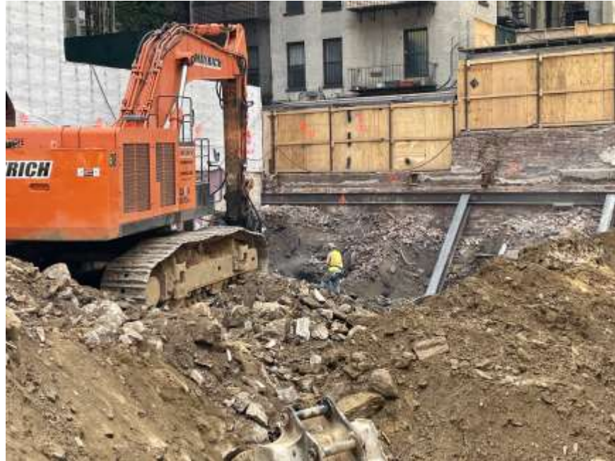
Photo 1: Mayrich using dust suppression while chipping bedrock in the southeastern part of the site (facing south)
