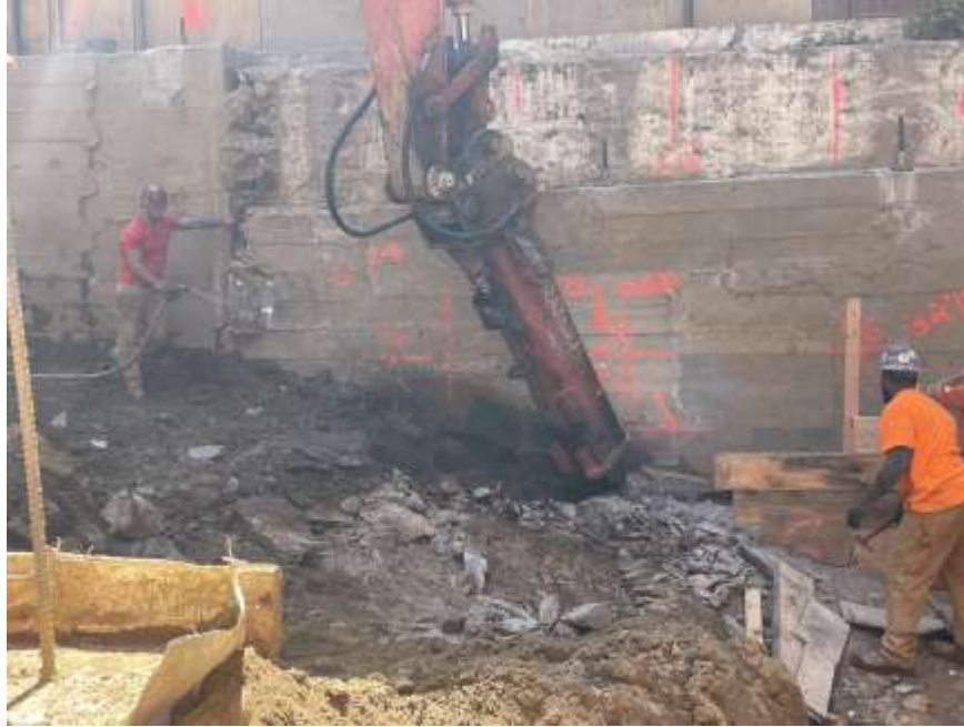
Photo 2: Mayrich applying dust suppression during bedrock chipping in the southwest part of the site (facing south).
