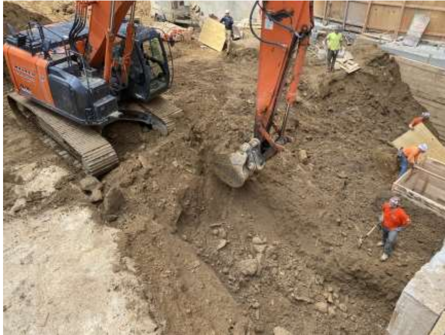
Photo 1: Mayrich excavating non-hazardous historical fill and native soil in the northwestern part of the site (facing southwest).
