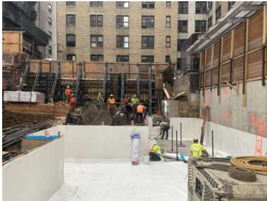
Photo 2: Mayrich installing waterproofing in the western part of the site (facing south)
