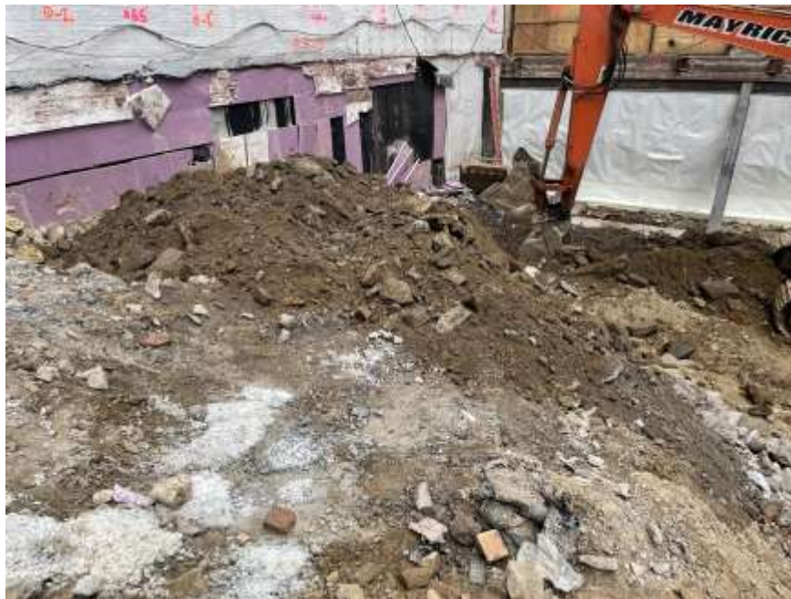
Photo 2: Mayrich excavating non-hazardous historic fill and chipped bedrock in the southeastern part of the site (facing south).
