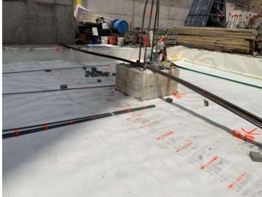
**Photo 1:** View of Mayrich installing waterproofing in the southwestern part of the site (facing west).
