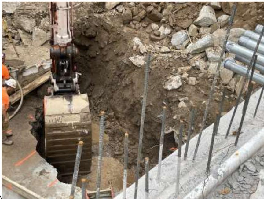
**Photo 2:** Mayrich removing chipped bedrock in the northeastern part of the site (facing south).
