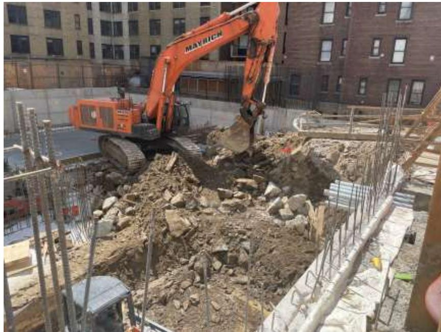
**Photo 2:** Mayrich excavating chipped bedrock in the northeastern part of the site (facing southwest).
