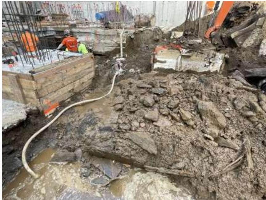
**Photo 1:** View of on-site components of the site's dewatering system in northwestern part of the site (facing west).
