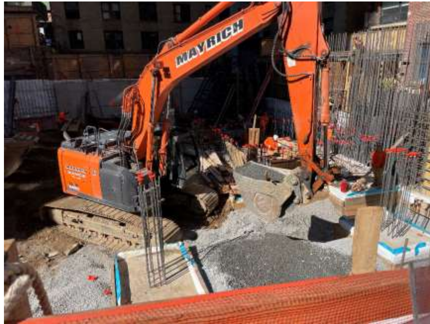
Photo 11: View of Mayrich removing 0.75-inch stone in the northwestern part of the site, facing south. Taken on 06/28/2022
