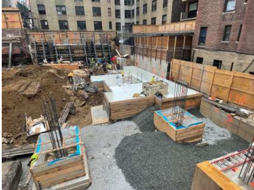
Photo 9: View of the area Mayrich temporarily backfilled with 0.75-inch stone to use as a construction entrance in the northwestern part of the site, facing south. Taken on 6/16/2022
