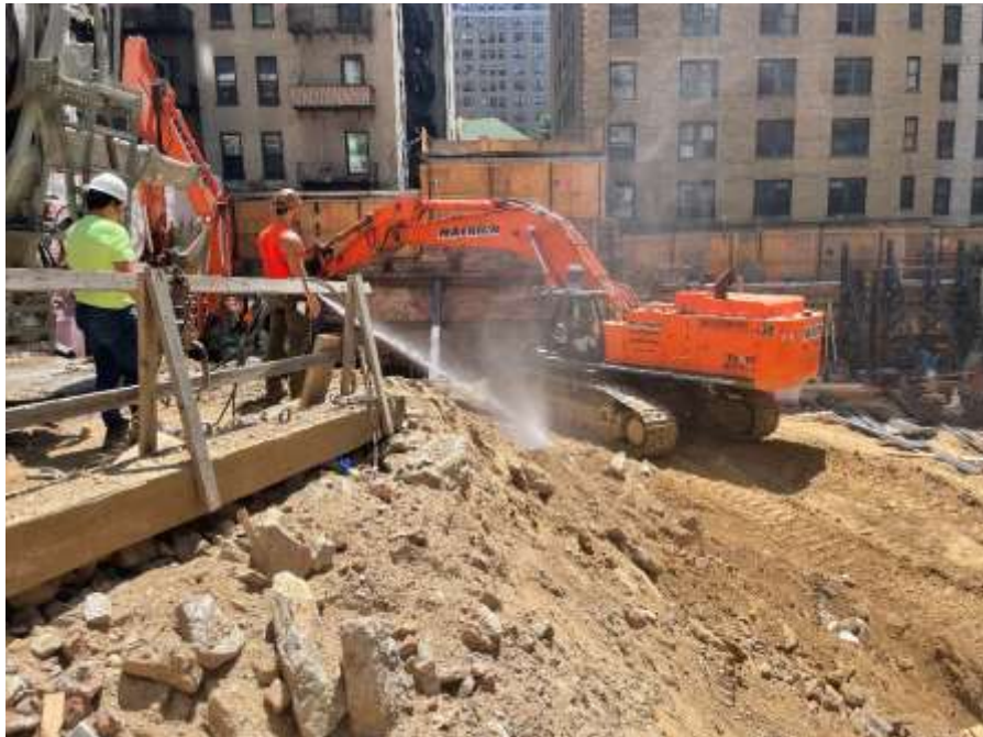
Photo 10: View of Mayrich apply water to mitigate dust on the central part of the site, facing south. Taken on 06/20/2022
