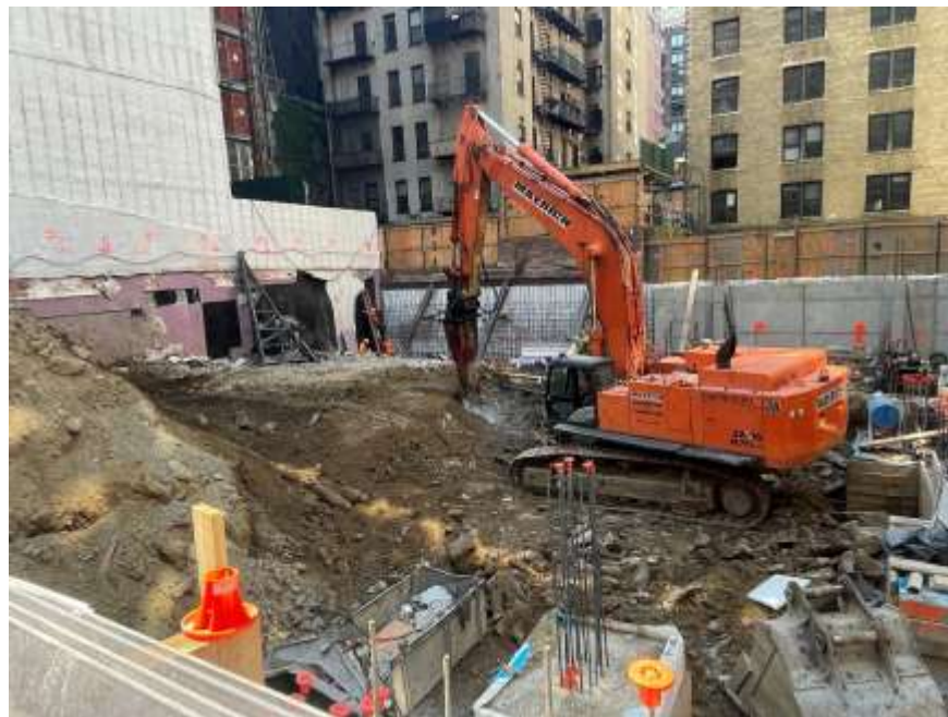
Photo 12: View of Mayrich chipping bedrock in central part of the site, facing southeast. Taken on 07/01/2022
