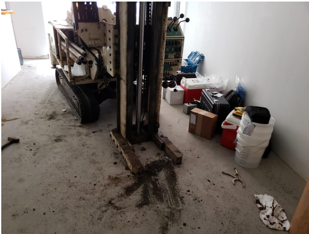
Photo 6, 6/1/2018: AARCO advancing soil boring SB4 using a Geoprobe 6610DT, facing north.
