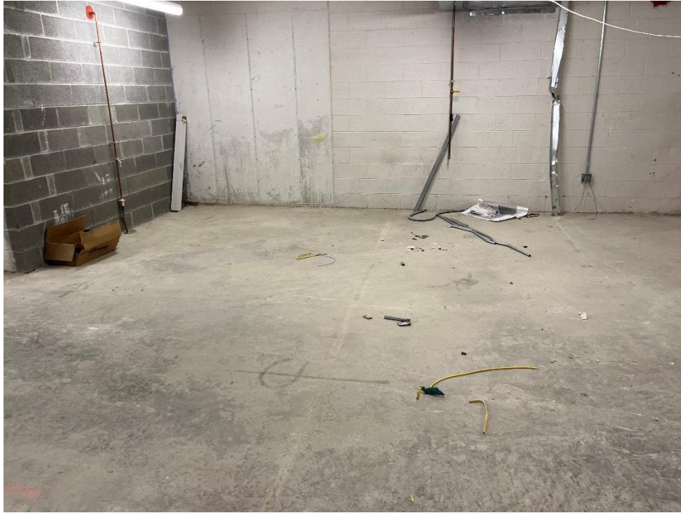
Photo 21, 01/17/2023: View of the cellar-level concrete building slab (facing east)
