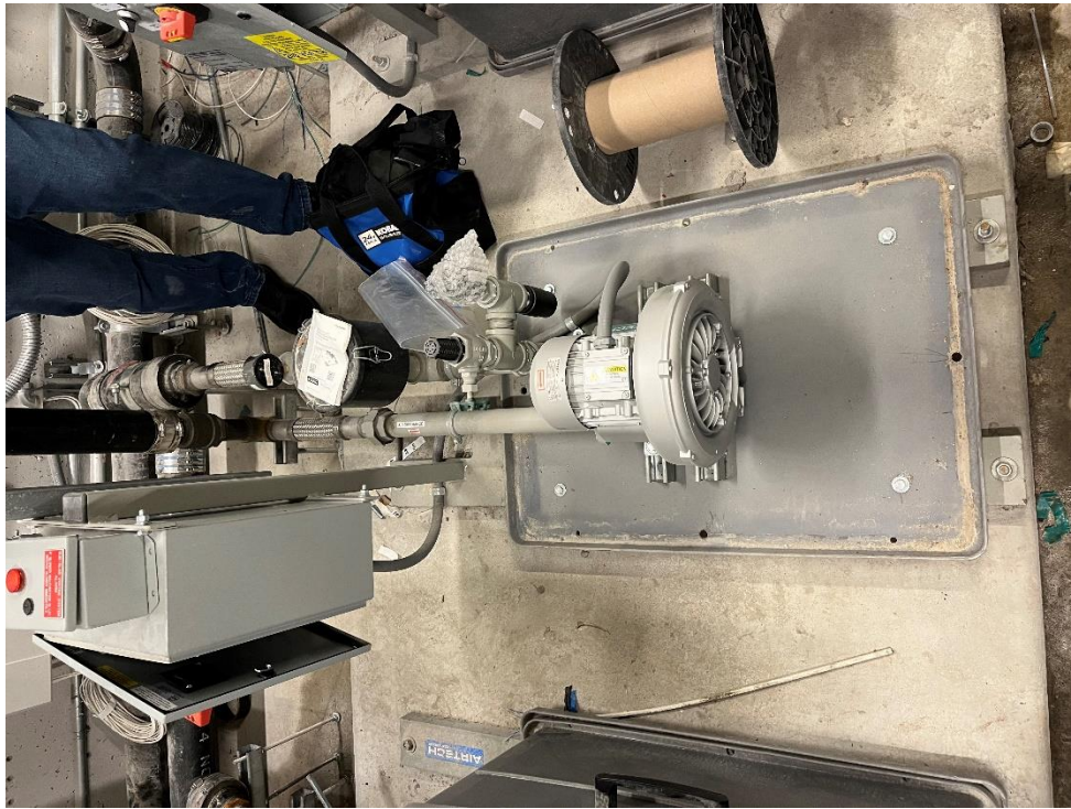
Photo 1, 01/04/2023: View of submembrane depressurization (SMD) system blowers being installed
