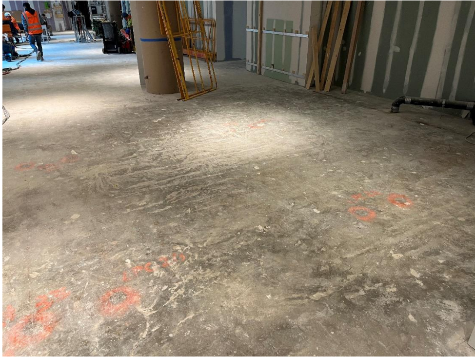
Photo 19, 01/04/2023: View of the first-floor concrete building slab (facing northeast)
