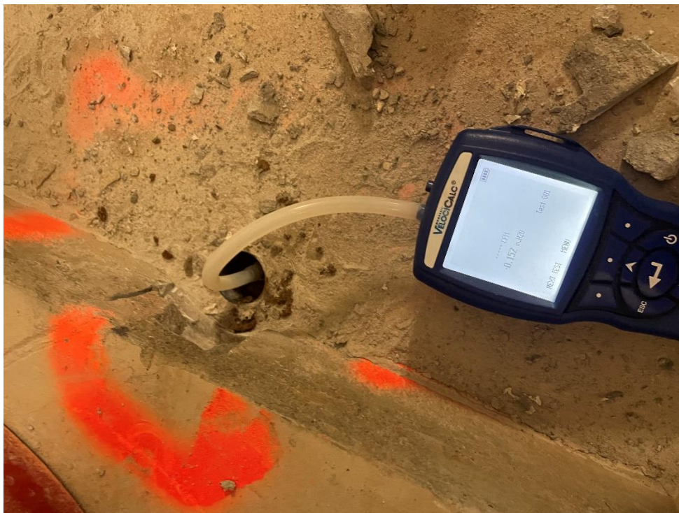
Photo 24, 04/25/2023: Langan collecting vacuum readings from vapor monitoring point VMP02
