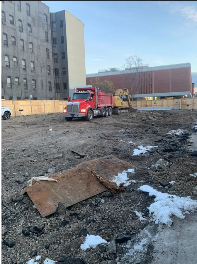
Photo 1 – View of trucking loading from SB-5 Hotspot for transport to Clean Earth of Carteret.
