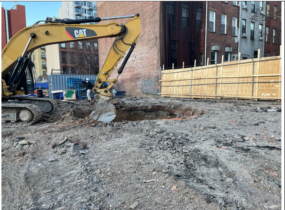
Photo 1 – View of SB-1 Hotspot Excavation.
