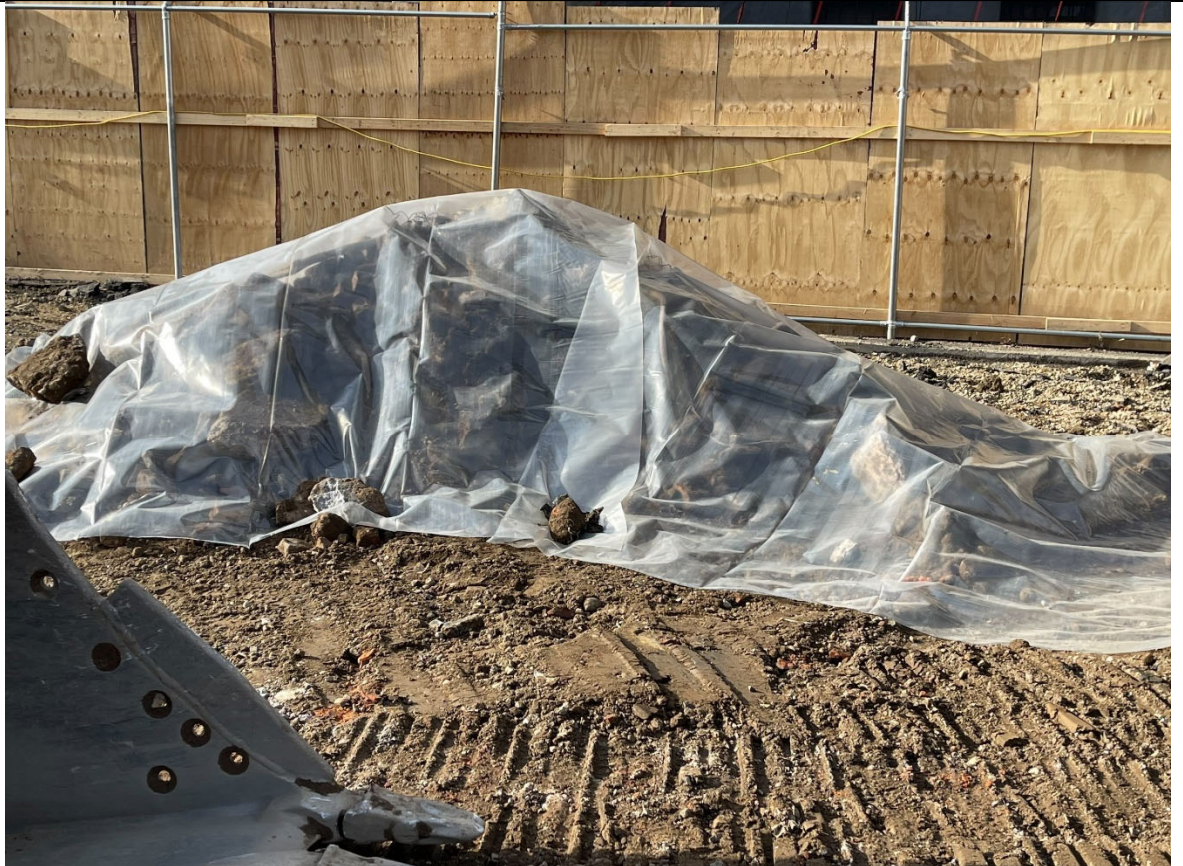
Photo 4 – Soil stockpiles covered with poly-sheeting.
