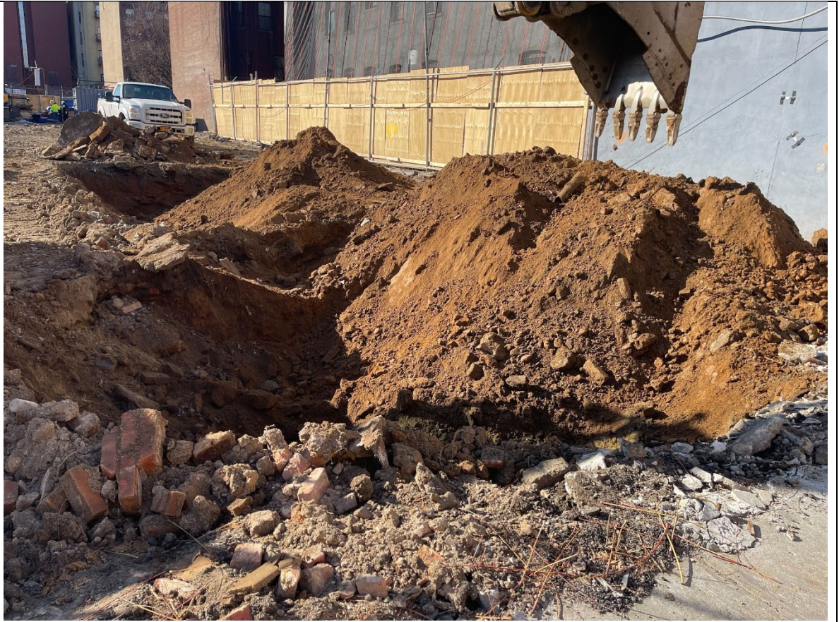
Photo 3 - View of excavation in Zone 7 to remove C & D material.
