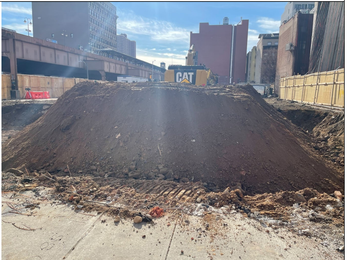
Photo 2 - View of Zone 7 excavation, stockpiling and C & D debris removed.
