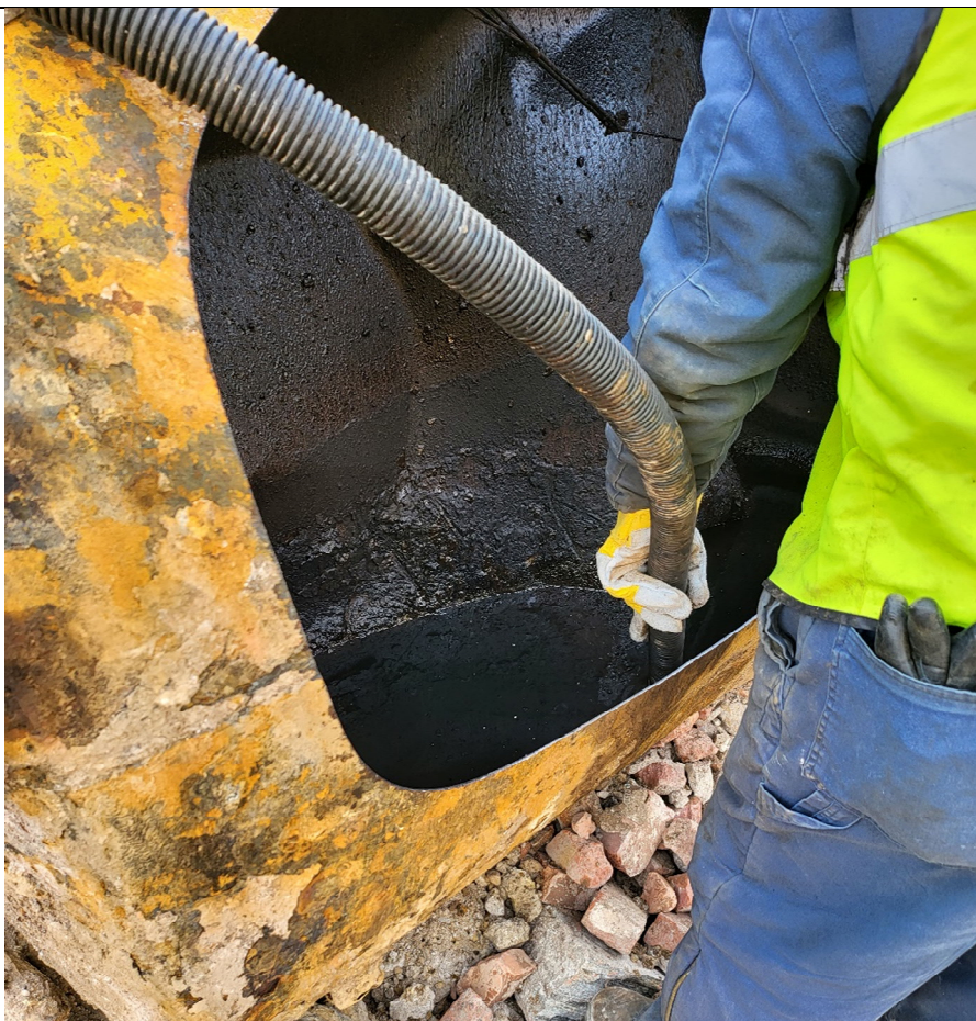
Photo 3 – View of tank content removal prior to cleaning.
