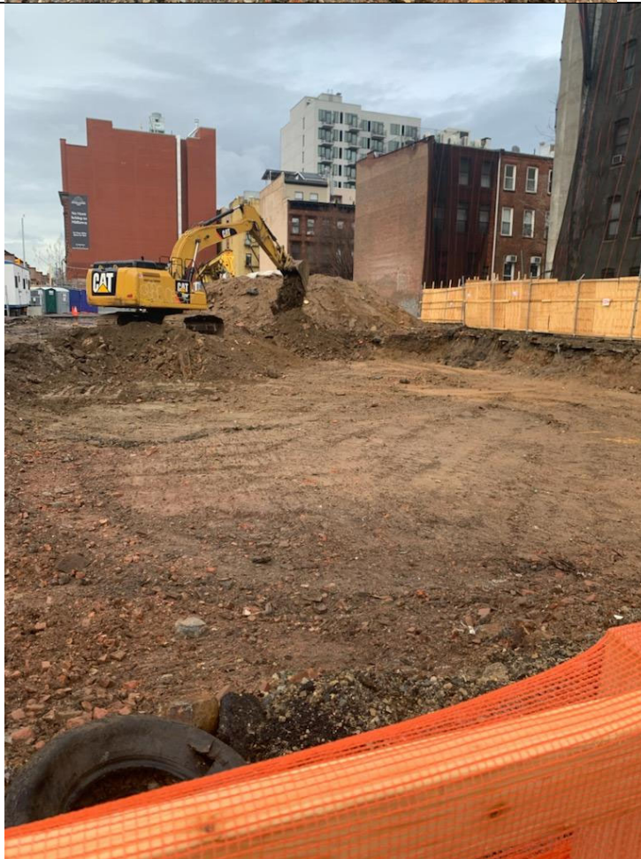
Photo 2 - View of Zone 4 0-4' excavation and stockpiling in preparation of trucking.
