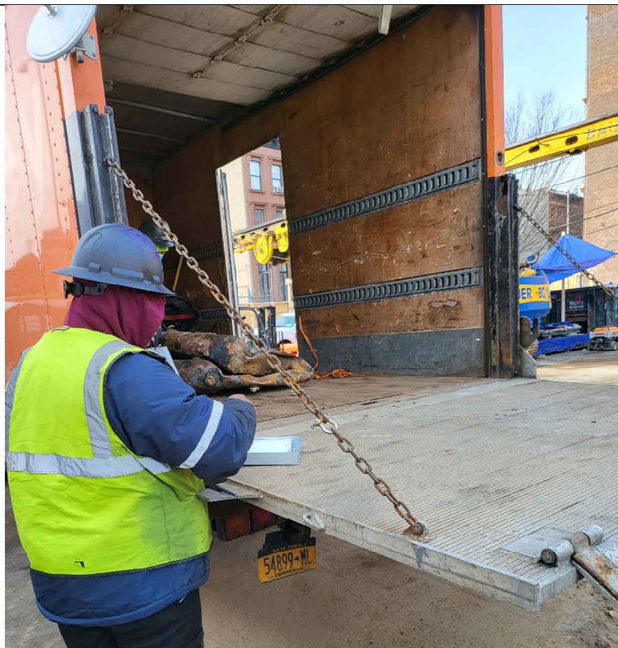
Photo 5 – View of tank loaded onto truck for disposal.
