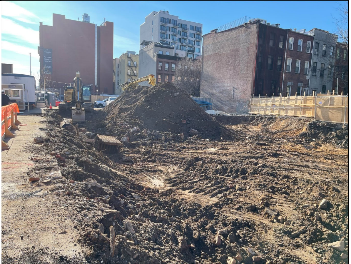
View of Zone 1/Zone 4 0-4' excavation and stockpiling in preparation for trucking.
