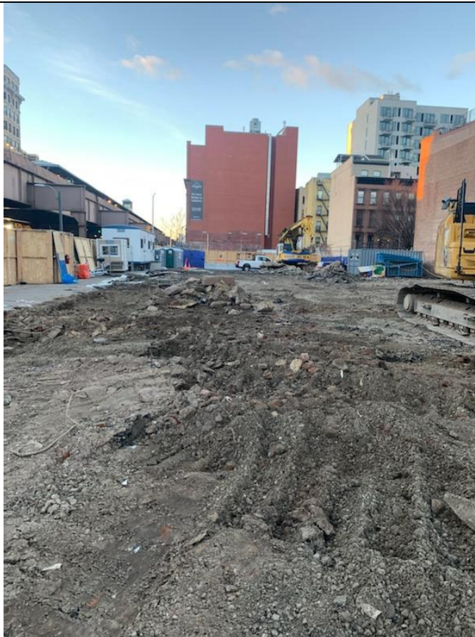
Photo 2 - View of SB-5 Hotspot location and excavation in Zone 7.
