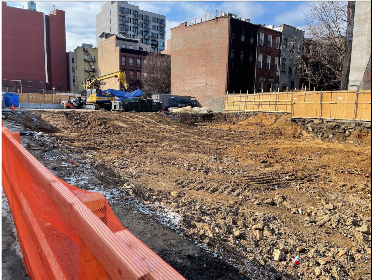
Photo 4 – View Site at EOD.
