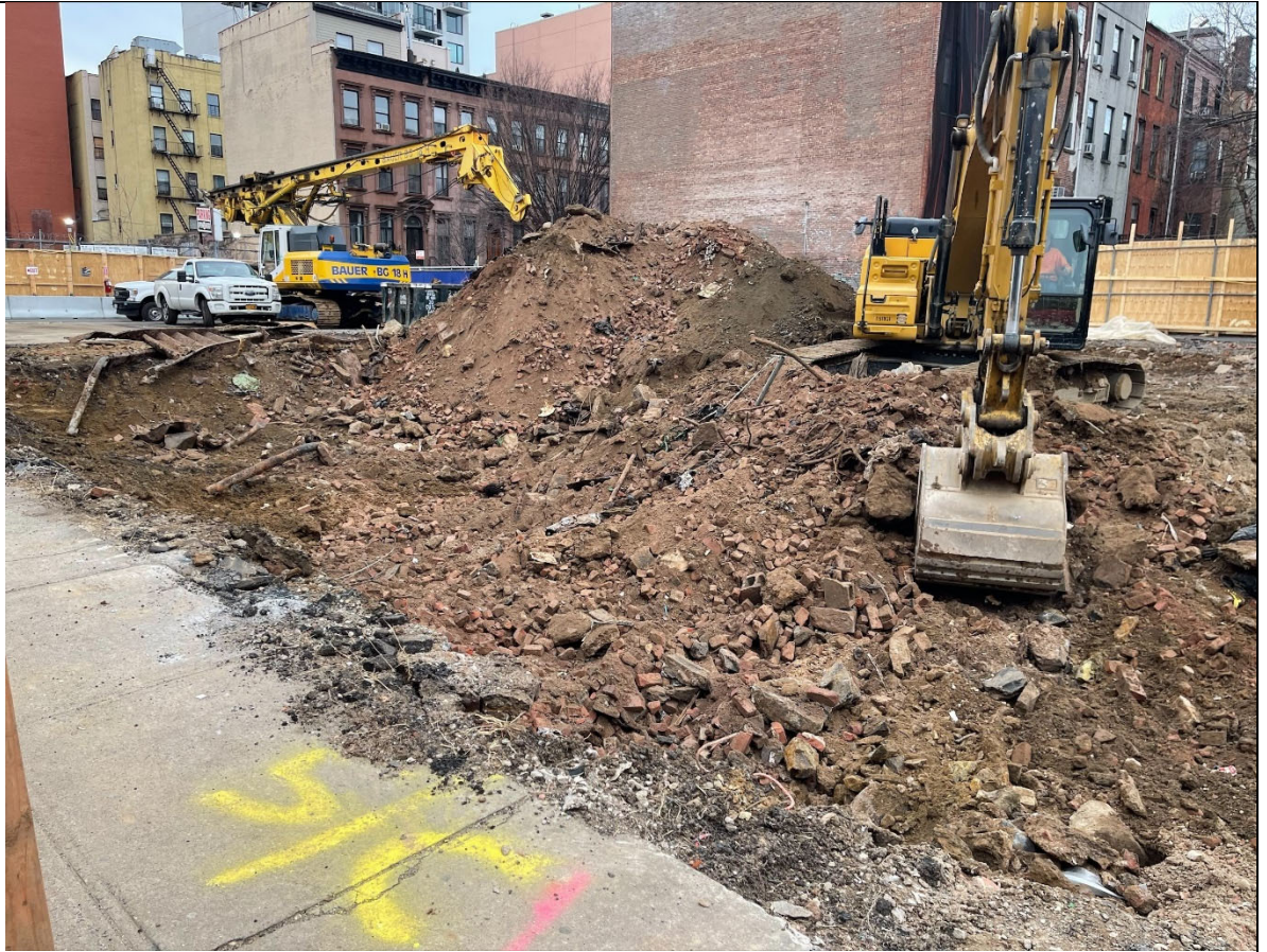
Photo 1 – View of Zone 1 0-4' excavation and stockpiling in preparation for trucking.
