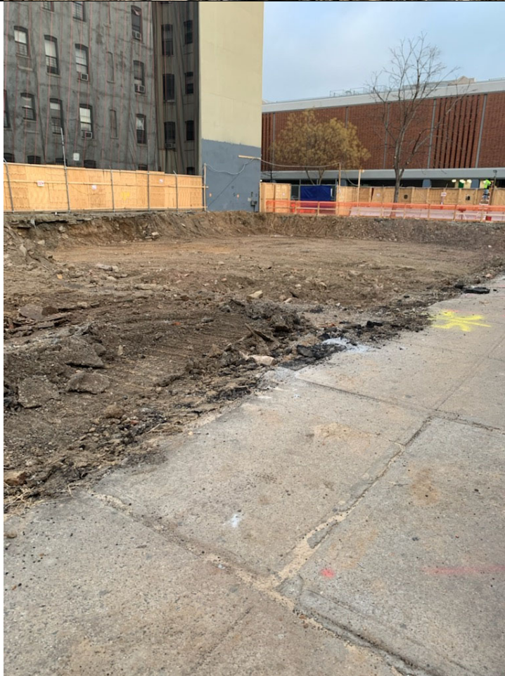
Photo 2 - View of Zone 4/7 0-4' excavation extent.
