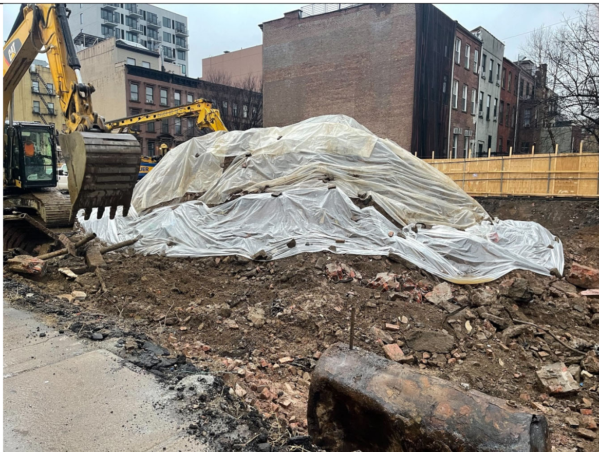
Photo 1 – View of Zone 1 0-4' stockpile covered with polysheeting.
