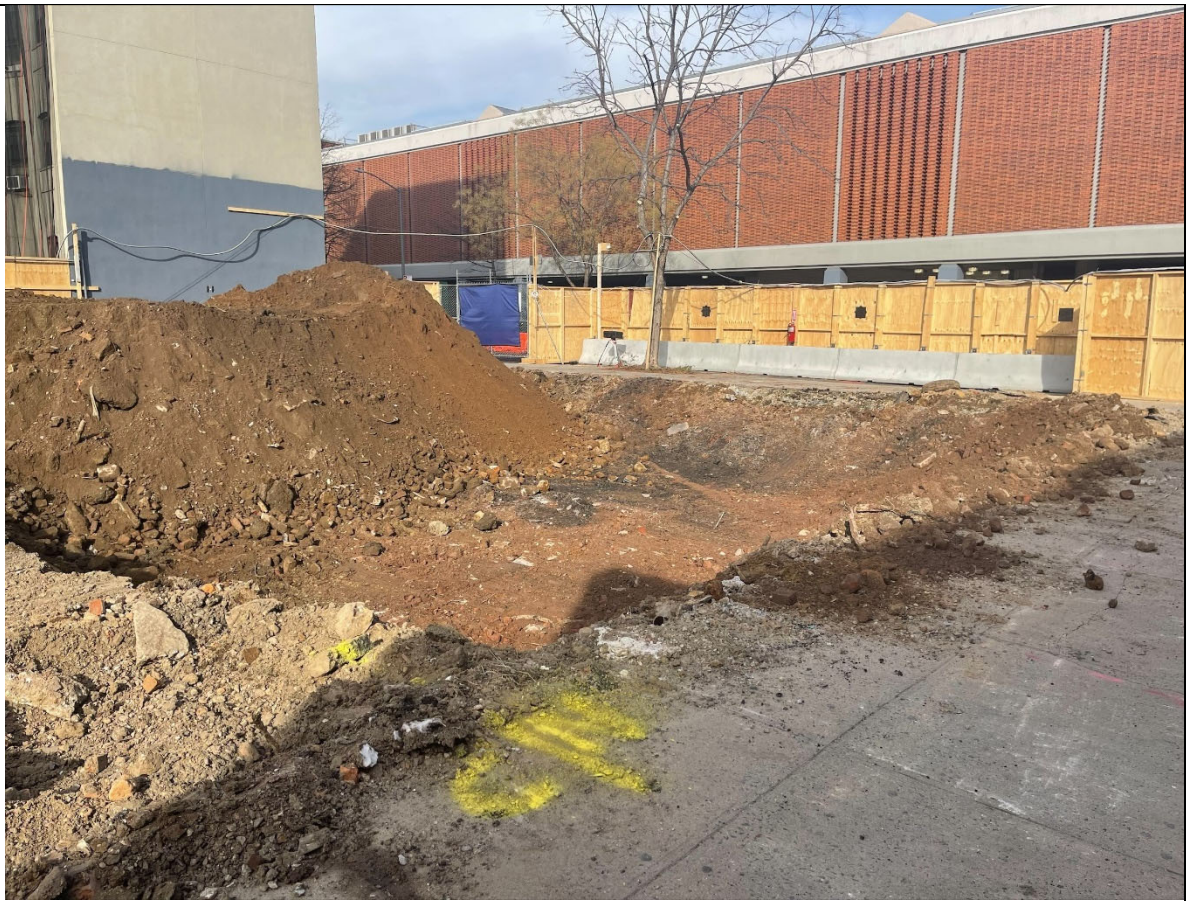
Photo 1 – View of Zone 7 excavation, stockpiling and C & D debris removed.
