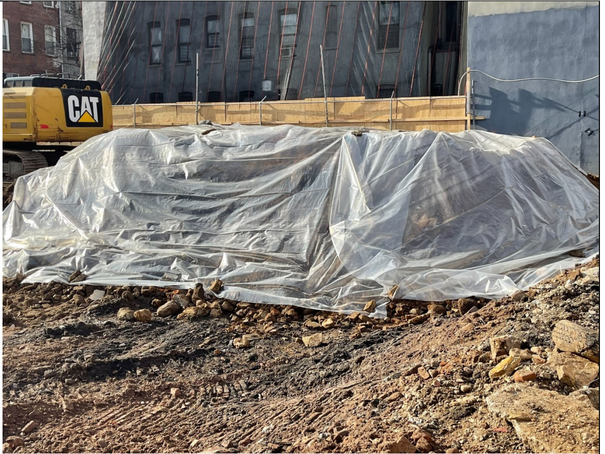
Photo 3 - Soil stockpiles covered with poly-sheeting.
