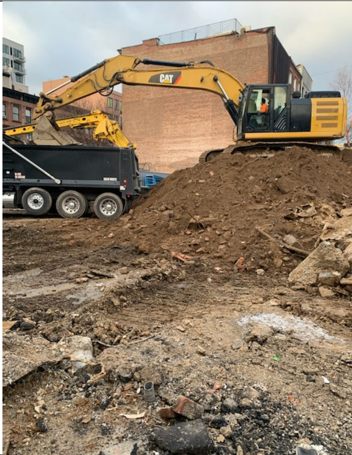
Photo 1 – View of Zone 4 0-4' excavation and truckloading for transport to Clean Earth of Carteret.
