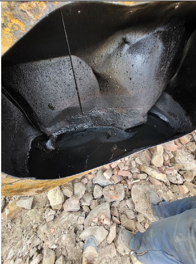
Photo 2 – View of tank contents.
