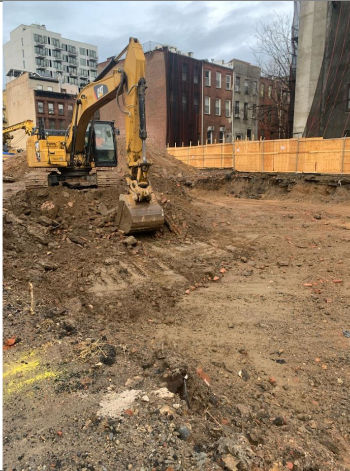
Photo 1 – View of Zone 4 0-4' excavation and stockpiling in preparation of trucking.
