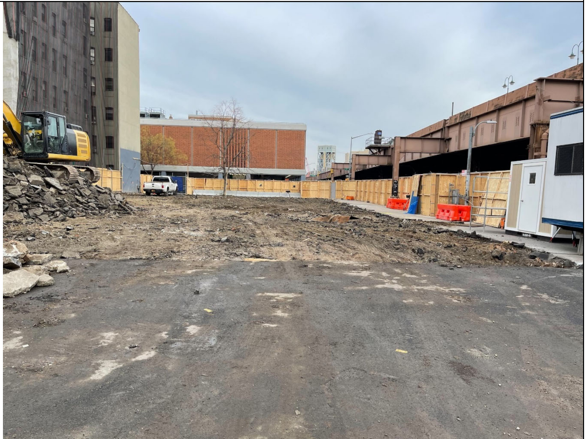
Photo 4 - View of asphalt scraping activities.
