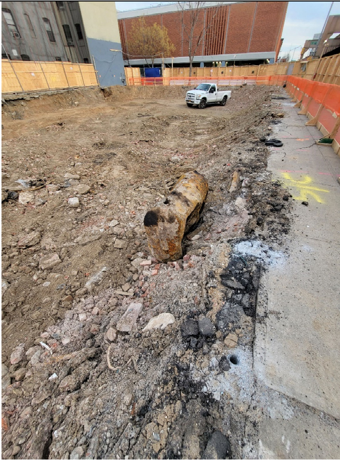
Photo 1 – View of Site at start of day and tank waiting to get cleaned and removed.
