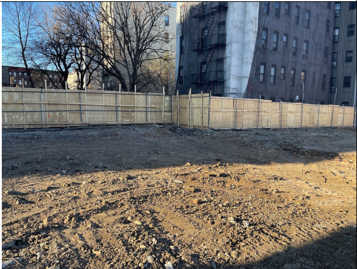
Photo 2 - View of SB-1 Hotspot location backfilled with surrounding soil to grade to safety reasons.
