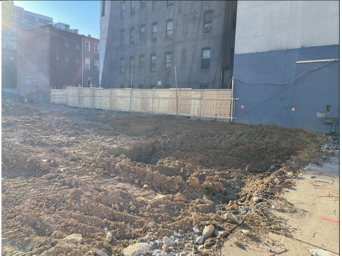
Photo 4 - View of Zone 7 grading after C & D Removal.
