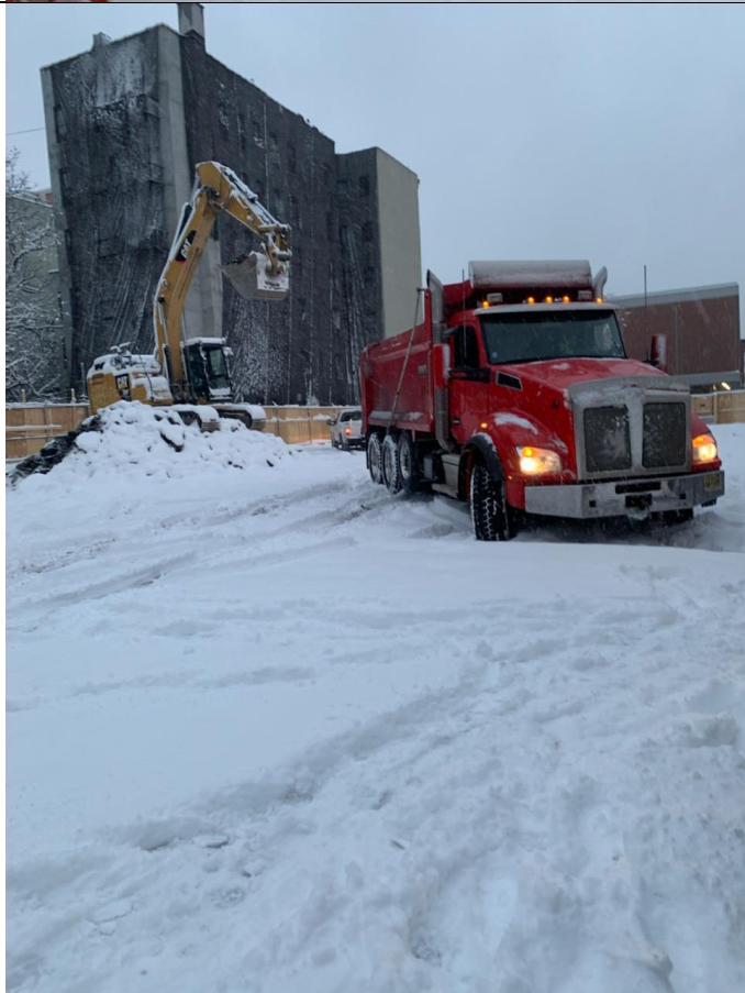
Photo 2 - View of asphalt scraping activities.
