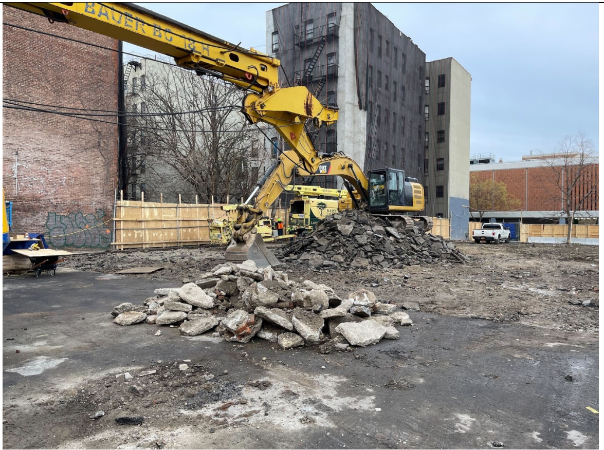
Photo 1 – View of asphalt scraping activities.
