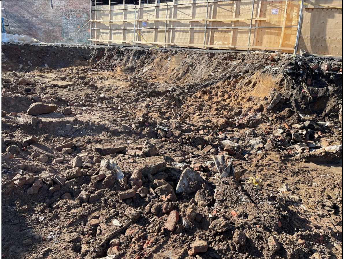
View of Zone 1 0-4' excavation extent and location of discovered tank.
