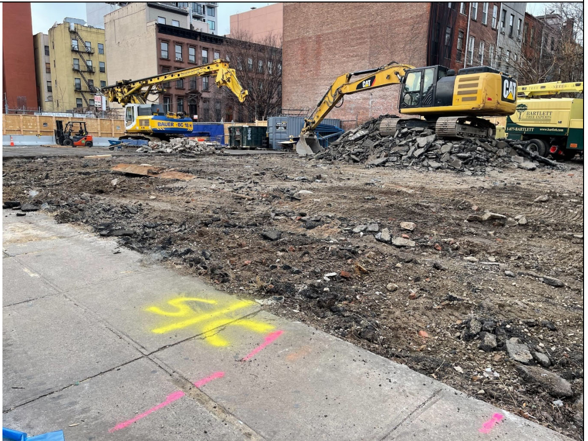
Photo 2 - View of asphalt scraping activities.
