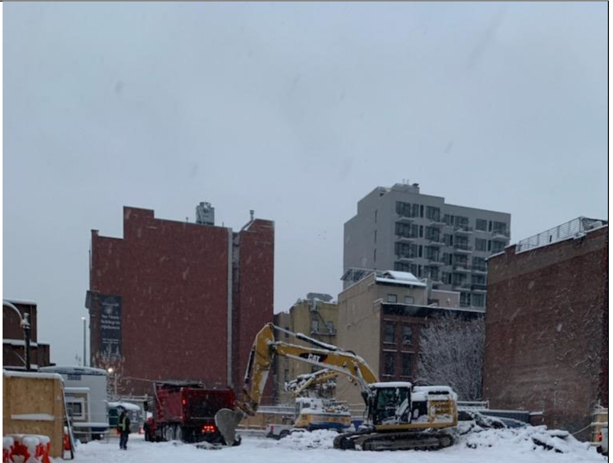
Photo 1 – View of asphalt scraping activities.
