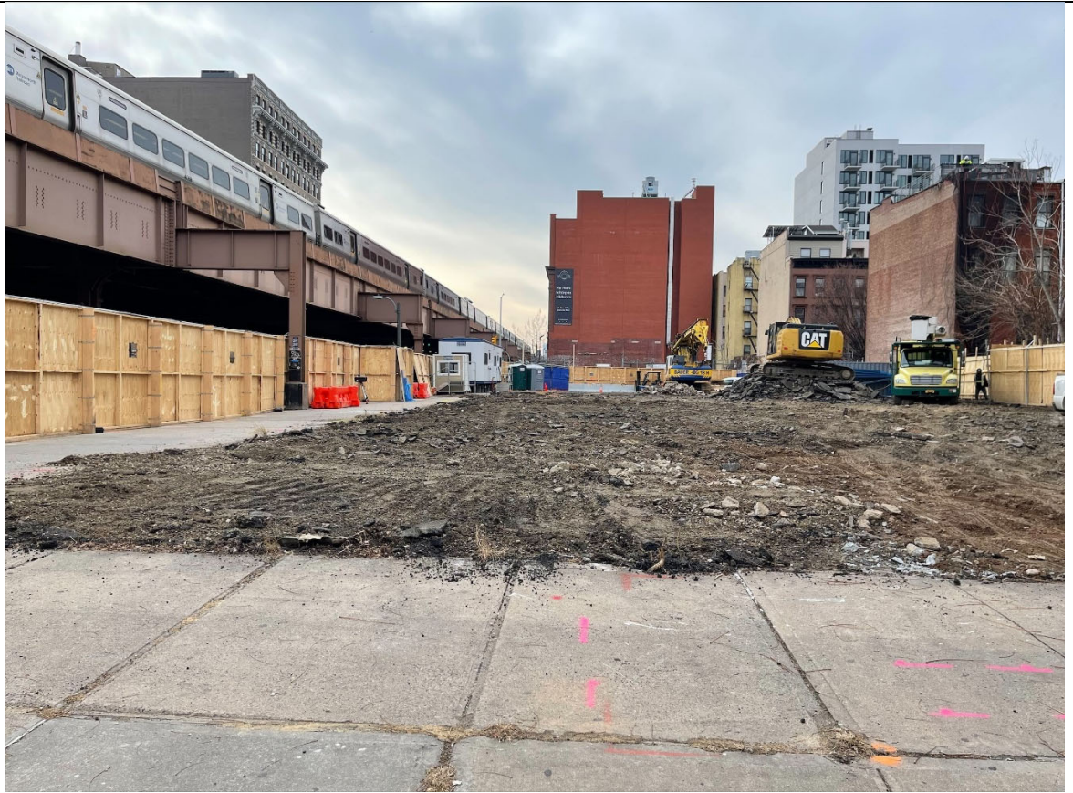
Photo 3 - View of asphalt scraping activities.
