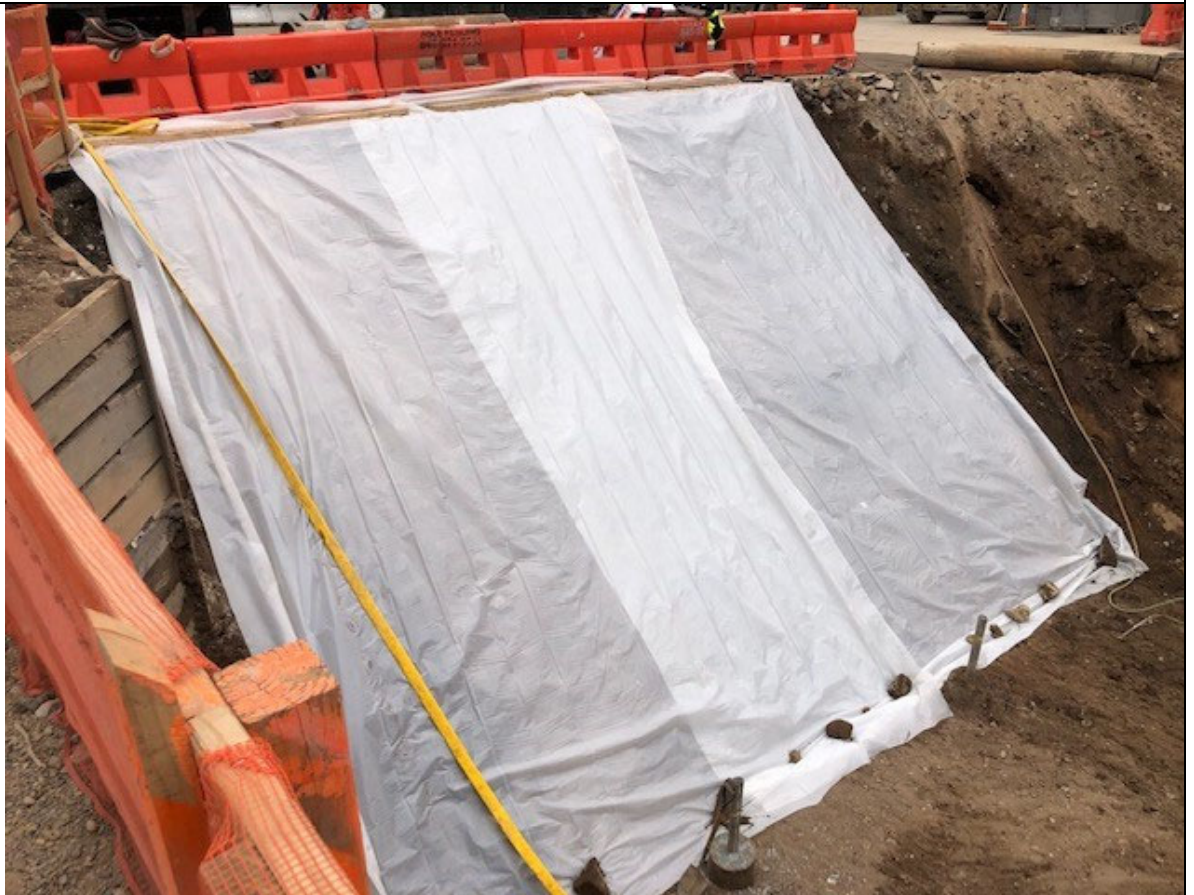
Photo 2 – View of covered ramp area
