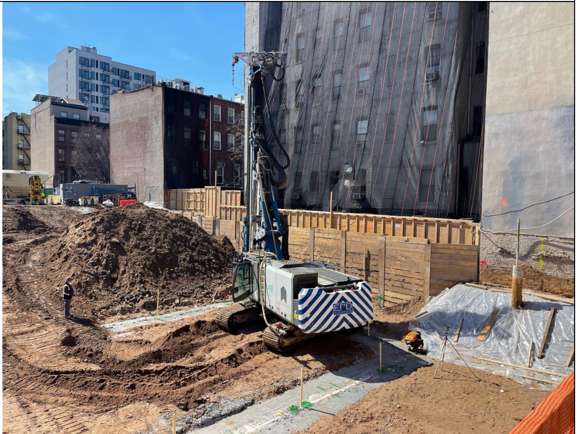
Photo 2 – View of drilling activities.
