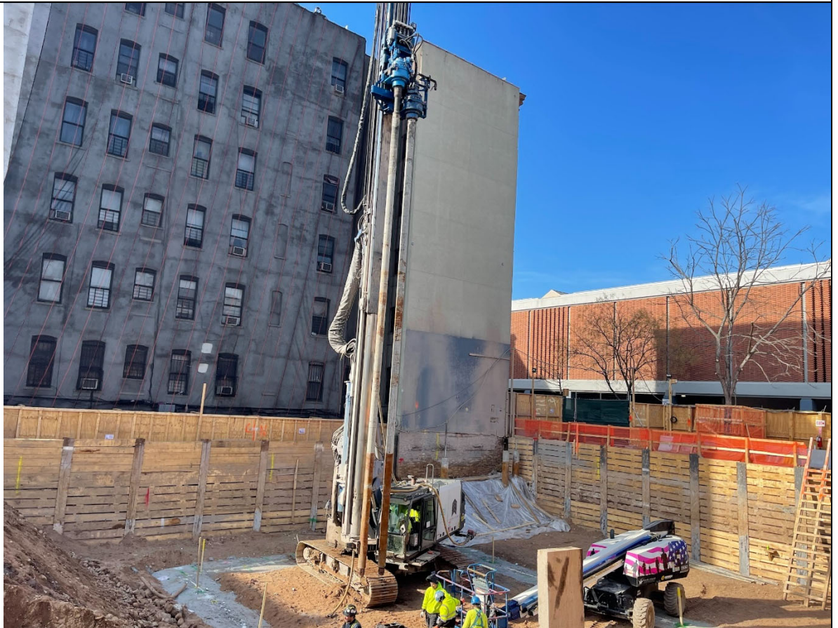
Photo 4 – View of drilling activities.
