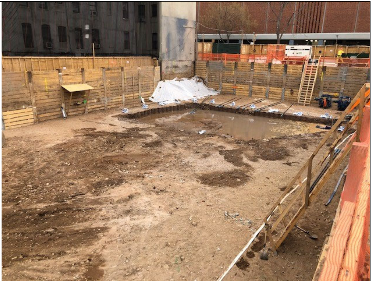
Photo 3 – View of the covered berm area and elevator pit.
