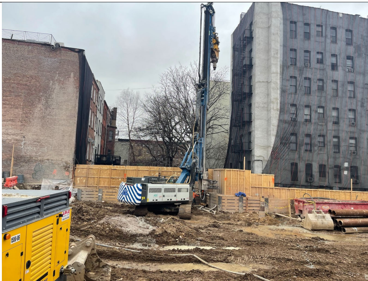
Photo 1 – View of caisson pile installation.
