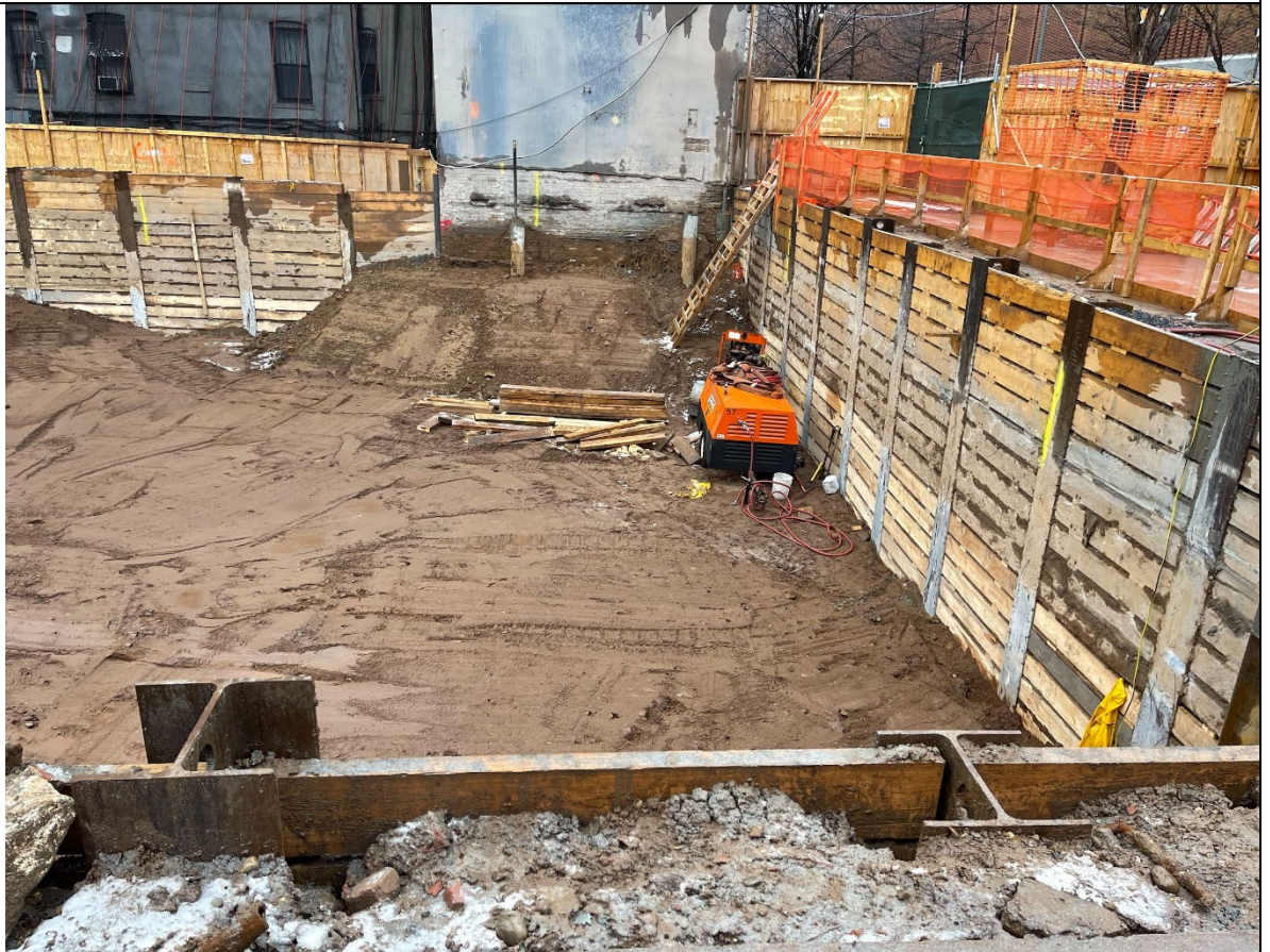
Photo 4 – View of bermed area.
