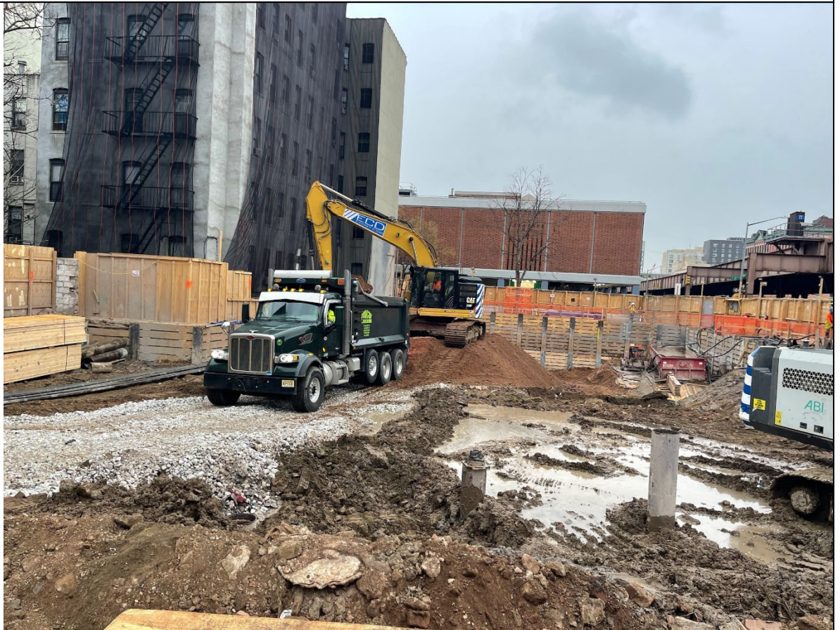
Photo 2 – View of truck loading activities to IRRC.
