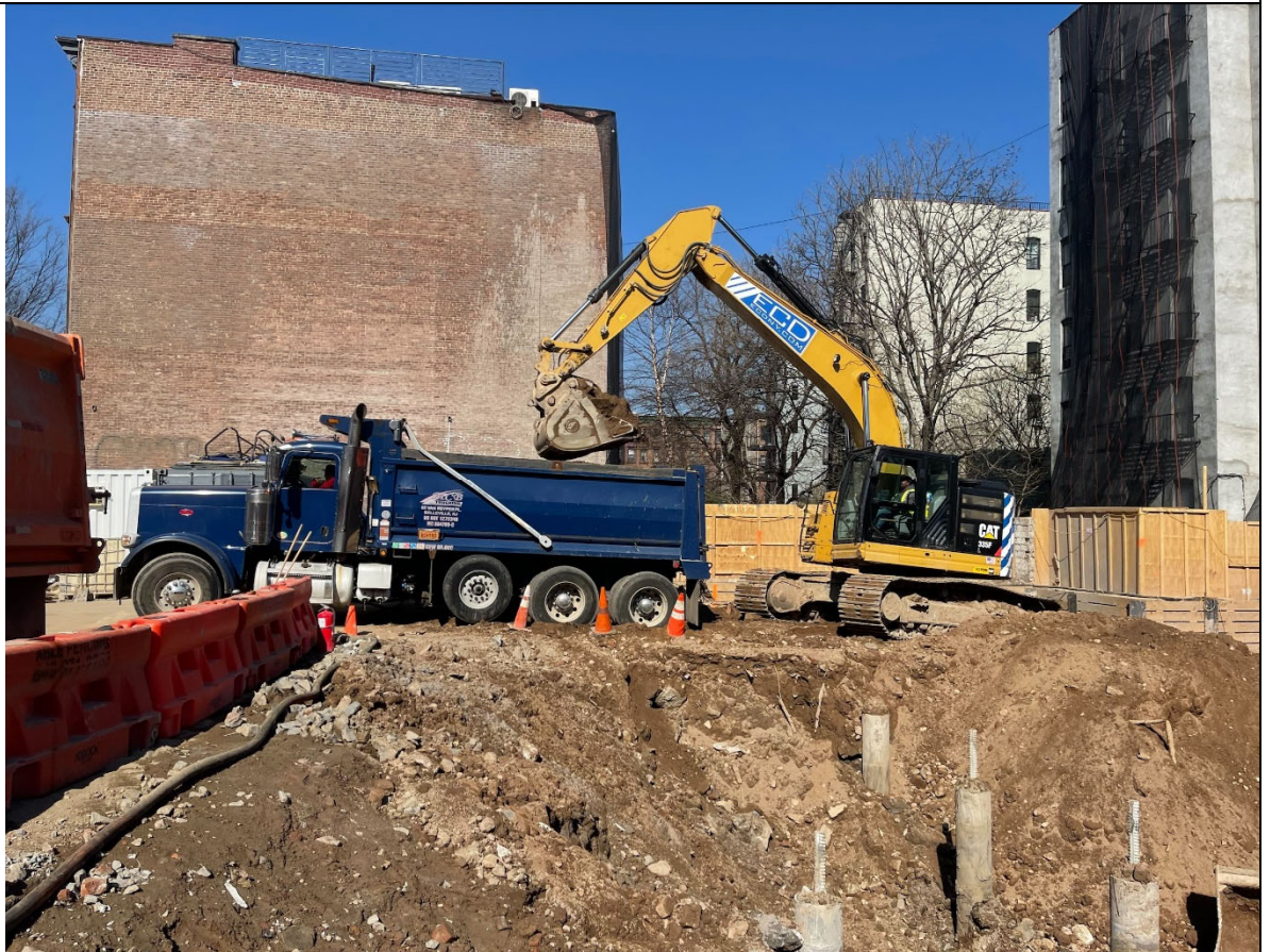
Photo 4 – View of trucking loading for transport to Clean Earth of Carteret.
