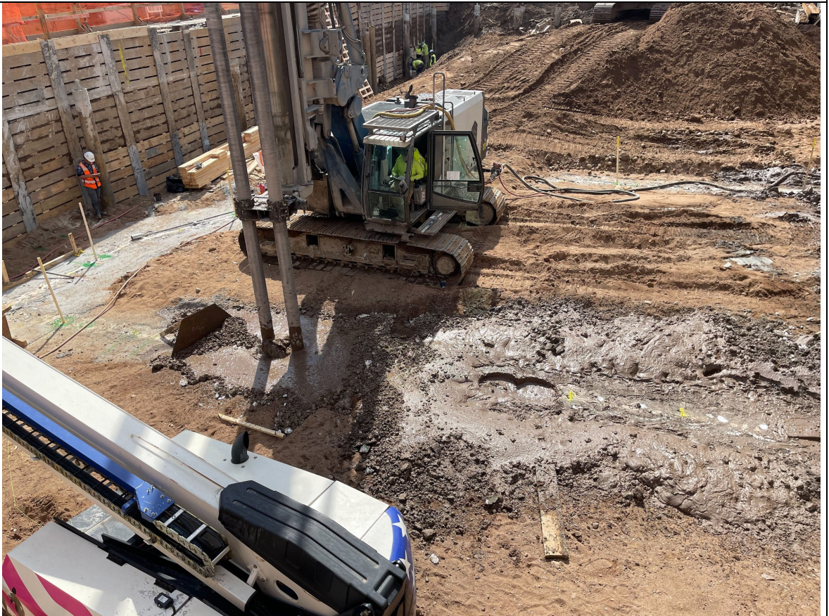
Photo 4 – View of drilling activities.
