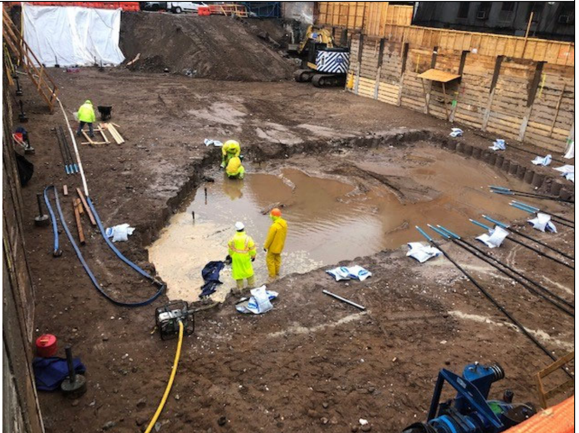
Photo 4 – View of dewatering activities.
