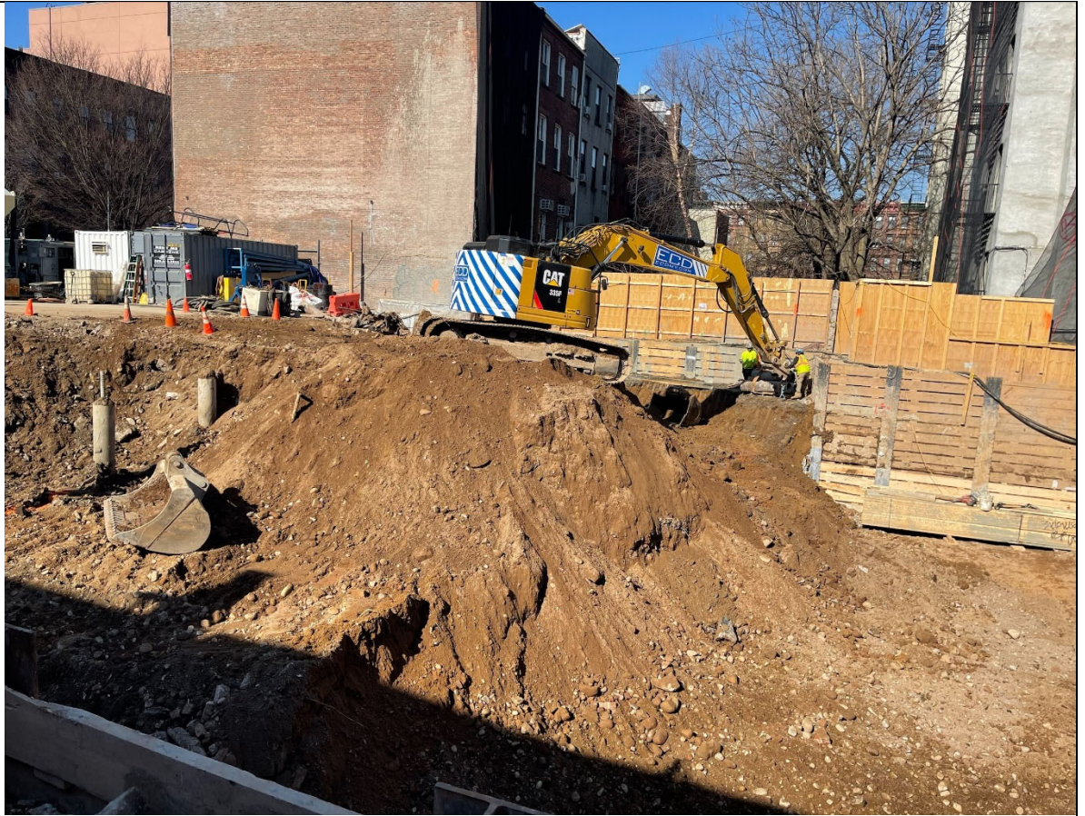
Photo 3 – View of the excavation of the 0-5' soil from the truck ramp.
