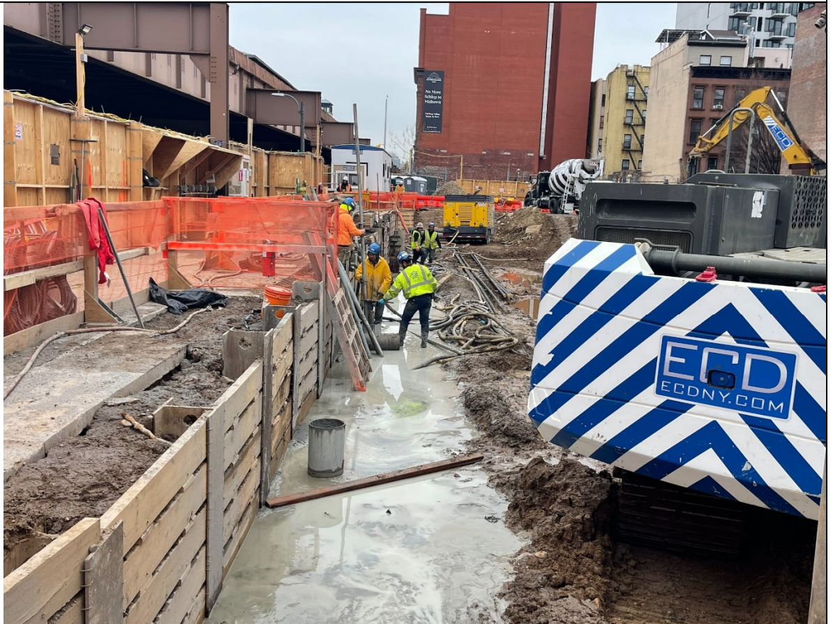
Photo 4 – View of caisson piles.
