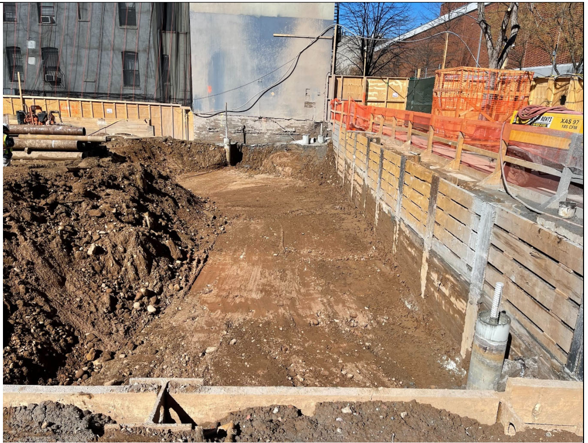
Photo 3 – View of excavated area.
