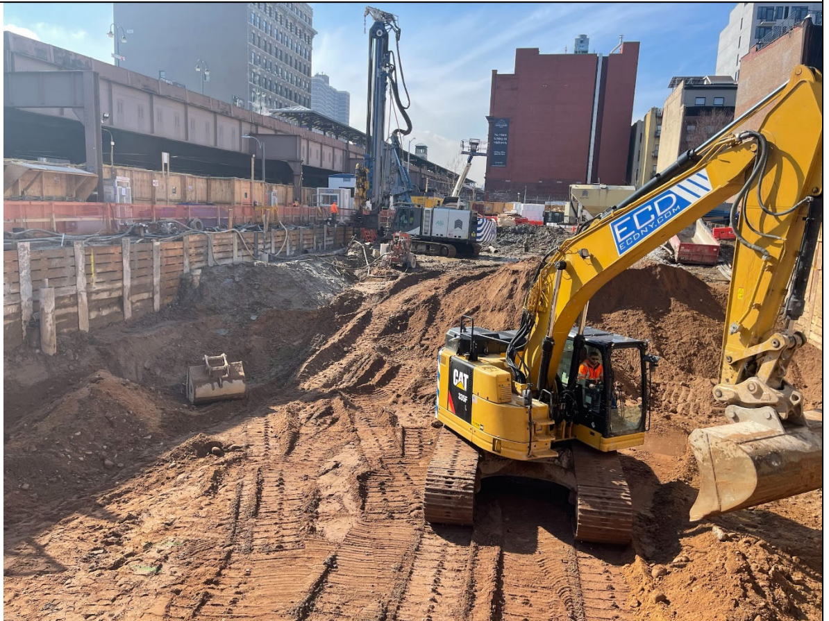
Photo 2 – View of Zone 5 excavation.
