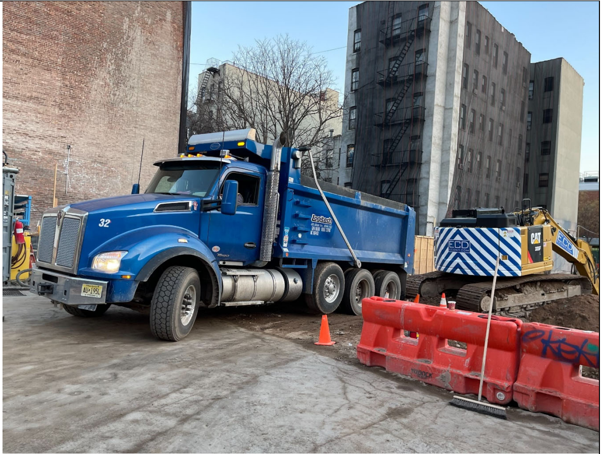
Photo 1 – View of truckloading activities for transport to PPark NJ LLC.
