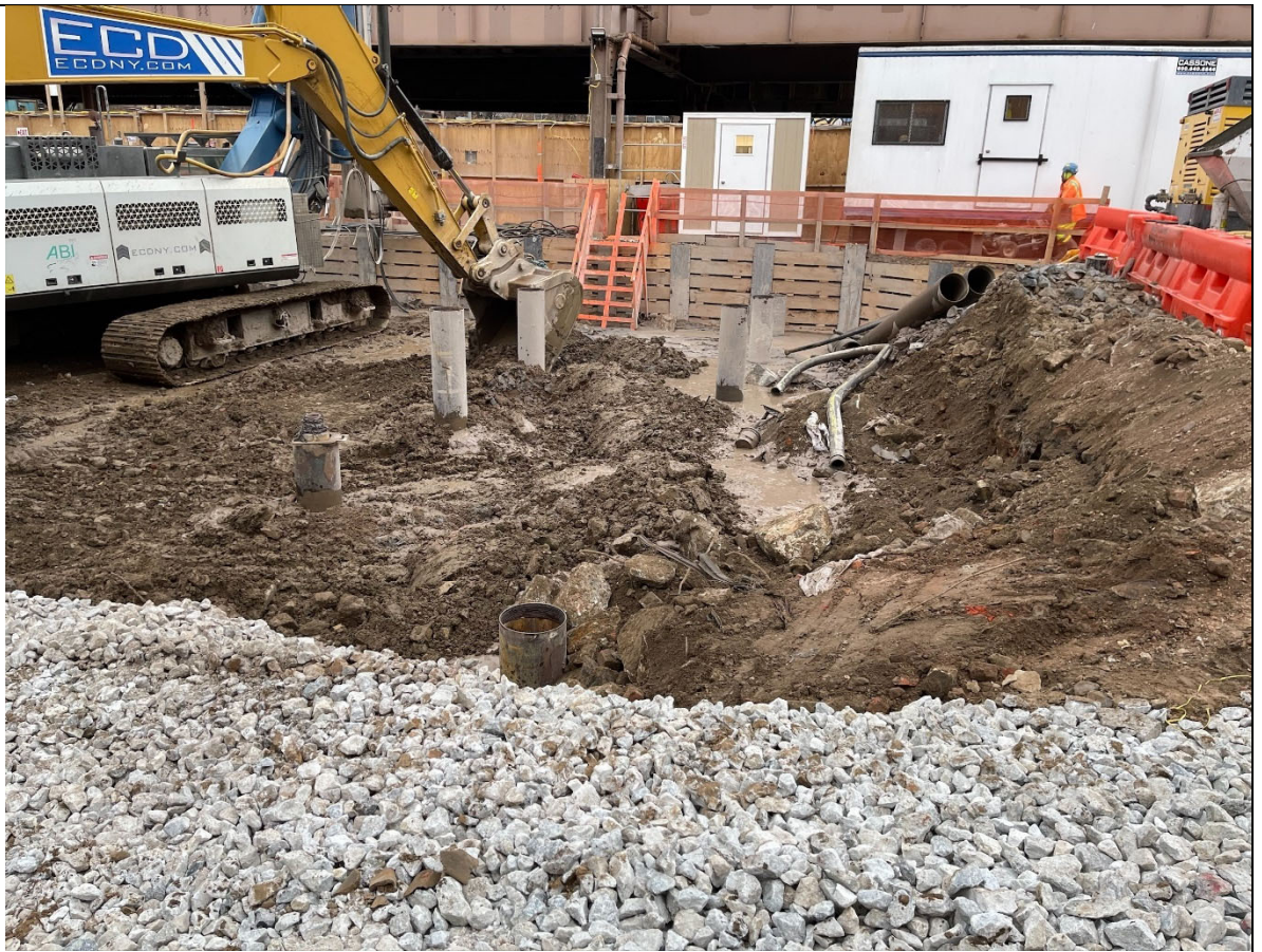
Photo 1 – View of excavation around caisson piles.
