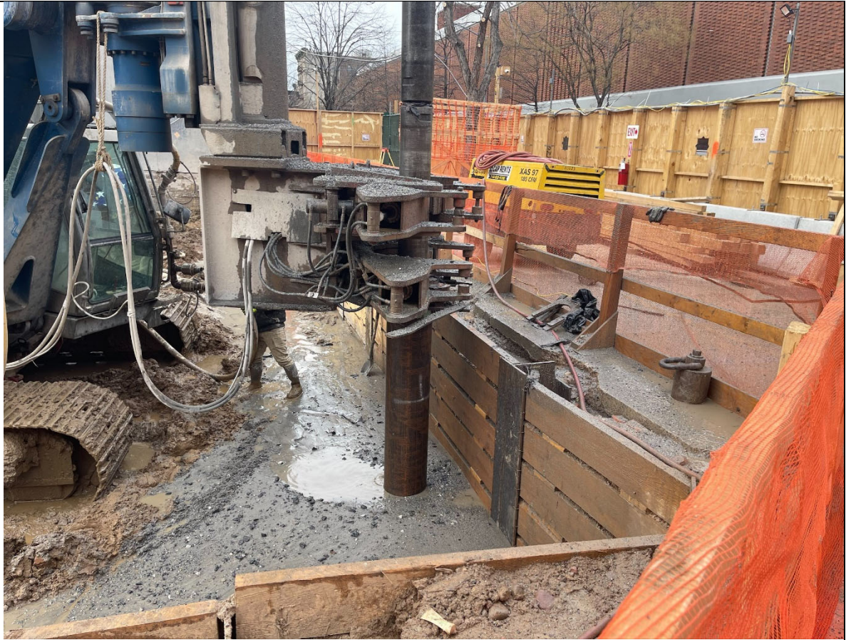
Photo 3 – View of caisson pile installation.
