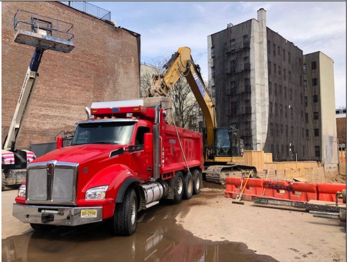
Photo 4 – View of trucking loading activities for transport to PPark NJ LLC.
