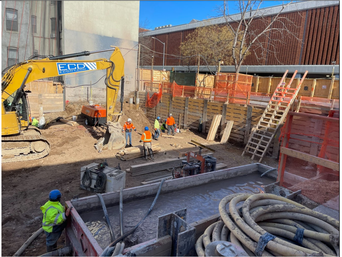
Photo 1 – View of excavation area.
