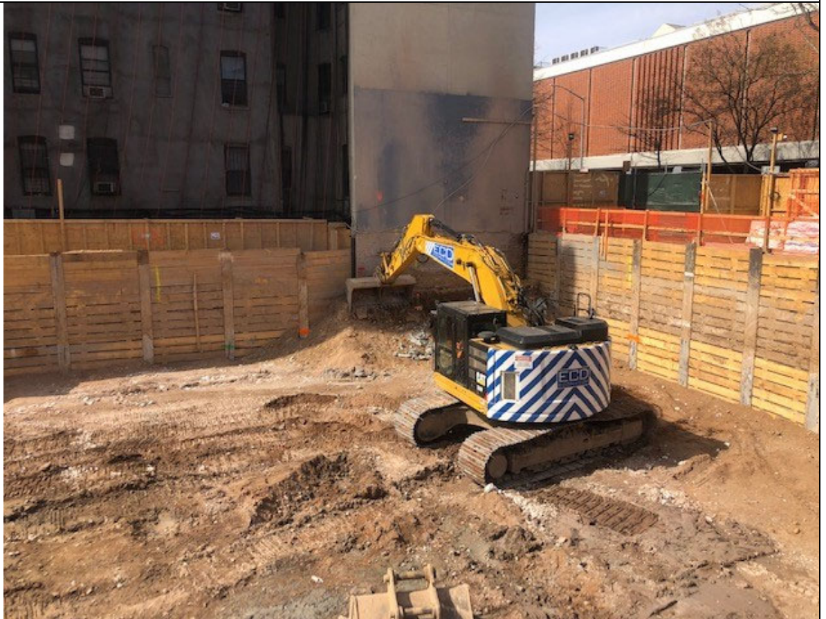
Photo 2 – View of berm reinforcement.
