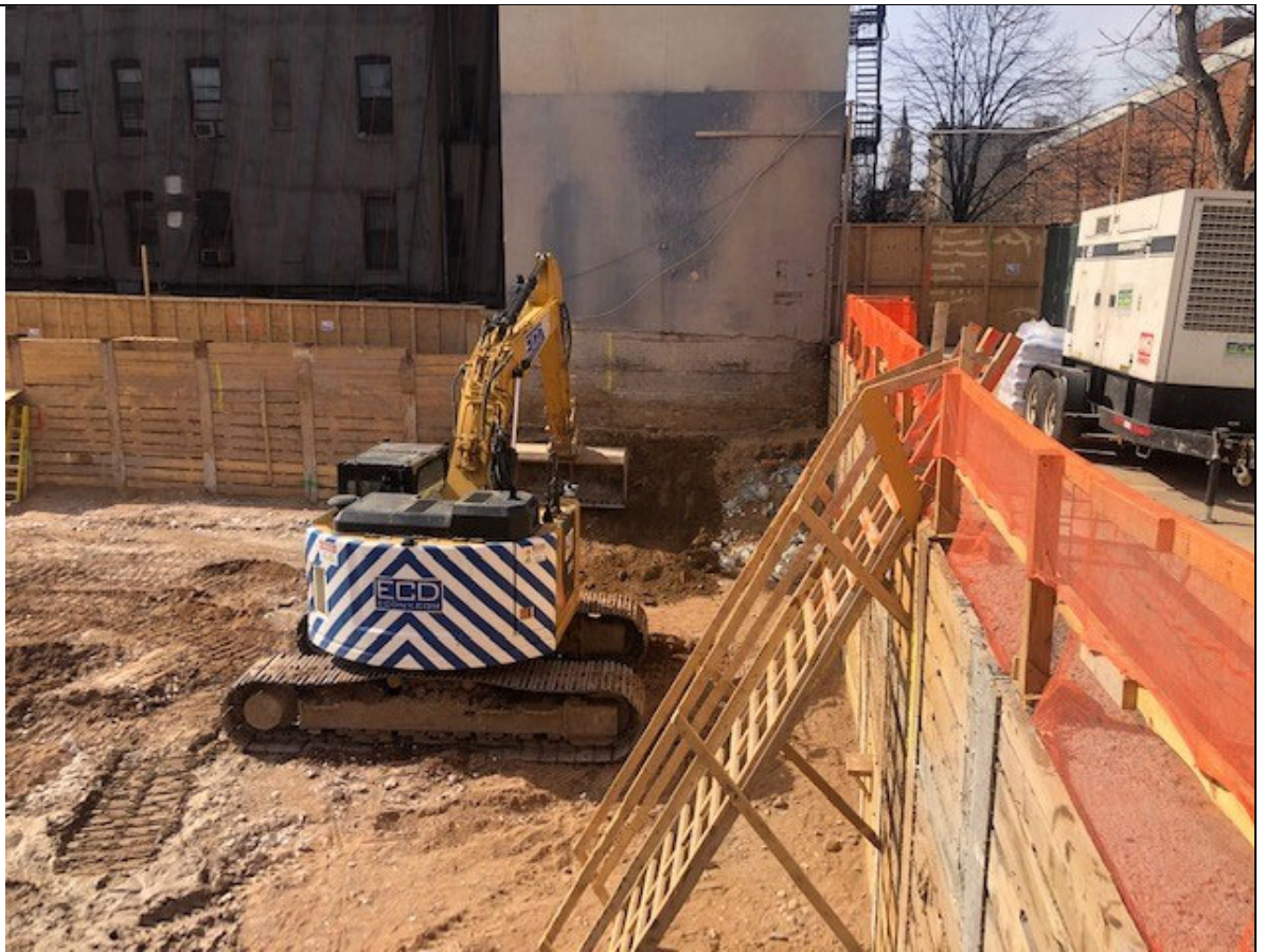
Photo 3 – View of berm reinforcement.
