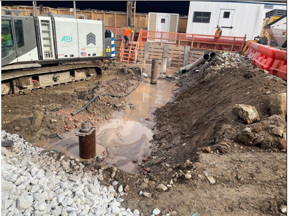
Photo 2 – View of caisson pile installation.
