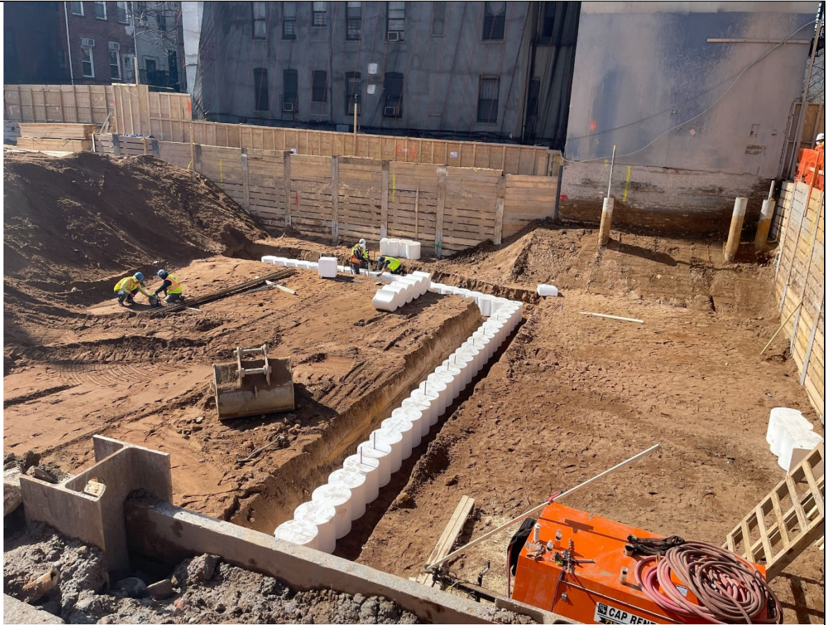
Photo 3 – View of dug out footing area.
