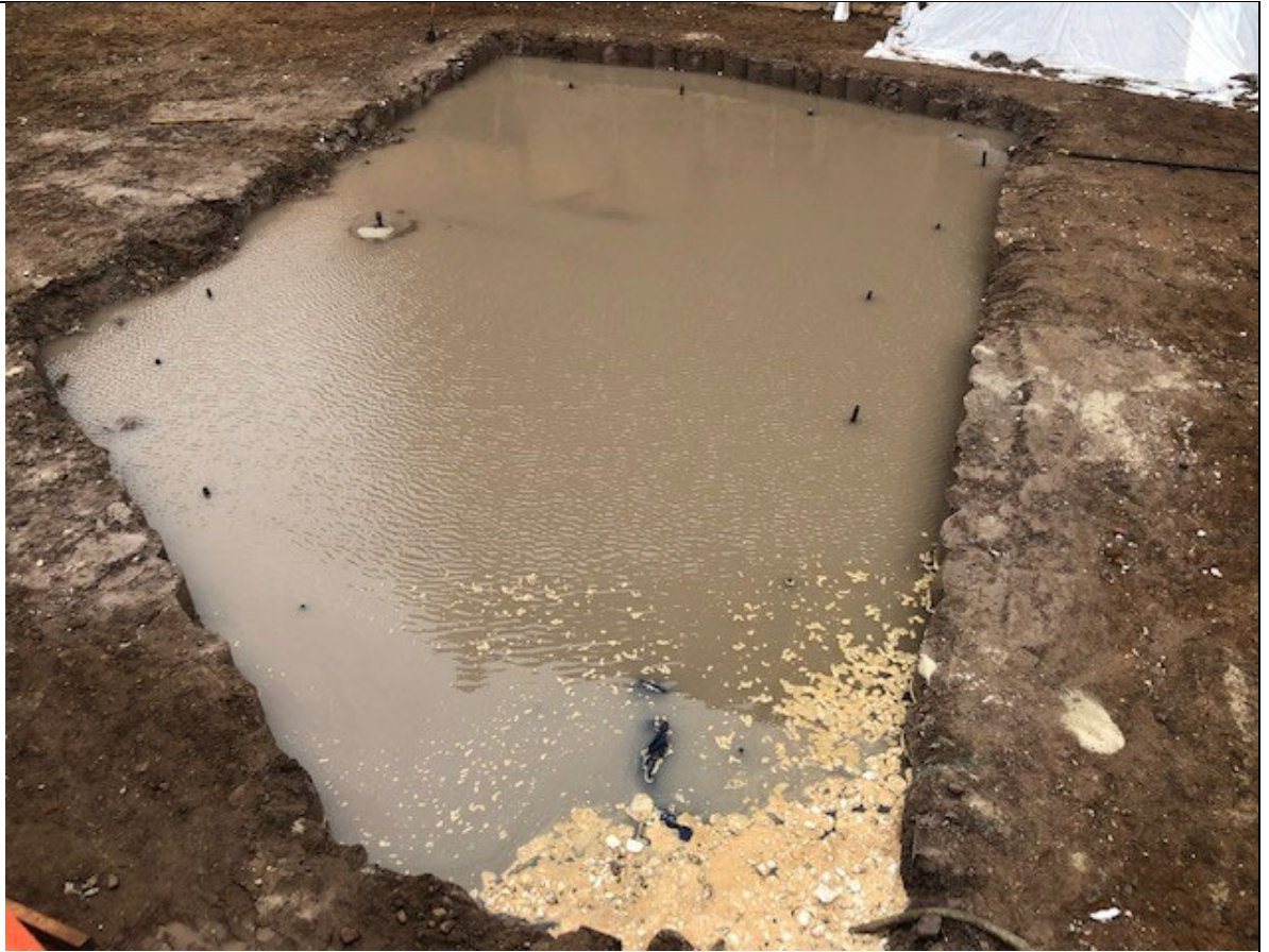
Photo 3 – View of elevator pit.
