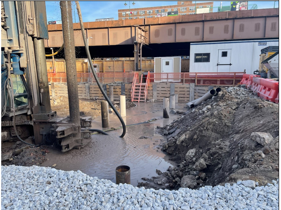
Photo 4 – View of caisson pile installation.
