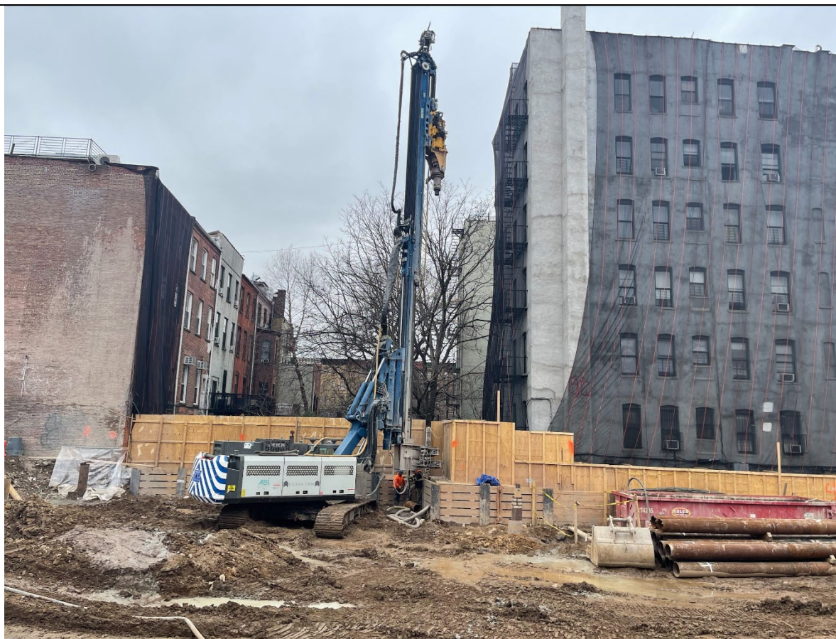
Photo 2 – View of caisson pile installation.
