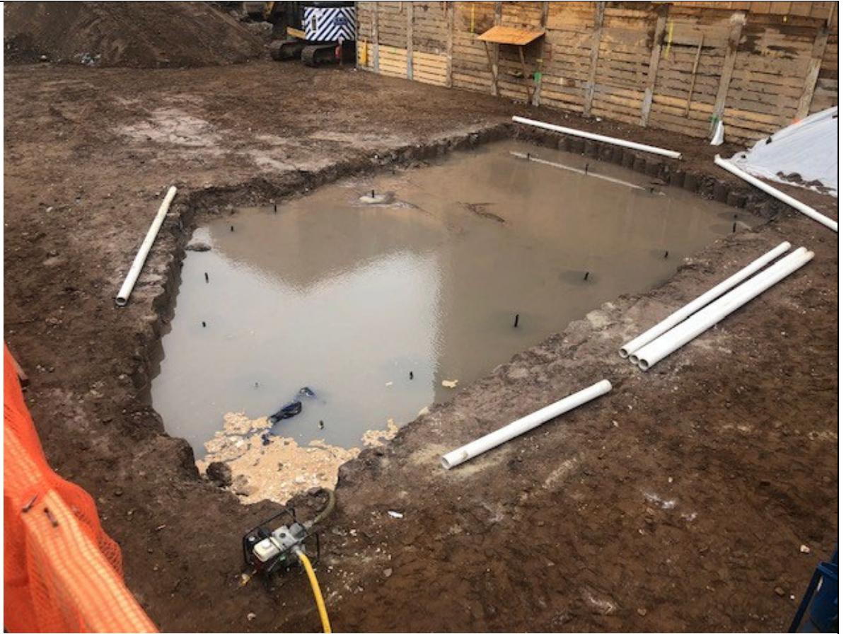
Photo 1 – View of dewatering activities.
