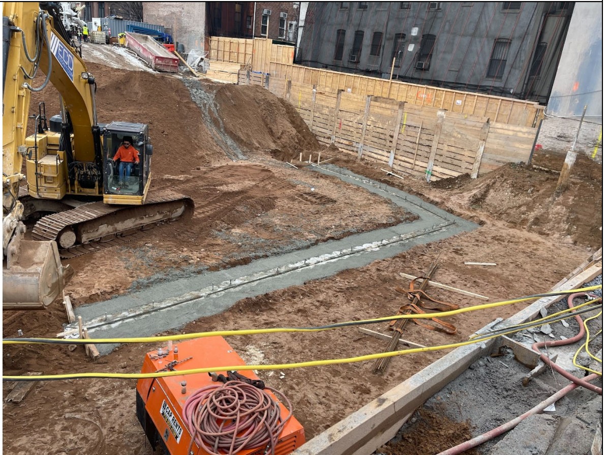
Photo 4 – View of concrete pour for footing area.
