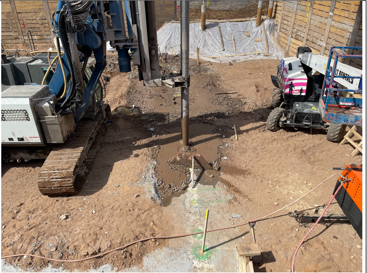
Photo 3 – View of drilling activities.
