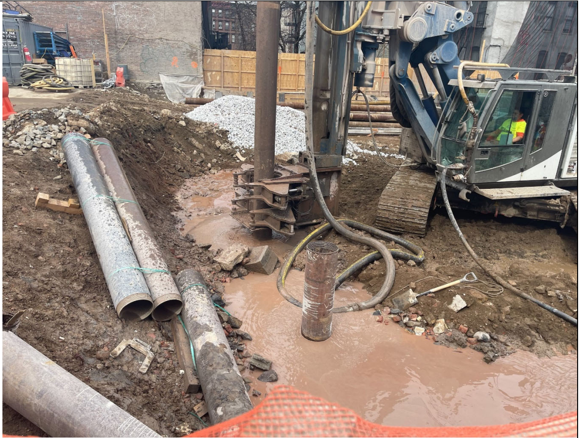
Photo 1 – View of caisson pile installation.
