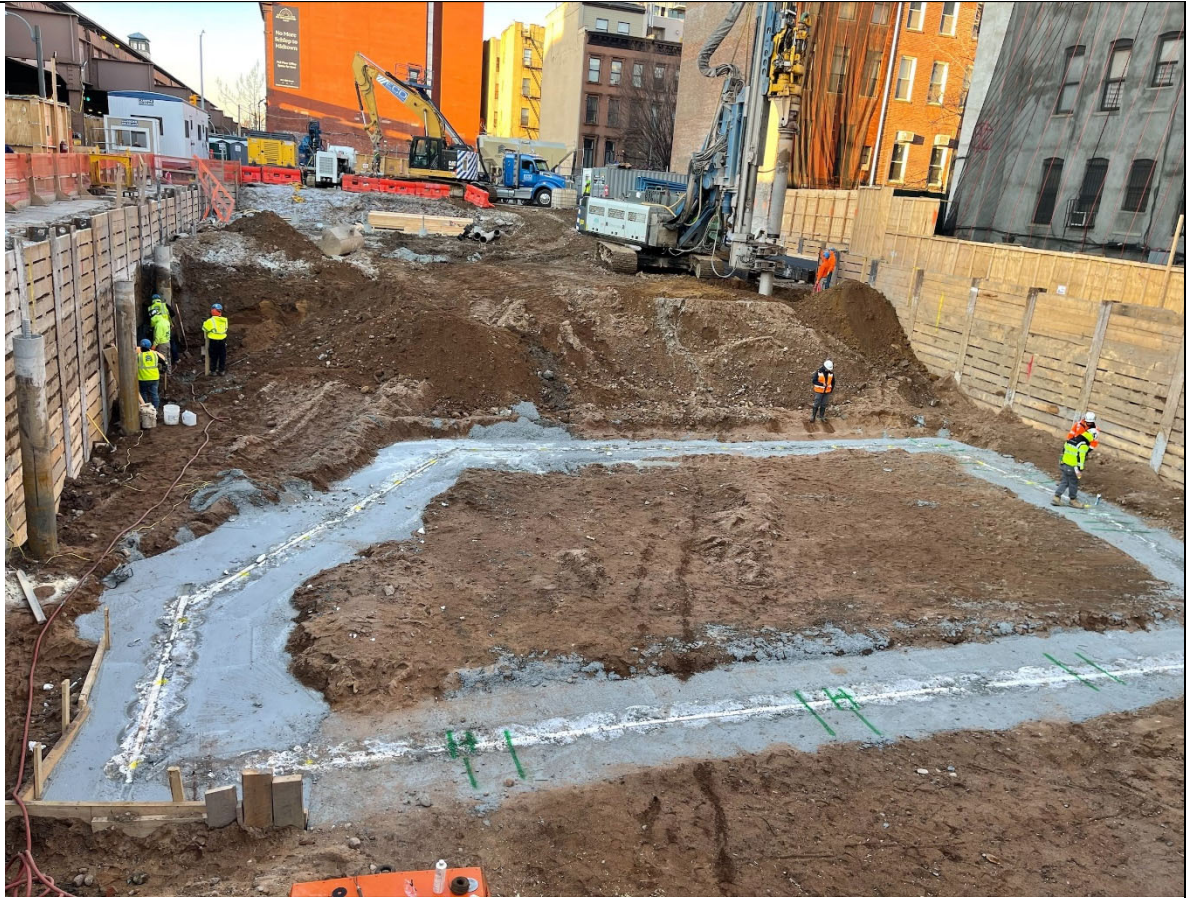
Photo 1 – View of Site conditions.
