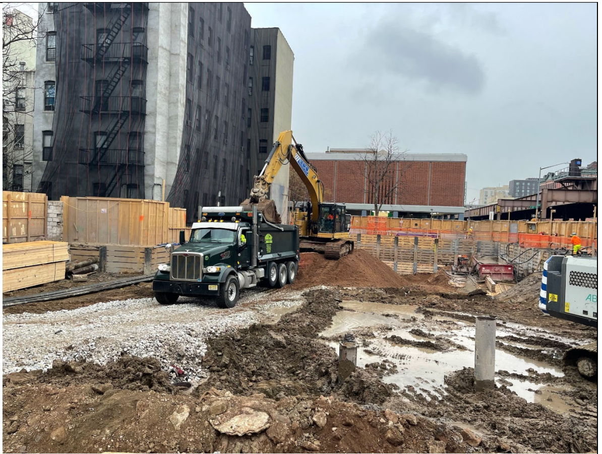
Photo 3 – View of truck loading activities to IRRC.
