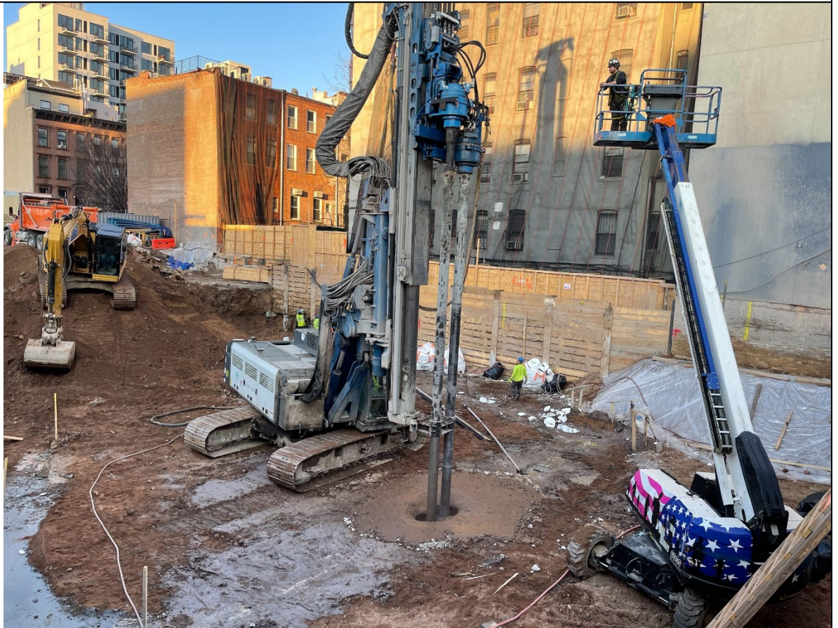
Photo 2 – View of Drilling activities.
