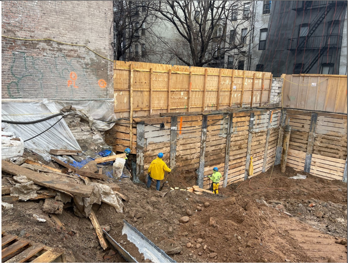
Photo 1 – View of shoring activities.
