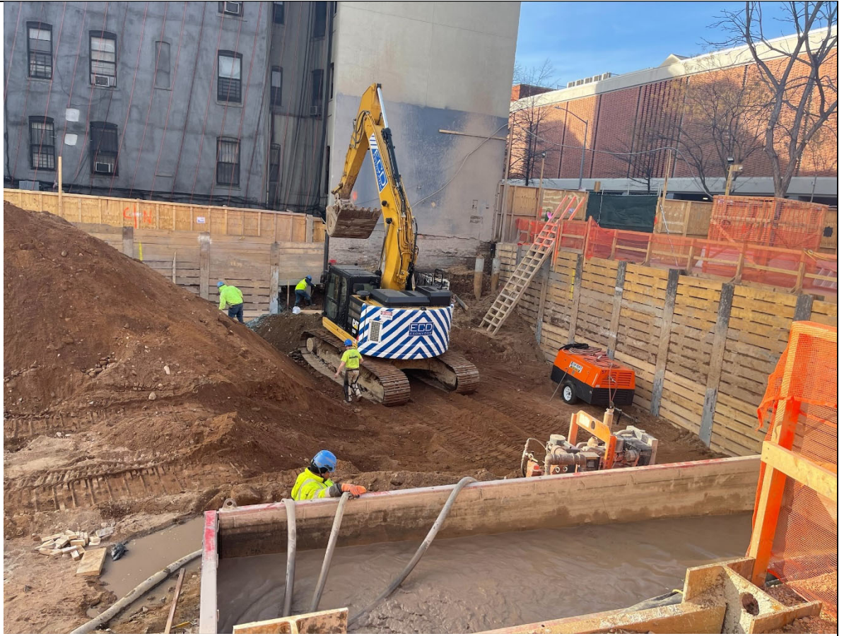
Photo 3 – View of excavated area.
