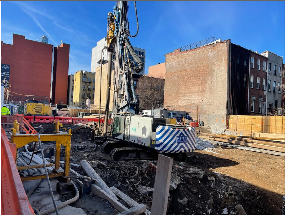
Photo 2 – View of caisson pile installation.
