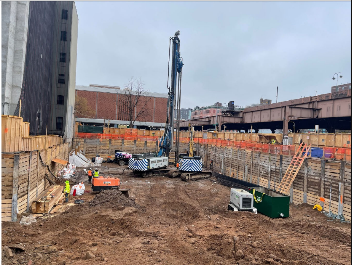
Photo 2 – View of drilling activities.
