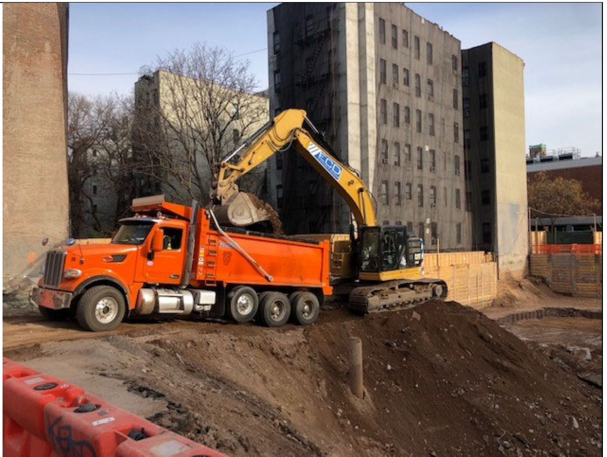
Photo 1 – View of trucking loading activities for transport to PPark NJ LLC.
