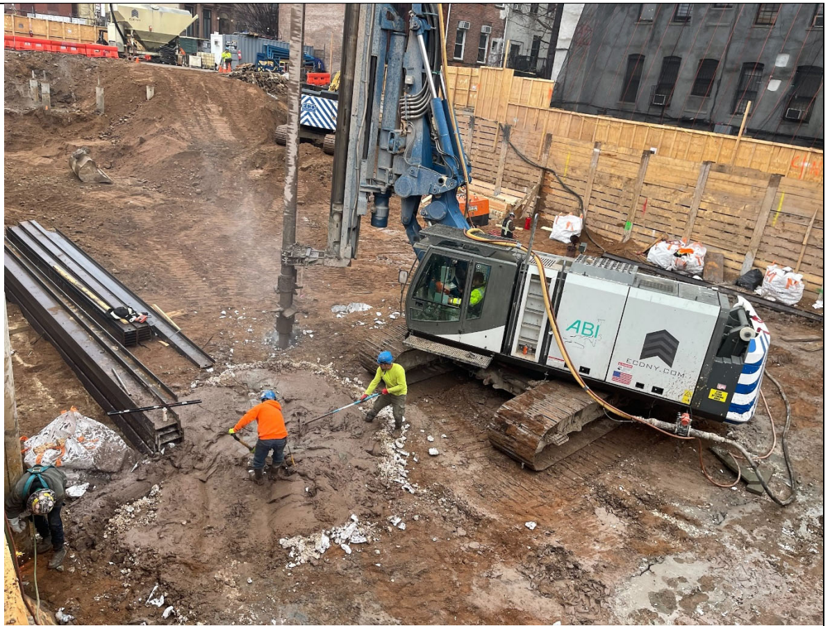
Photo 3 – View of drilling activities.
