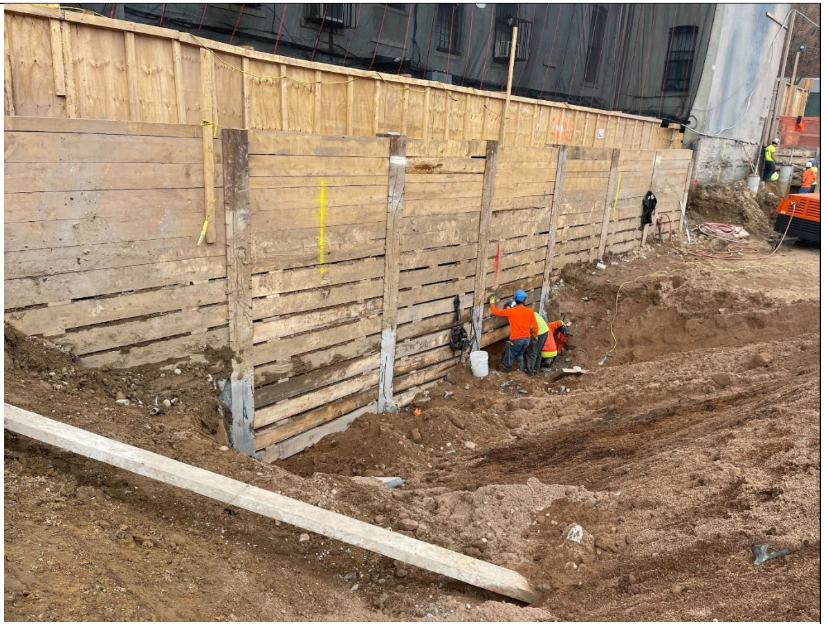
Photo 3 – View of excavated area.
