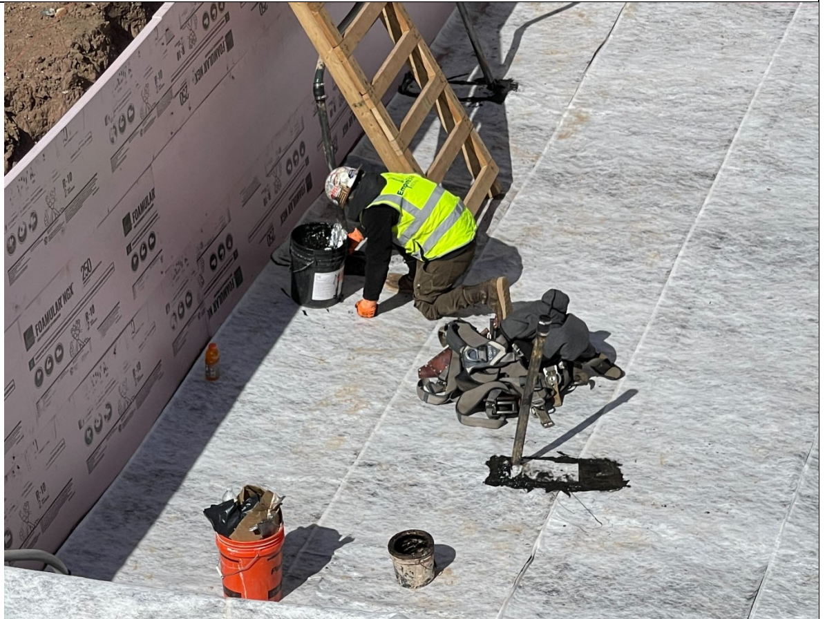
Photo 2 – View of W.R. Meadows Sealtight Waterproofing System being installed within the elevator pit.
