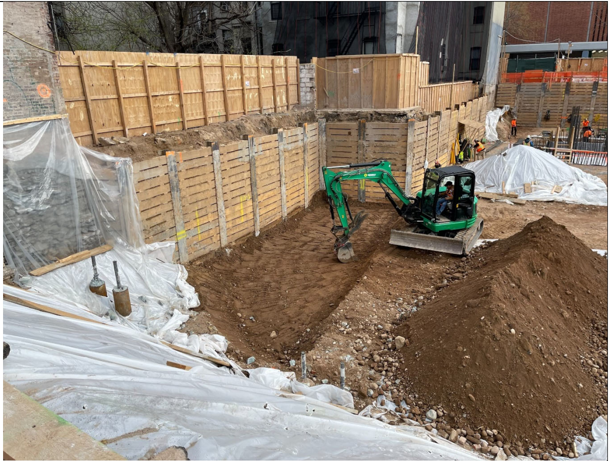
Photo 1 – View of excavated Grid 1.
