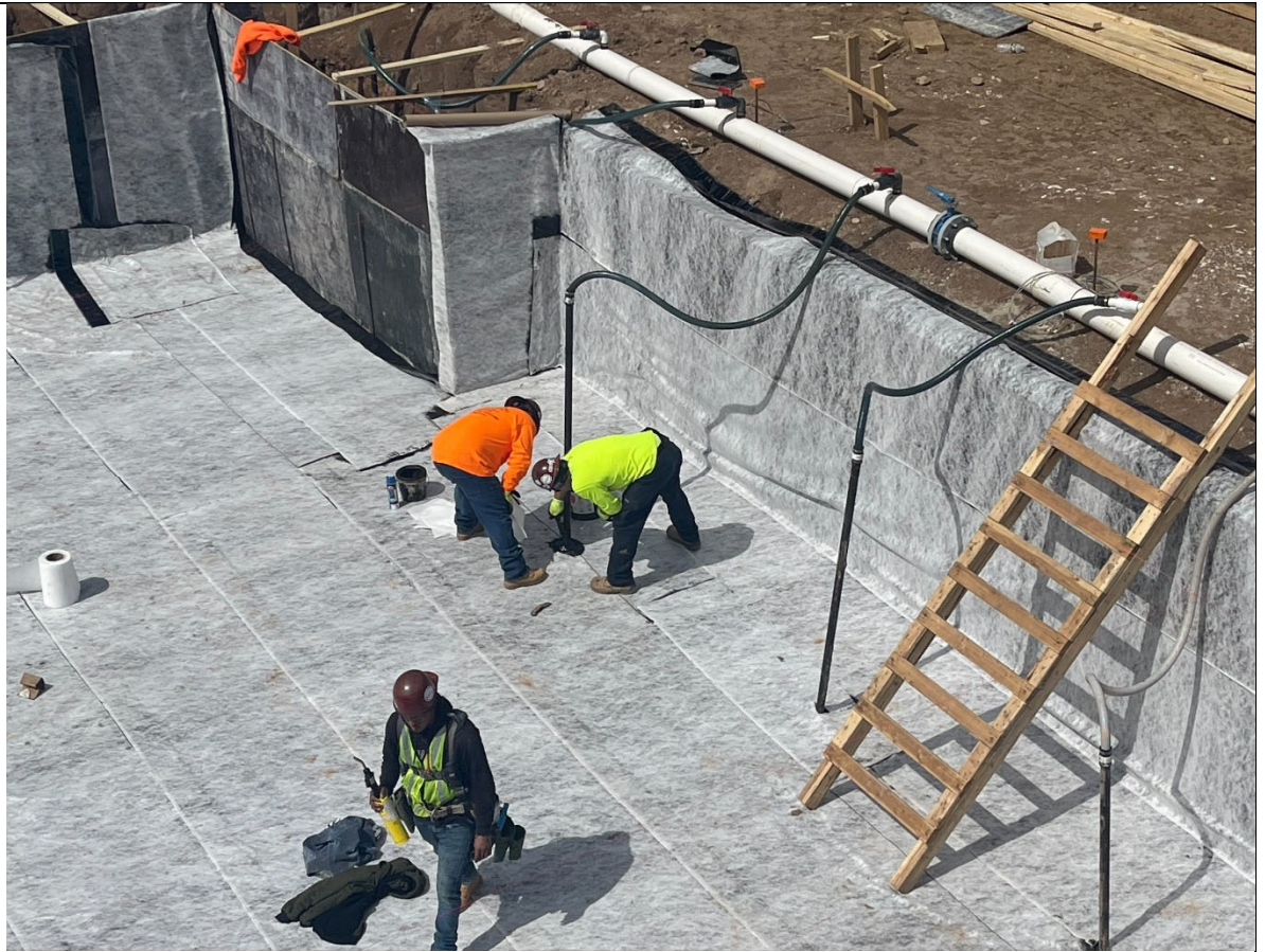
Photo 3 – View of W.R. Meadows Sealtight Waterproofing System being installed within the elevator pit.
