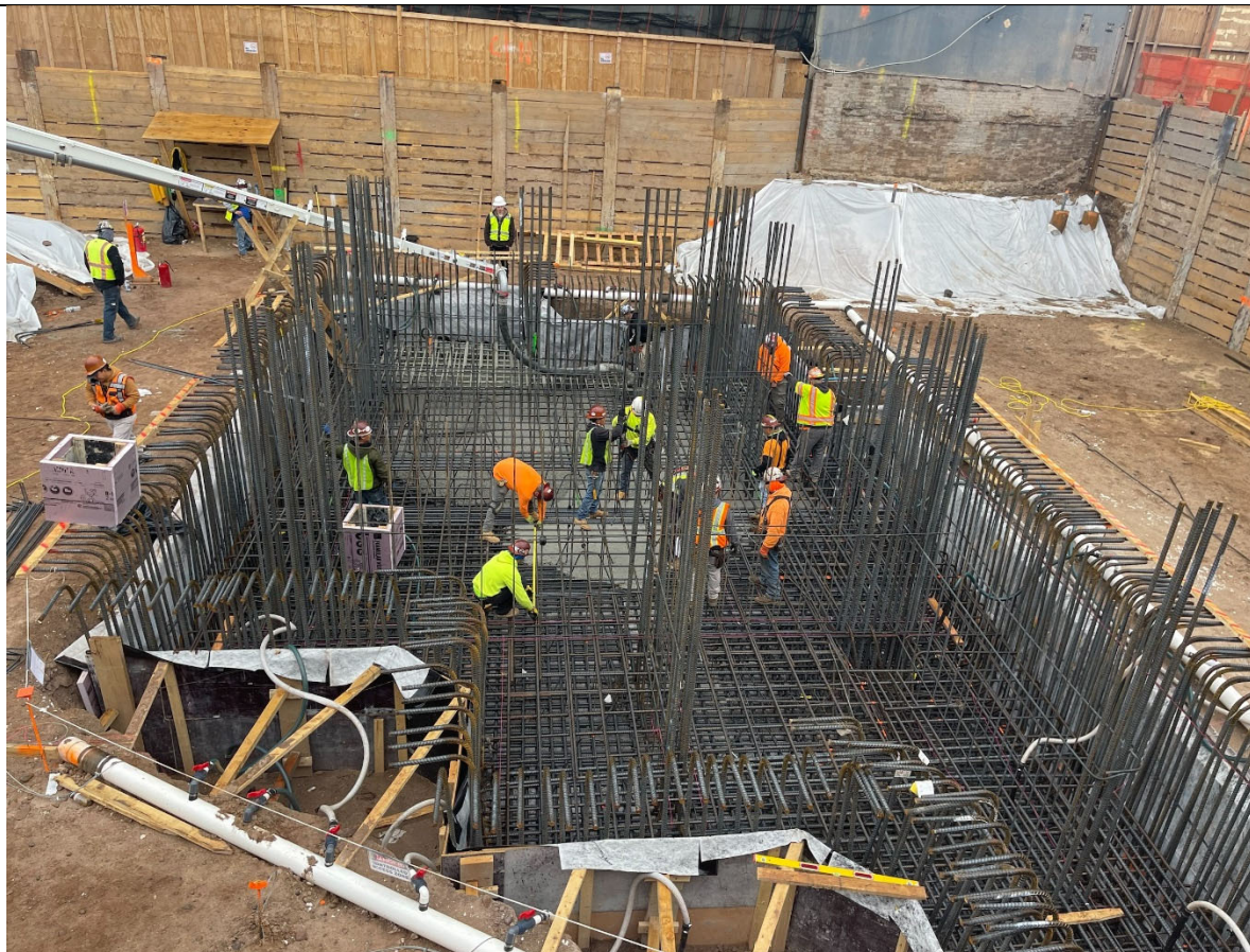
Photo 1 – View of rebar work within the elevator pit.
