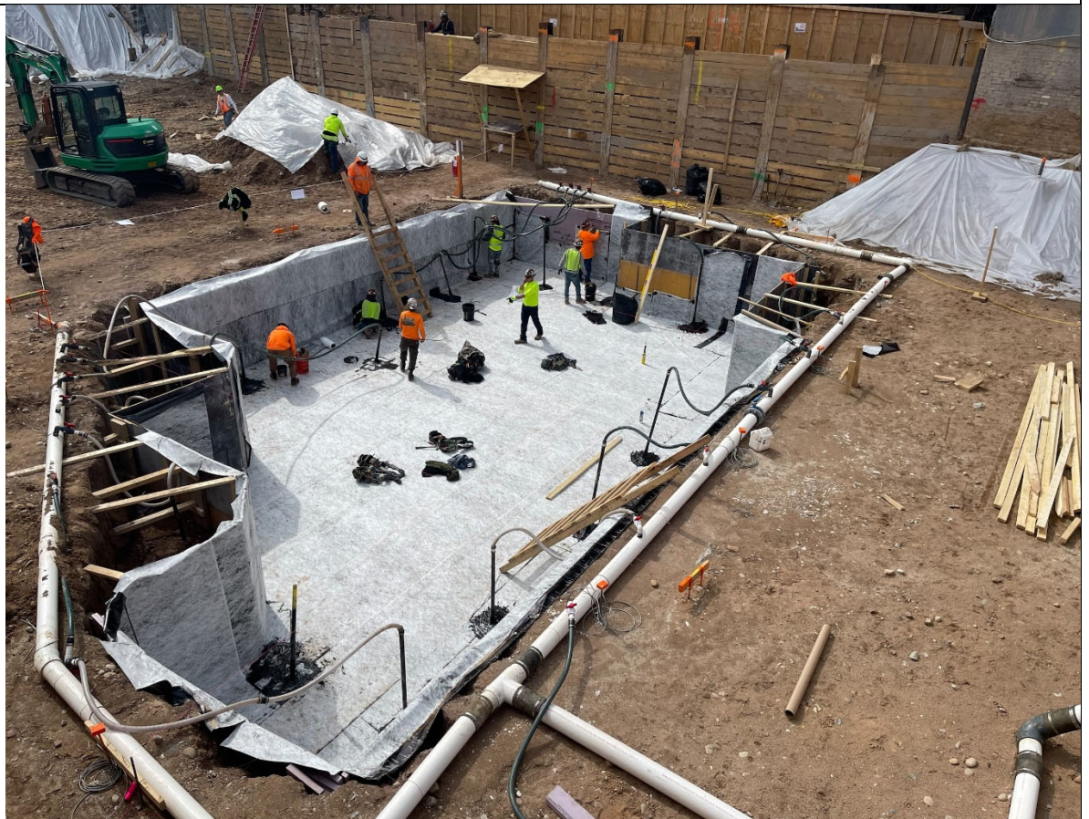
Photo 4 - View of W.R. Meadows Sealtight Waterproofing System being installed within the elevator pit.
