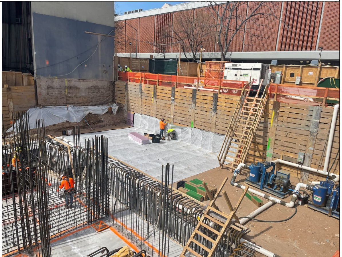
Photo 4 - View of waterproofing installation.
