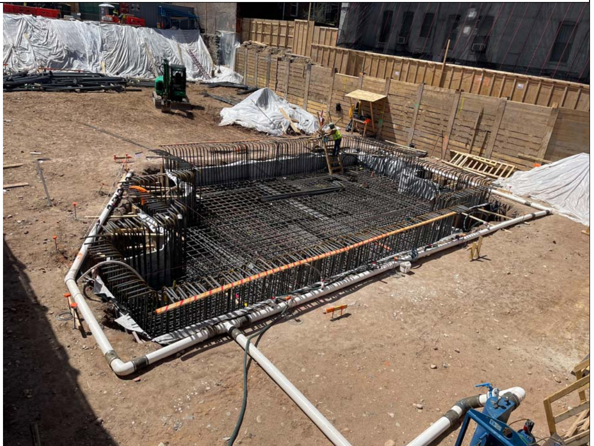
Photo 4 - View of rebar work within the elevator pit.
