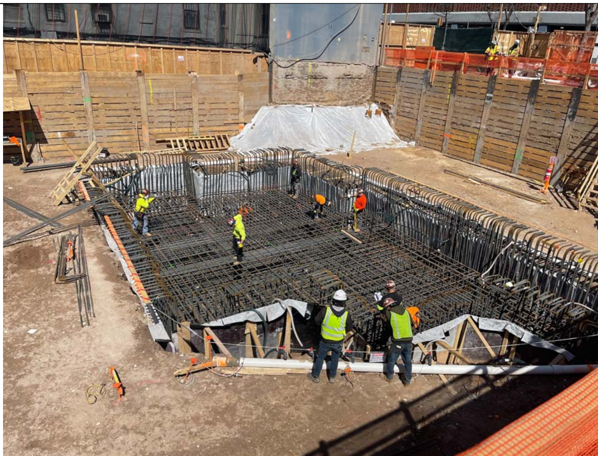
Photo 2 – View of rebar work within the elevator pit.
