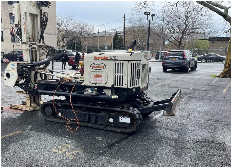
Photo 3: Looking north, Geoprobe 7822DT breaks down during borehole drilling at location B2.
