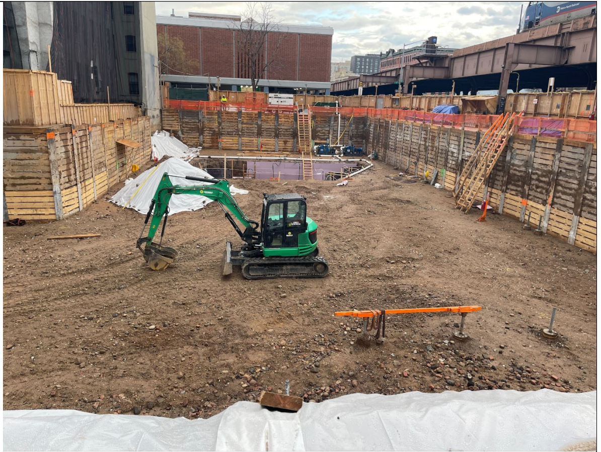
Photo 1 – V Overall Site view from 126 th Street.
