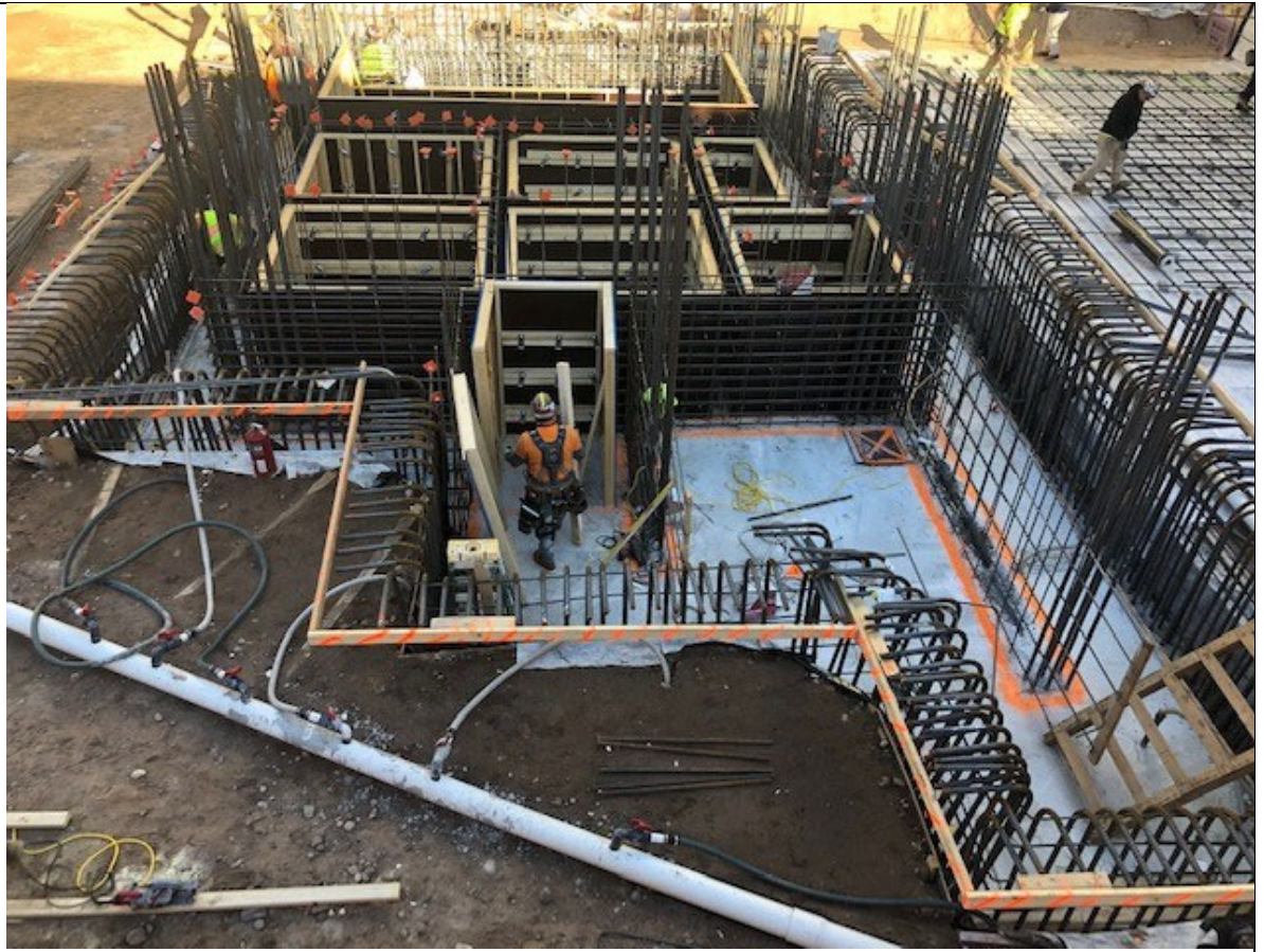
Photo 1 – View of building construction.
