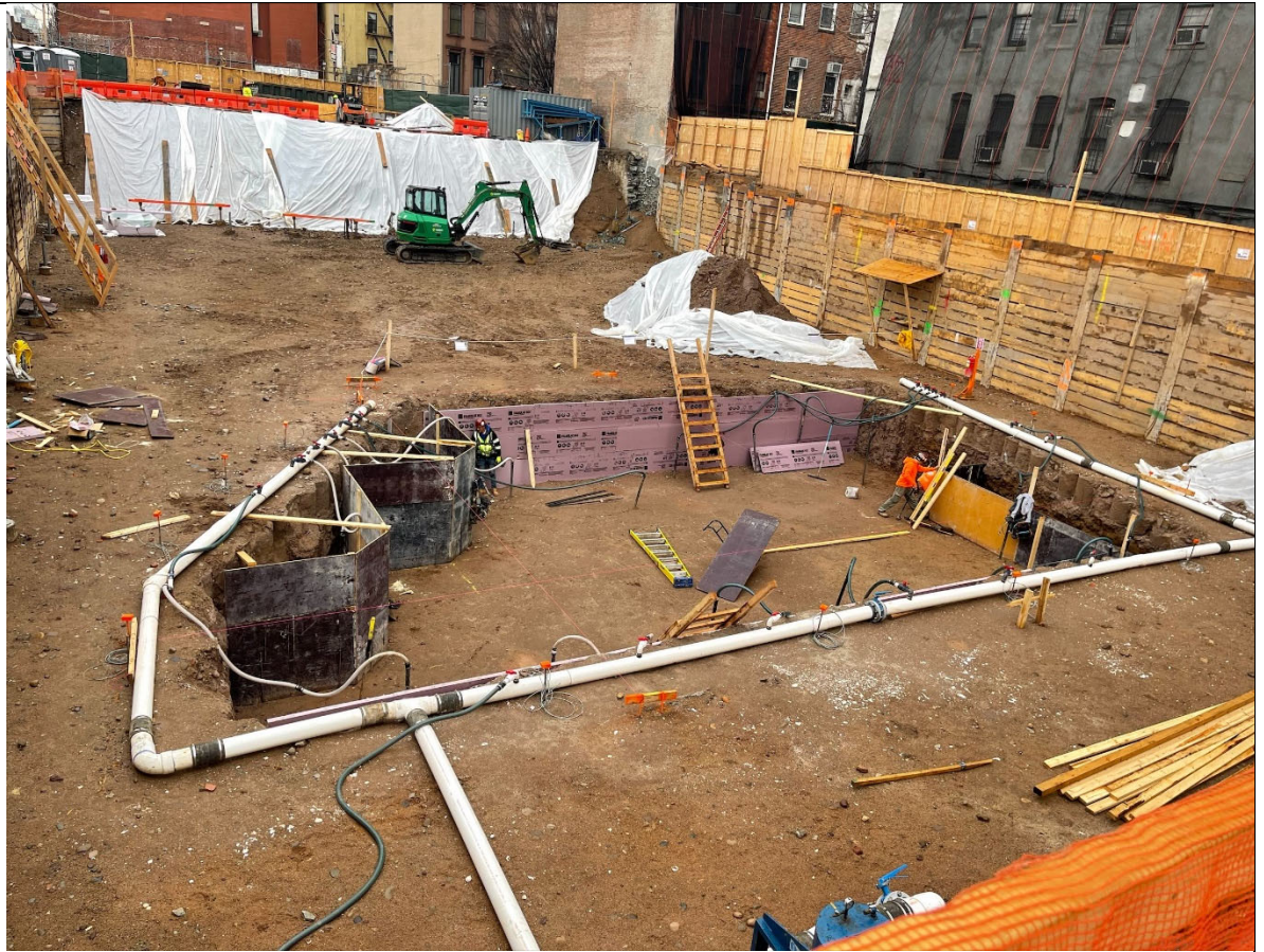
Photo 3 – Overall Site view from 127 th Street.
