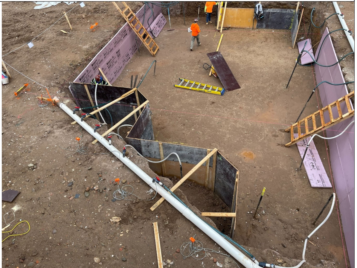
Photo 2 – View of dewatering equipment and work within the elevator pit.
