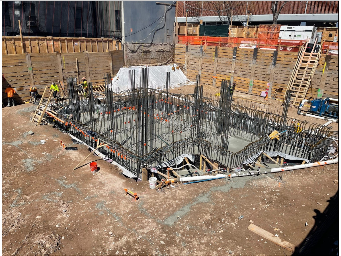
Photo 3 – View of rebar work within the elevator pit.
