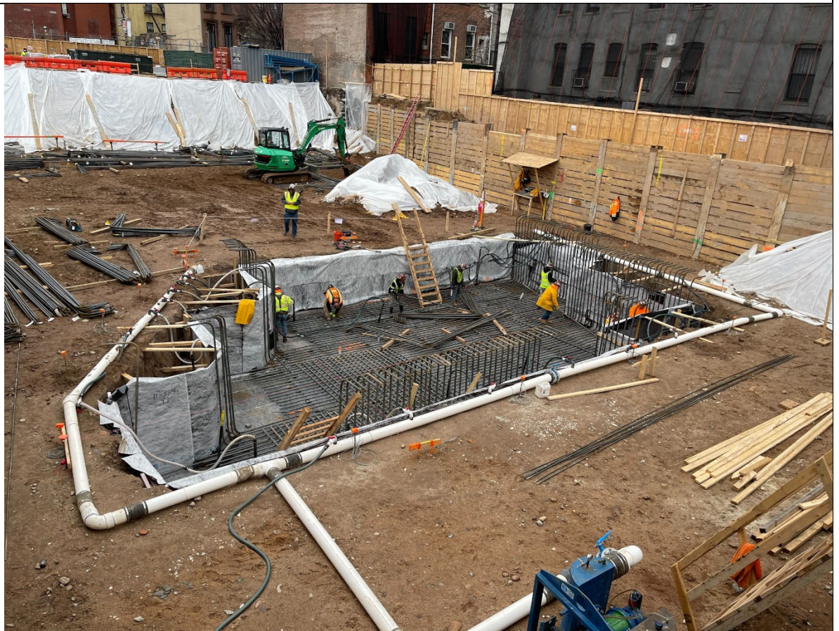
Photo 2 – View of rebar work within the elevator pit.
