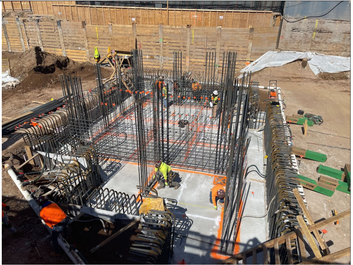
Photo 3 – View of poured concrete within the elevator pit.
