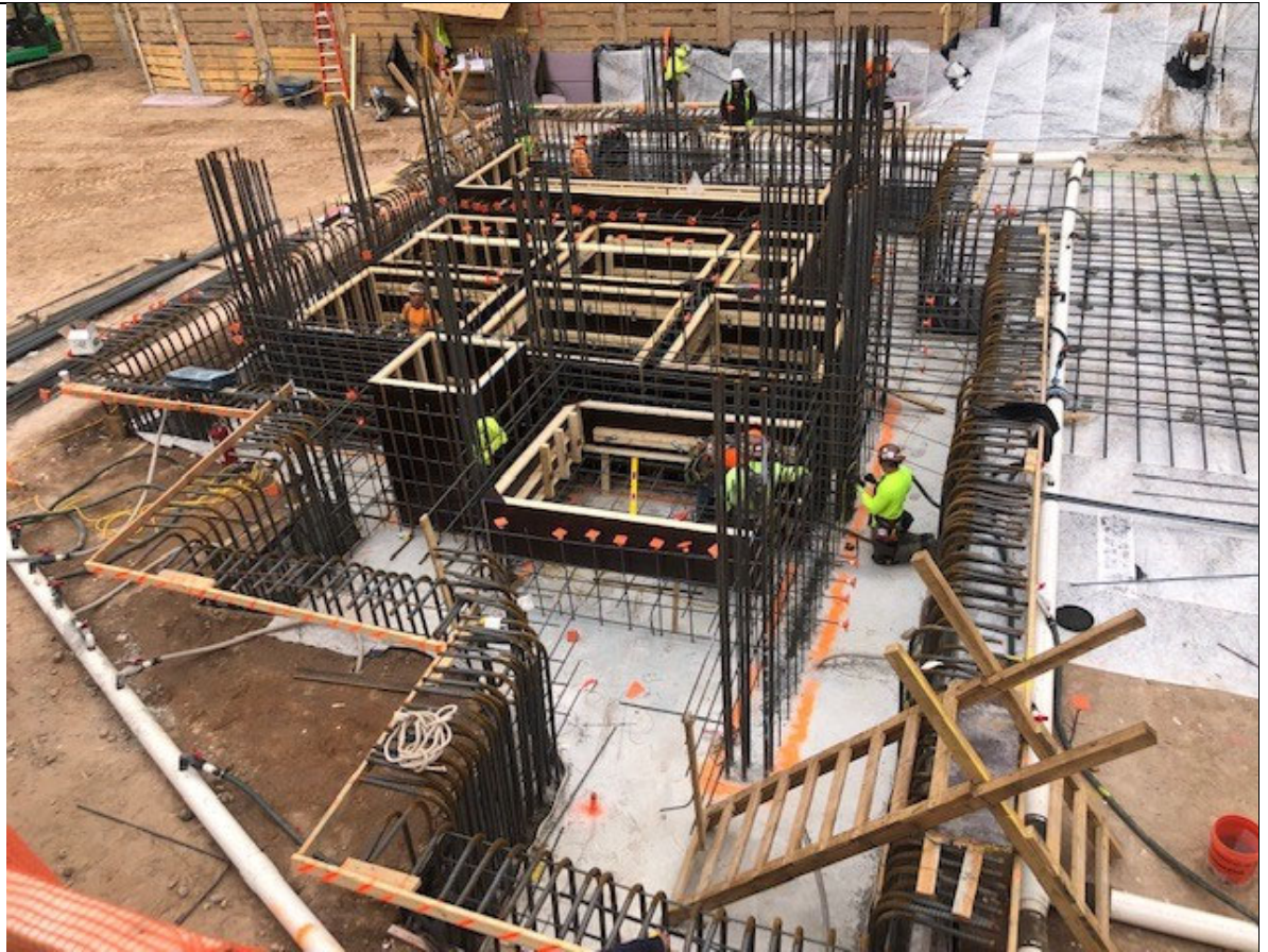
Photo 3 - View of building construction.
