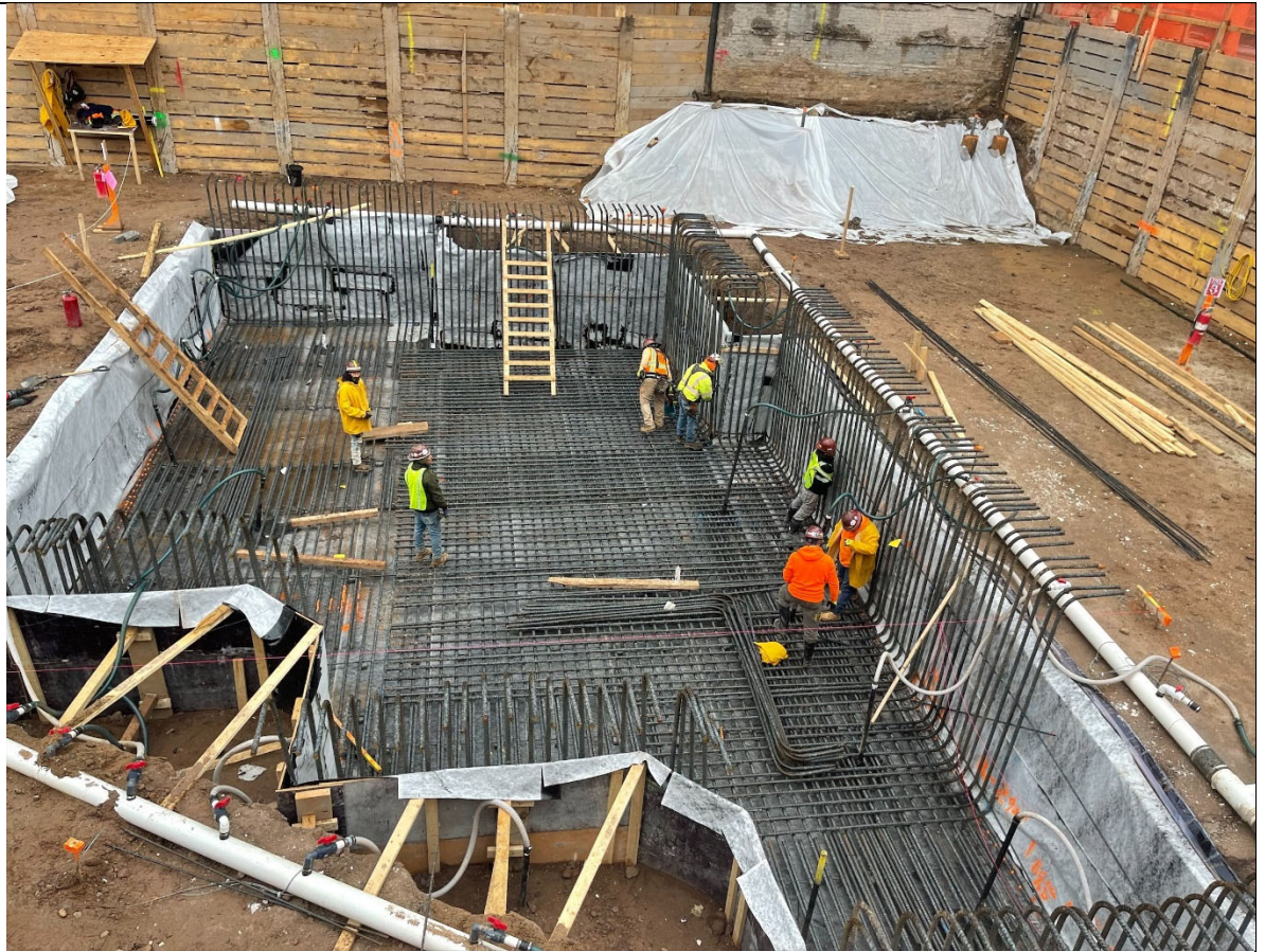
Photo 1 – View of rebar work within the elevator pit.
