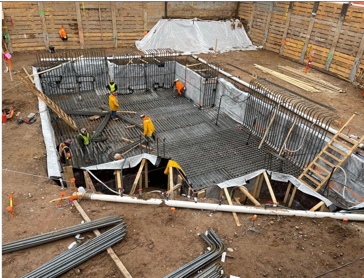
Photo 3 – View of rebar work within the elevator pit.
