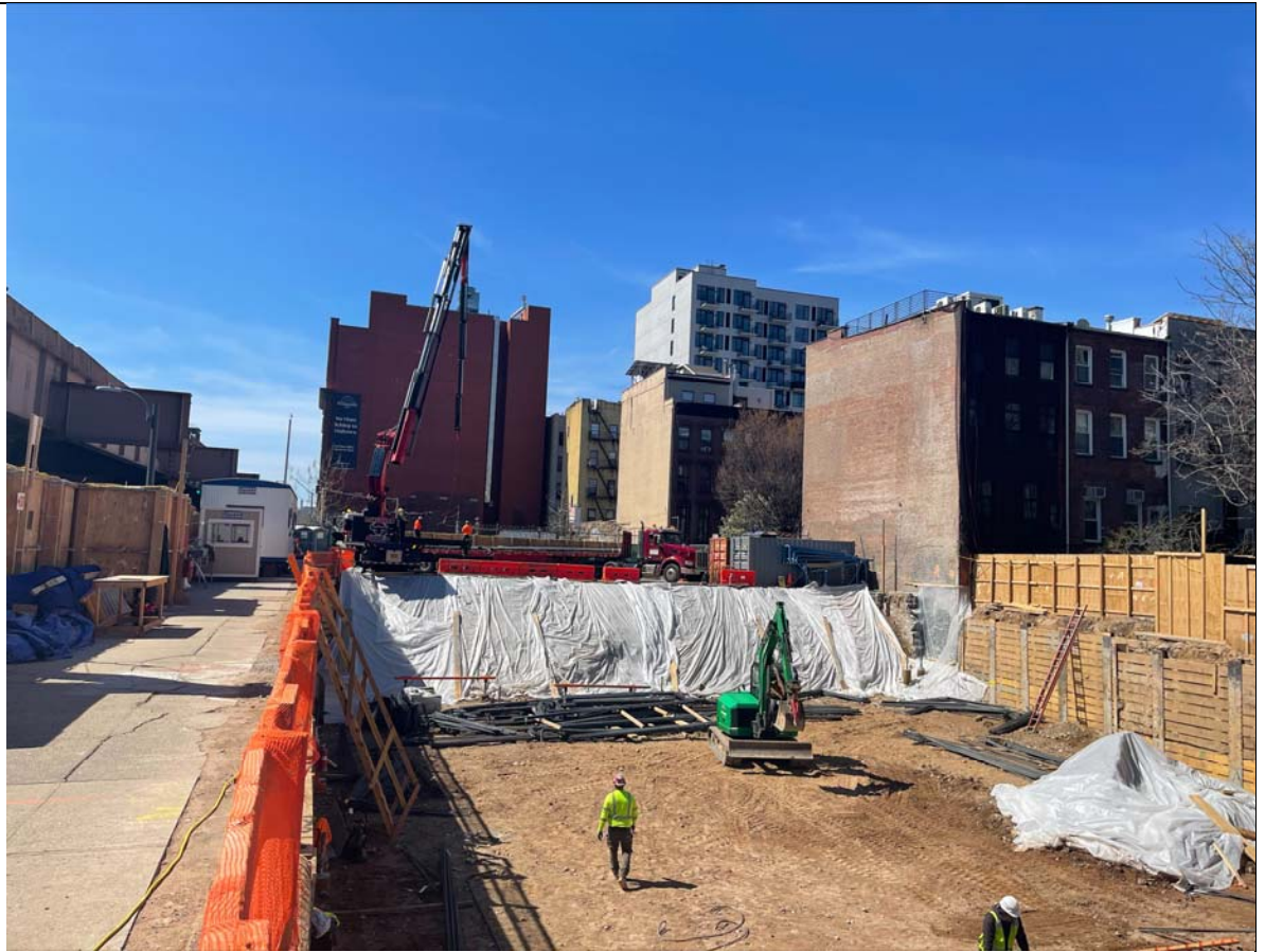
Photo 3 – Overall Site view.
