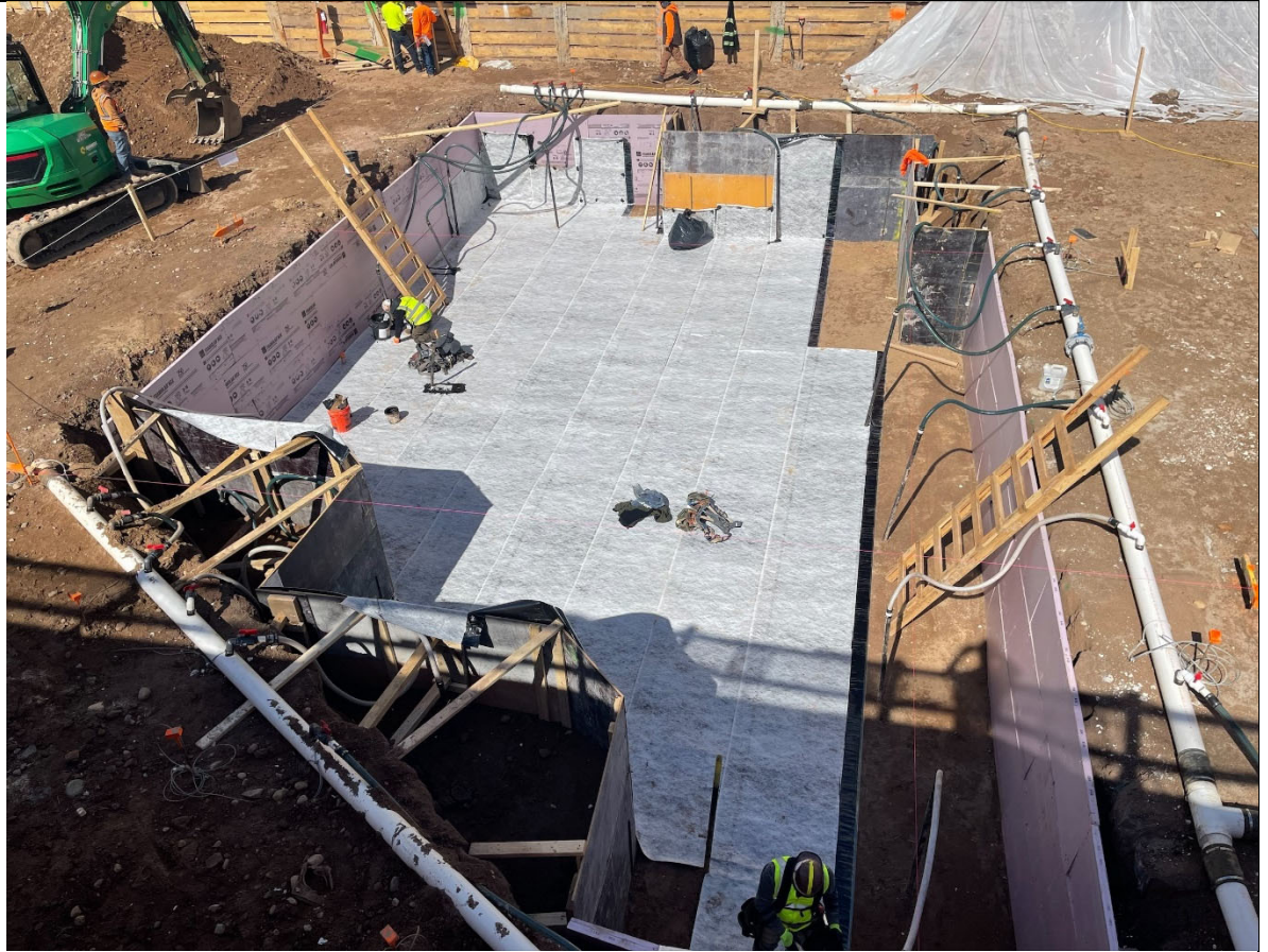
Photo 1 – View of W.R. Meadows Sealtight Waterproofing System being installed within the elevator pit.
