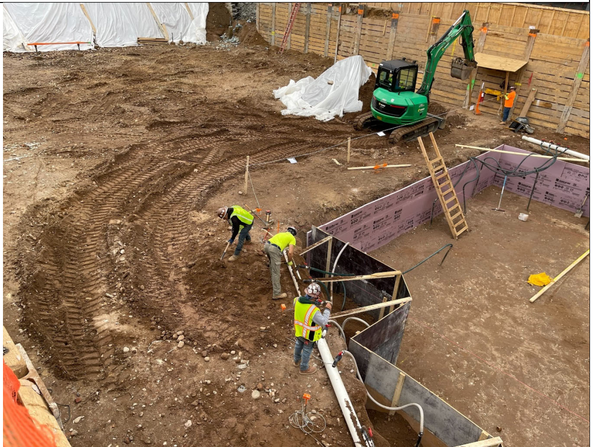
Photo 4 - View of formwork within elevator pit.
