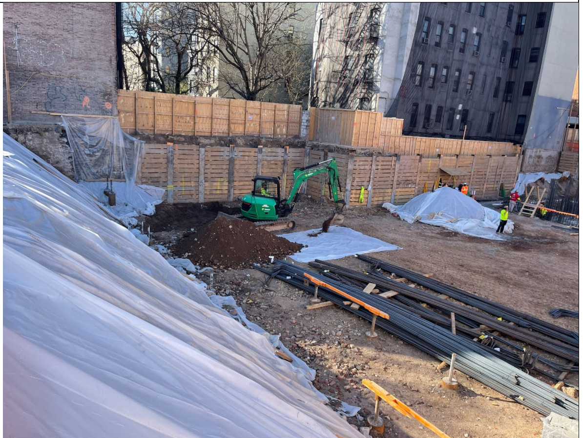
Photo 4 - View of excavation of Grid 1 to 15' for EP 1.
