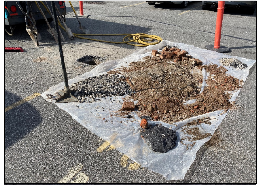
2. Photo Taken 02.12.2020. Pre-clearing activities showing asphalt and bricks removed from the hole and segregated from the soil
