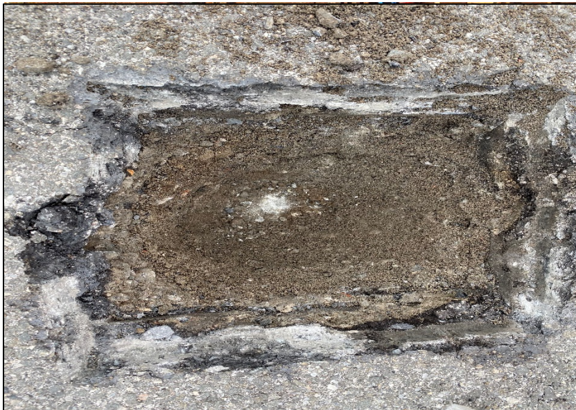
3. Photo Taken 02.12.2020. Photo showing cleared hole after asphalt layer was removed
