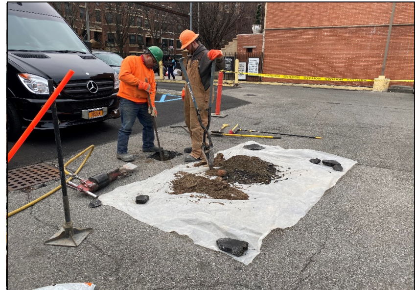
4. Photo Taken 02.12.2020. Drilling crew performing pre-clearing activities after asphalt layer was removed
