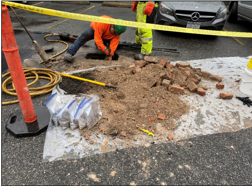
1. Photo Taken 02.11.2020. Pre-clearing activities for soil boring installation
