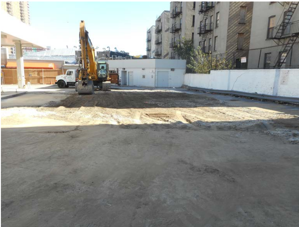
UST Tank Field Excavation Backfilled
