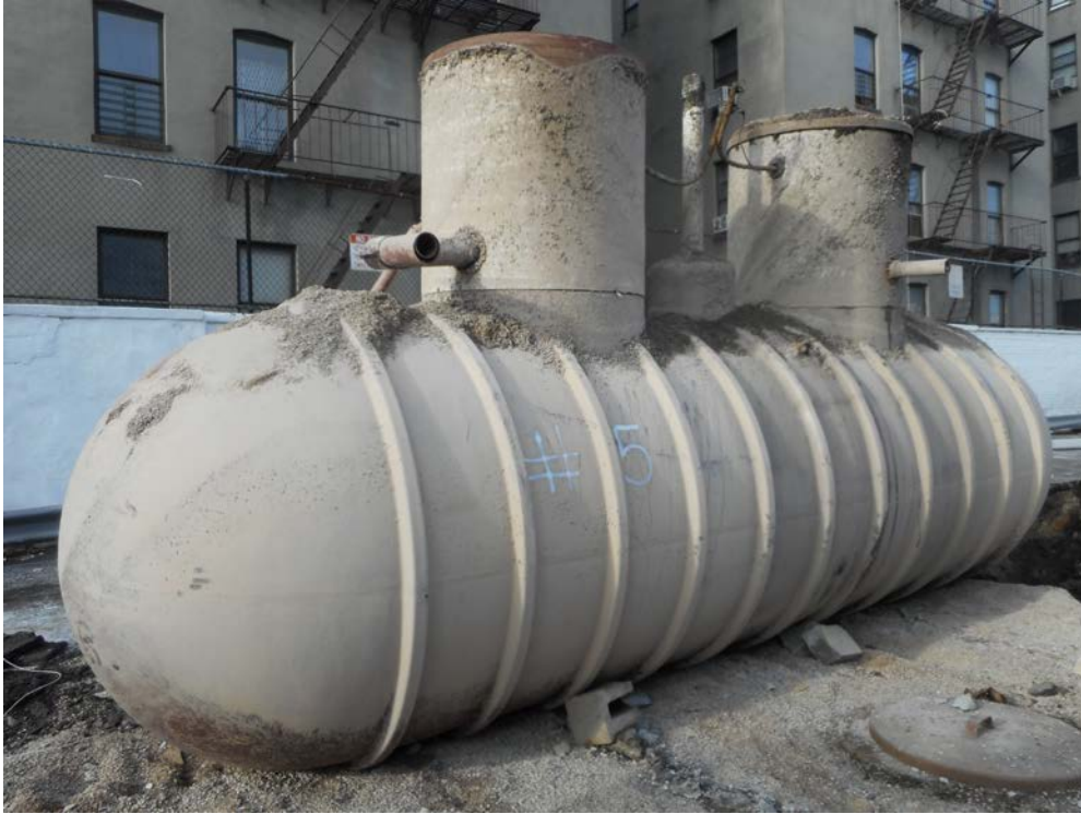
Condition of Tank #5
