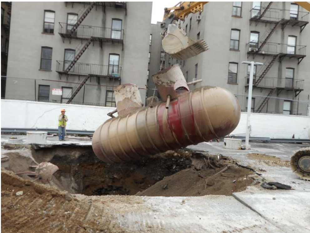
Removal of Tank #4
