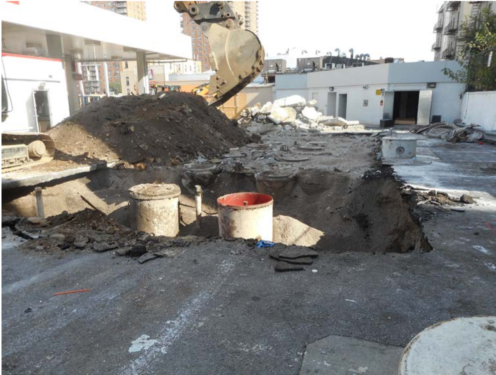
Excavating Soil from UST Tank Field
