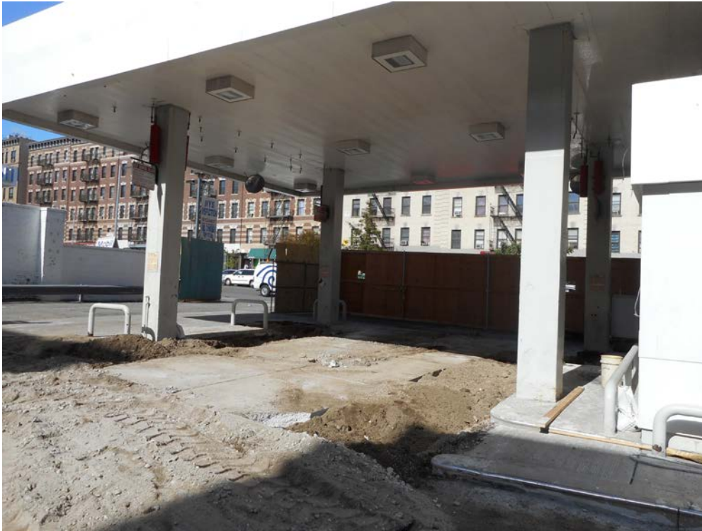
Product Piping Excavation Areas
