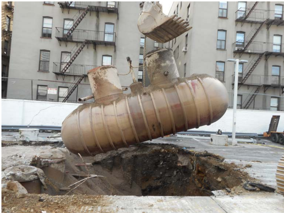
Removal of Tank #5
