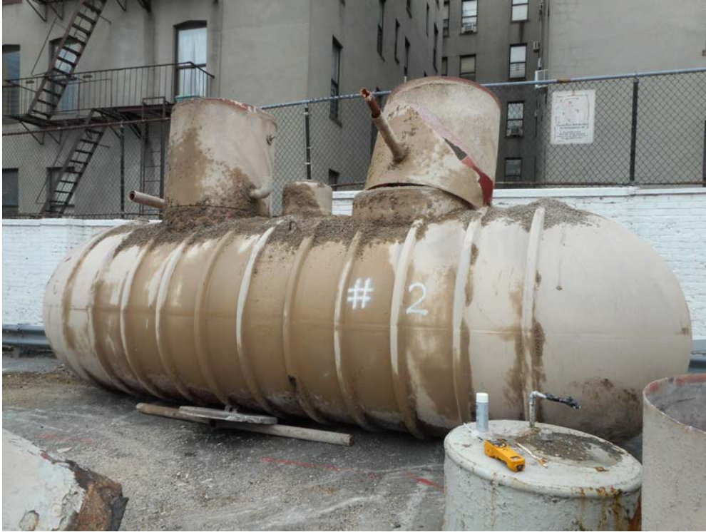
Condition of Tank #2
