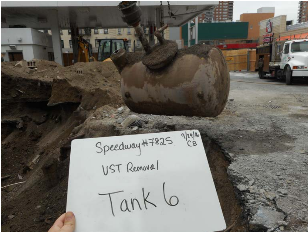
Removal of Tank #6 (Waste-water UST)
