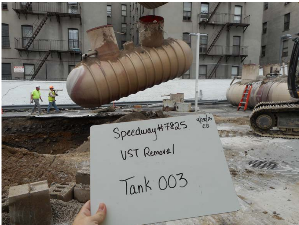
Removal of Tank #3
