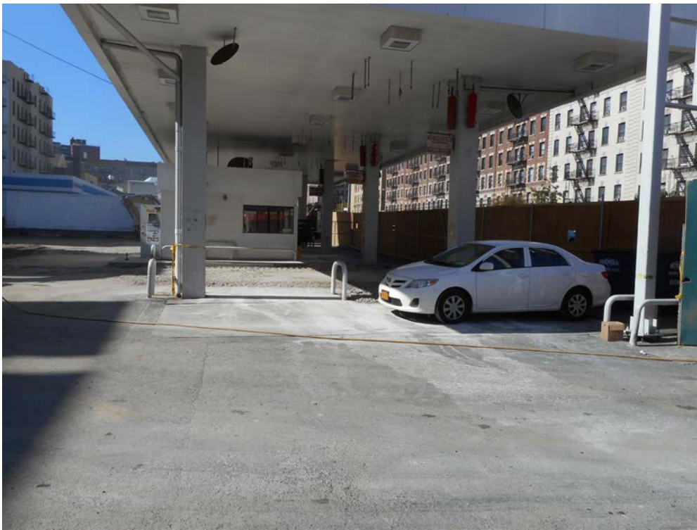
Product Piping Excavations/Dispenser Islands Backfilled
