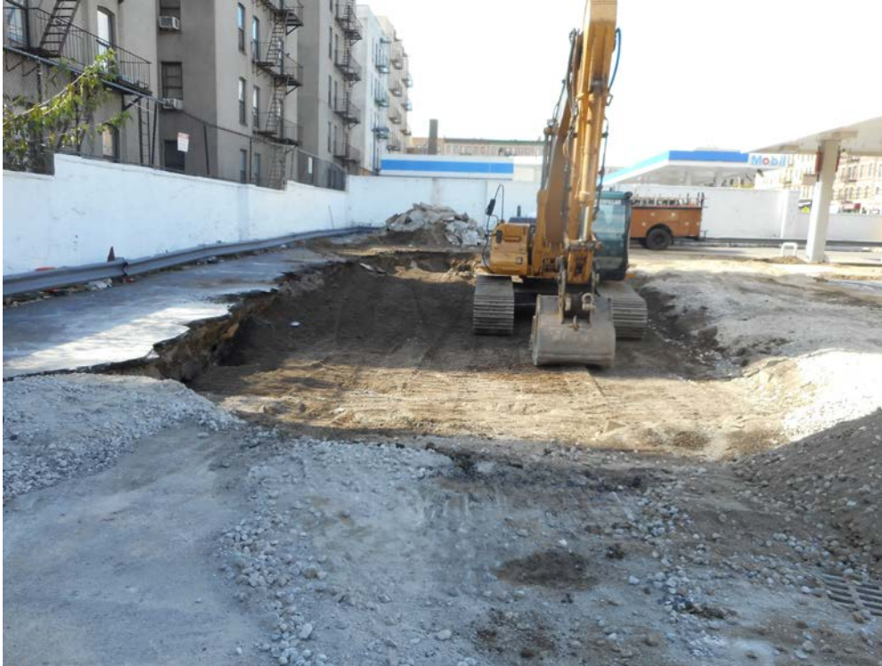
Backfilling/Tamping of UST Tank Field Excavation
