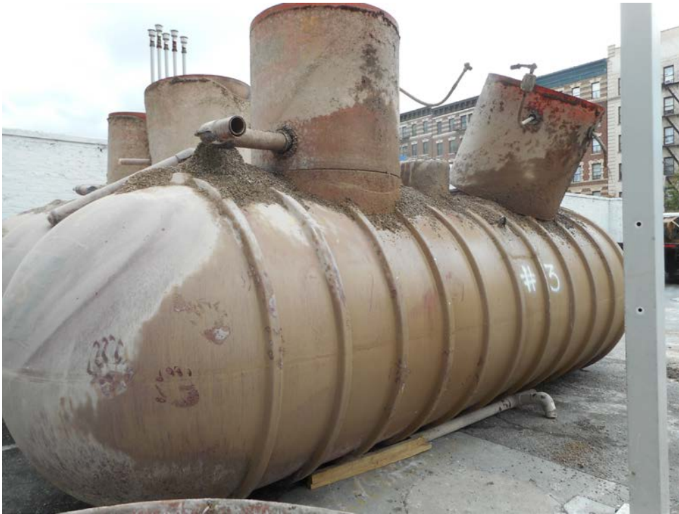
Condition of Tank #3
