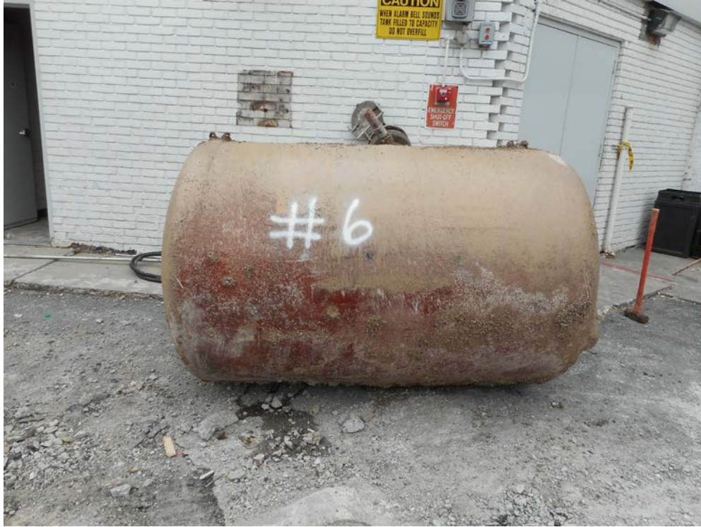
Condition of Tank #6 (Waste-water UST)
