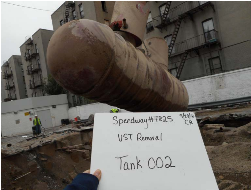
Removal of Tank #2
