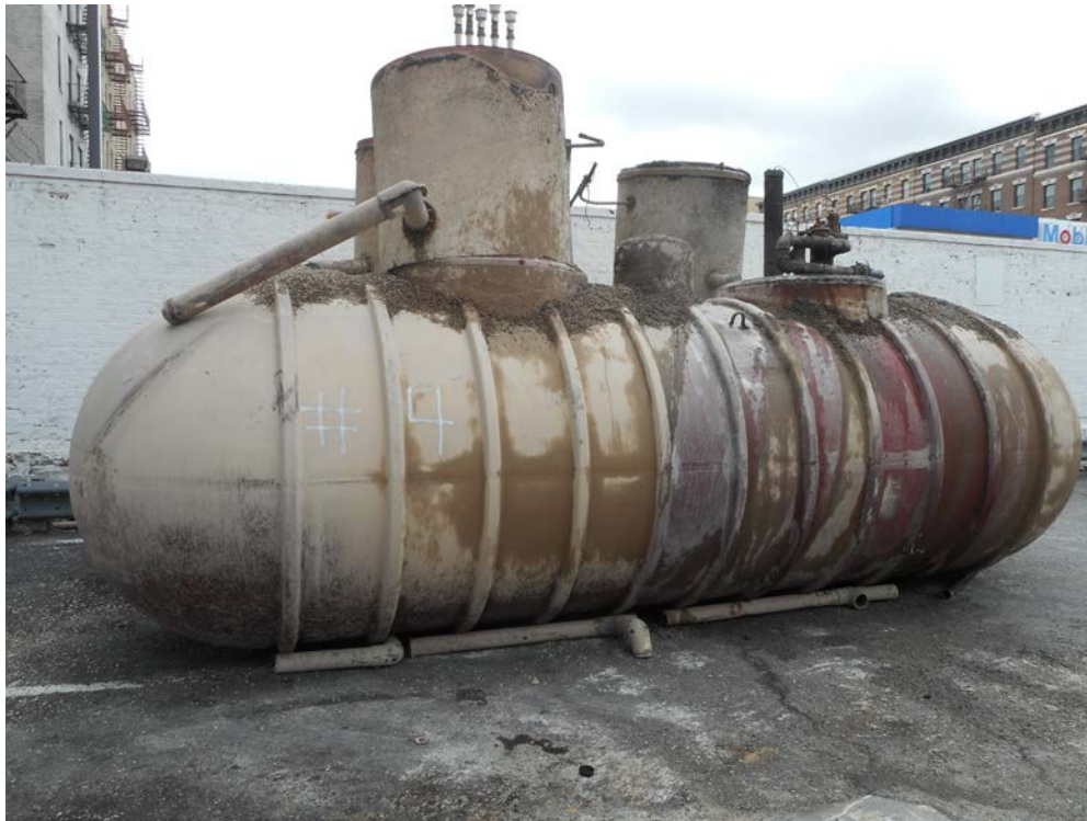
Condition of Tank #4
