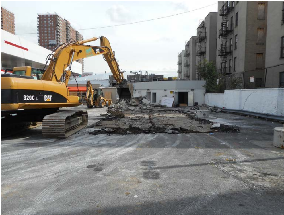
Removing Concrete Mat above UST Tank Field
