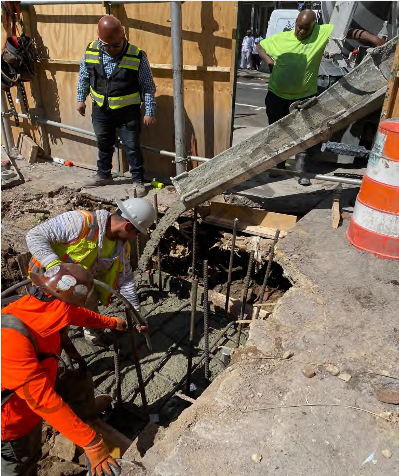
Picture 1 shows 7000 PSI concrete cast at Pile cap PC-1A base of Buttress 24.
