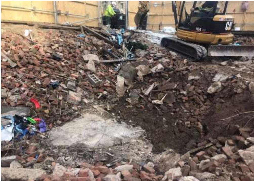
Photo 14: Remaining stained soil and clean concrete pad below AST staging area, facing northeast. 15 March 2022.
