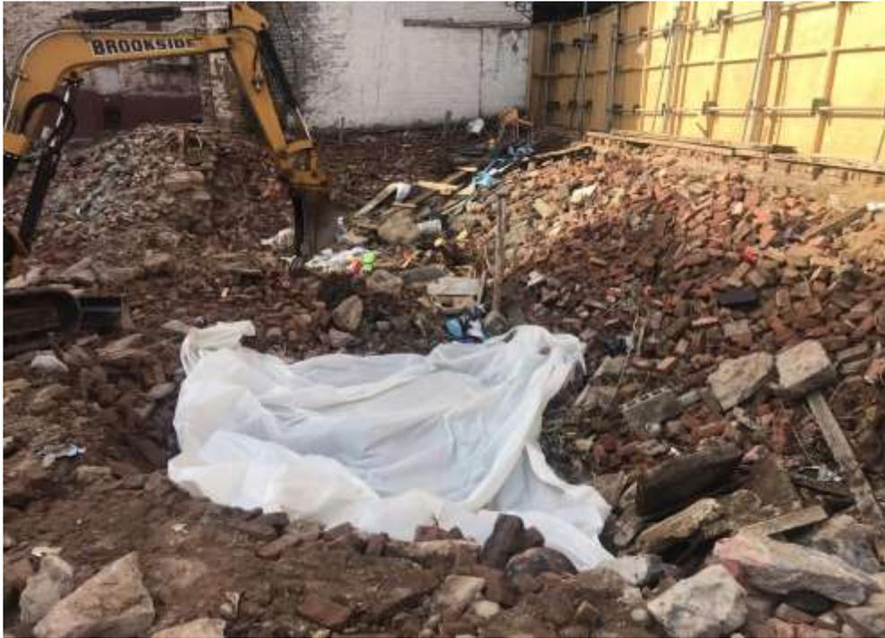
*Photo 15:* Placement of polysheeting over AST staging area and stained soil as a demarcation layer for future remediation, facing west. 15 March 2022.
