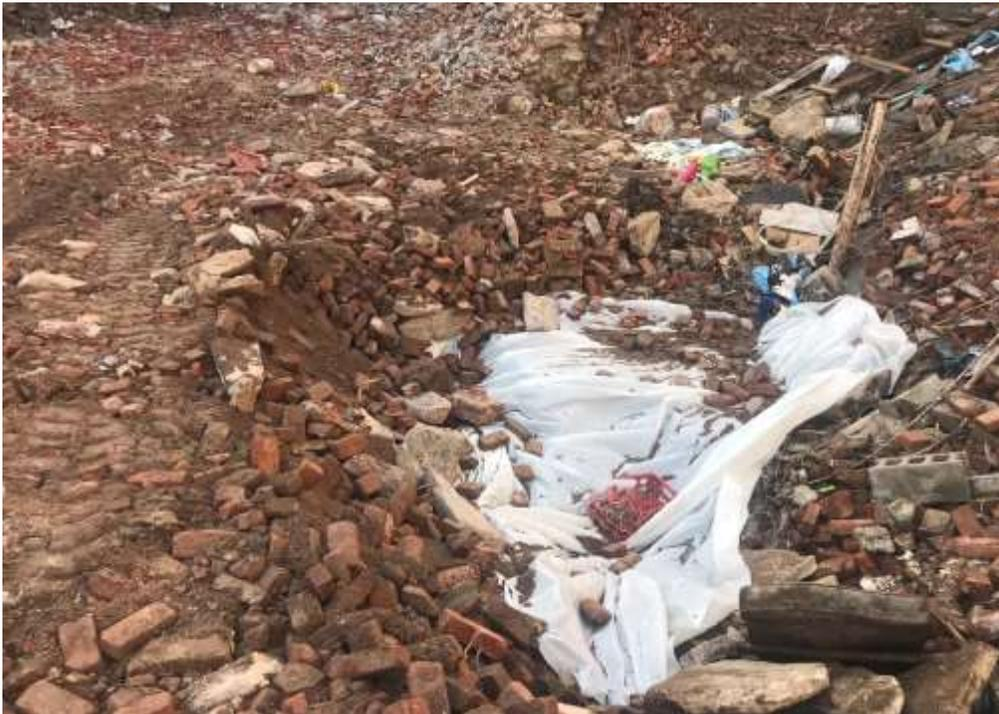
*Photo 16:* Placement of polysheeting over AST staging area and stained soil as a demarcation layer for future remediation, facing west. 15 March 2022.
