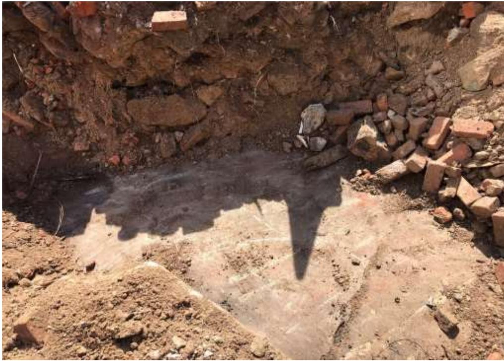
Photo 7: Concrete slab below original AST location, facing southeast. 14 March 2022.
