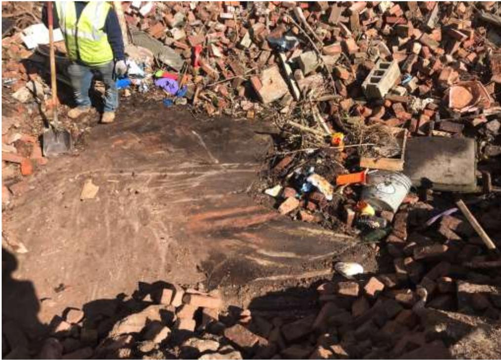
Photo 11: Stained concrete below AST staging area, facing north. 15 March 2022.
