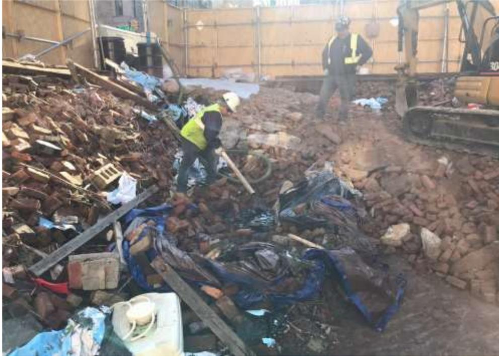
*Photo 9:* Removal of remaining product and impacted demolition debris previously stockpiled and staged on tarpaulins, facing east. 15 March 2022.
