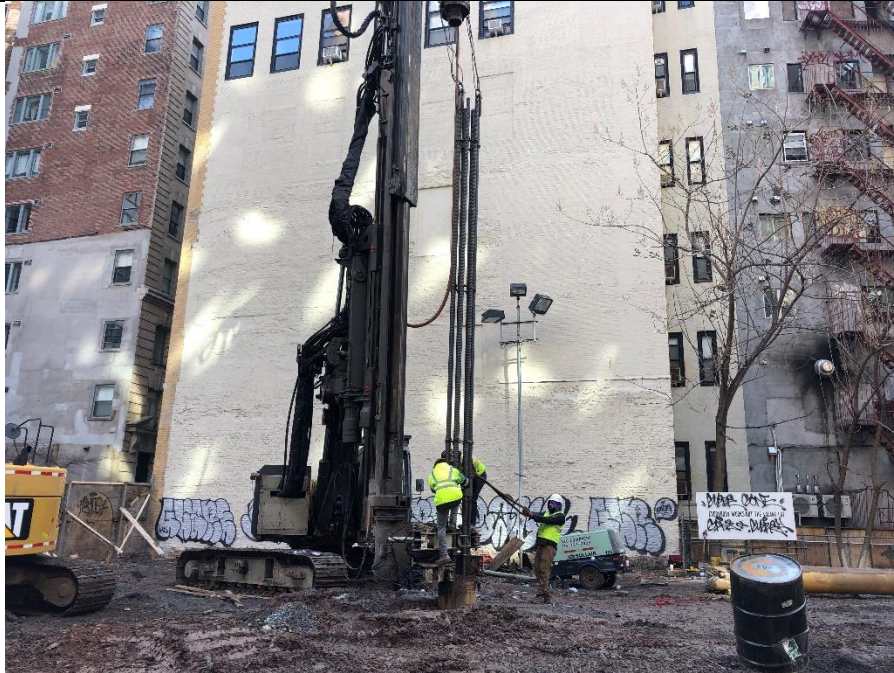
Contractor placing reinforcement for Caisson 1 on 10 March 2022.
