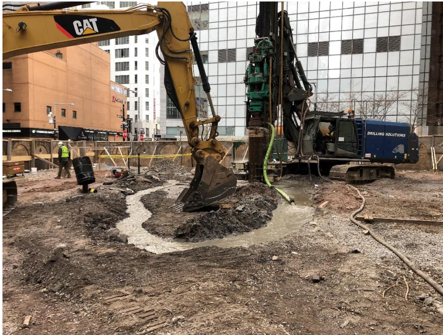
Photo 1: Contractor drilling permanent casing for Caisson 1, looking north.
