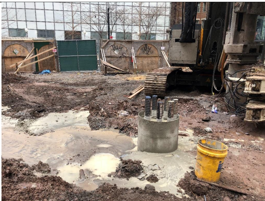
View of completed Caisson 1 on 10 March 2022.
