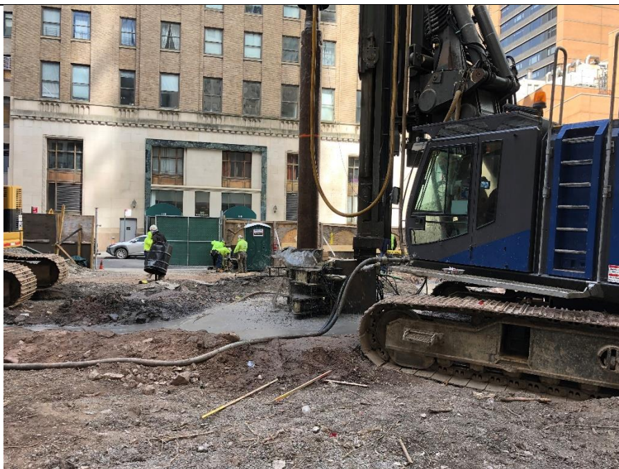
Contractor starting to drill rock socket for Caisson 1 on 8 March 2022.
