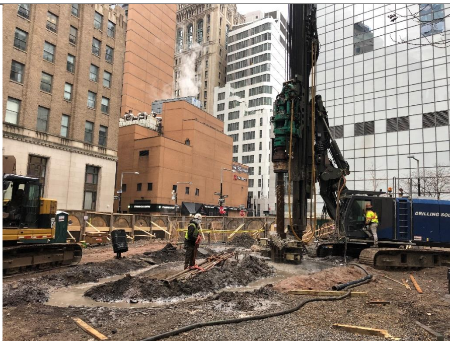
Contractor continuing to drill rock socket for Caisson 1 on 9 March 2022.
