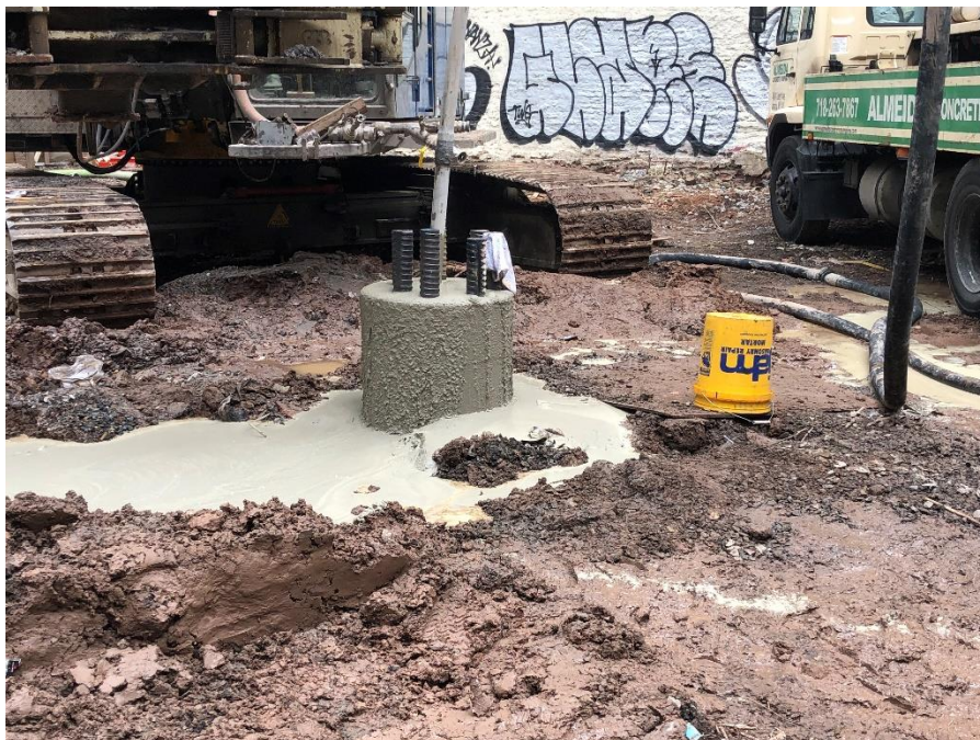
Photo 2: Contractor placing grout for Caisson 1, looking east.
