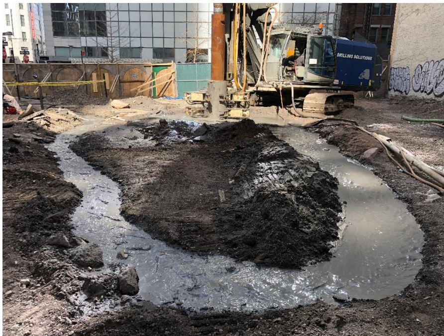
Photo 2: Contractor constructing rock socket for Caisson 1, looking north.
