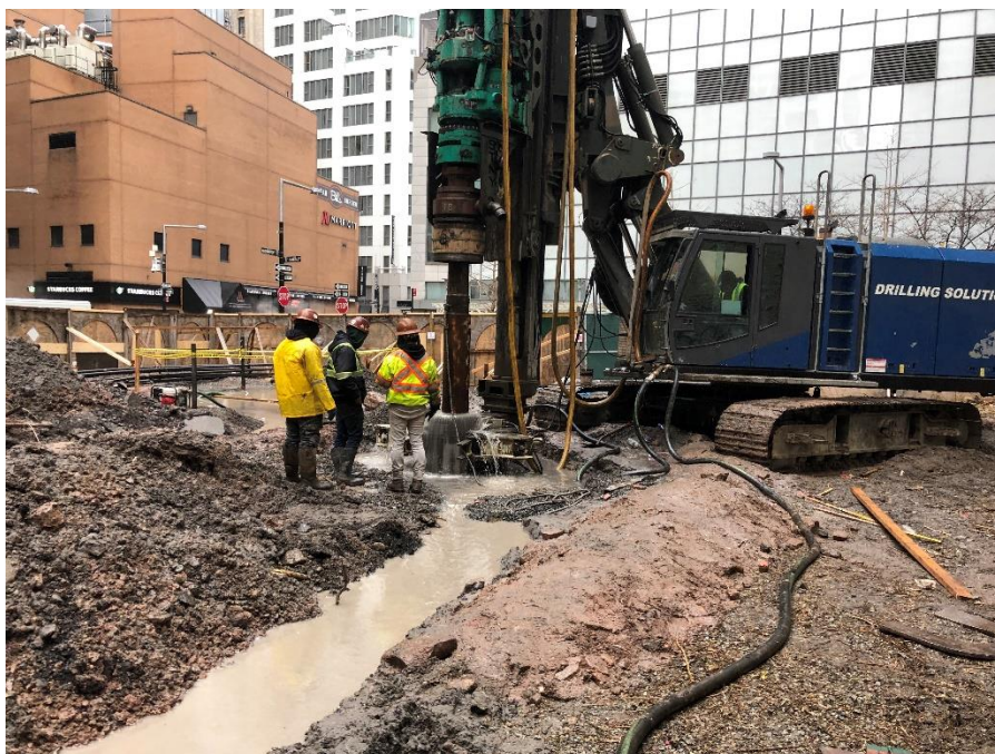
Photo 2: Contractor constructing rock socket for Caisson 1, looking northwest.
