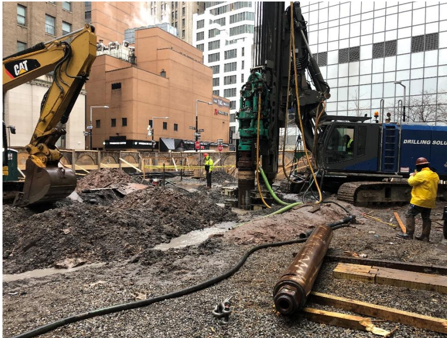
Photo 1: Contractor drilling permanent casing for Caisson 1, looking northwest.
