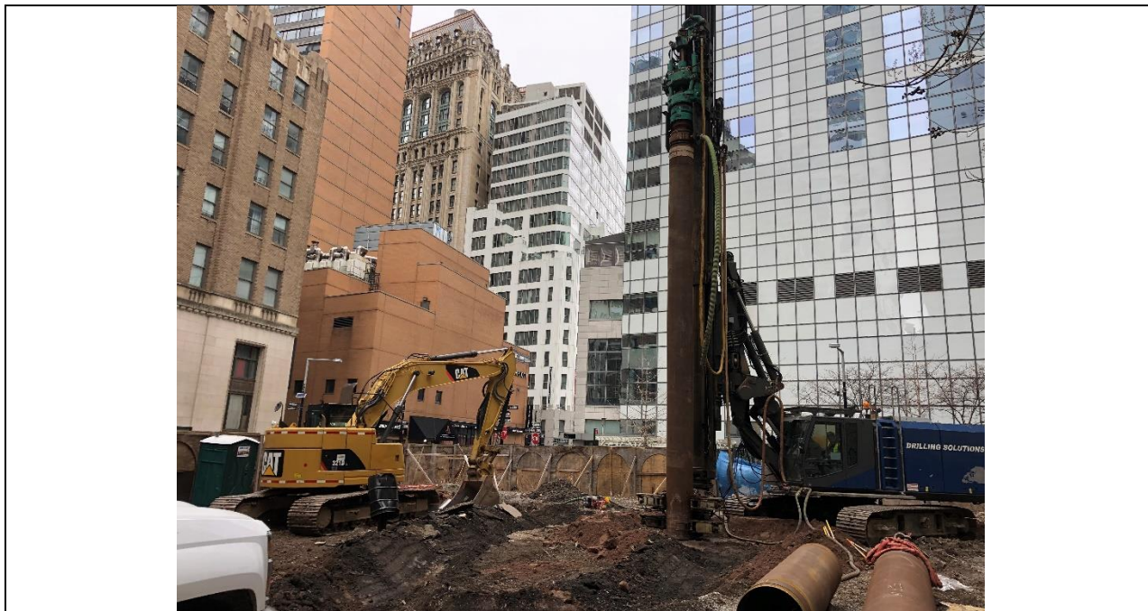
Contractor starting to drill permanent casing for Caisson 1 on 1 March 2022.
