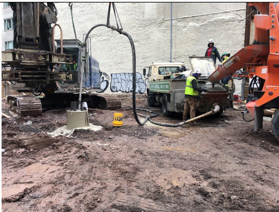
Contractor grouting Caisson 1 on 10 March 2022.
