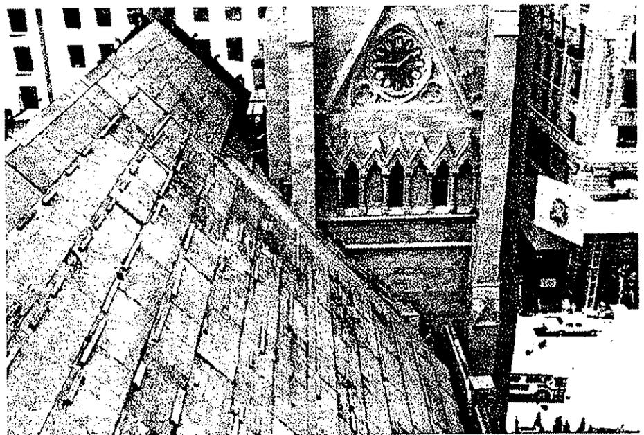
Figure 4. Dropped equipment, tools, and materials all present risks when new construction rises above neighboring historic structures. In this case, the historic slate roof was completely covered with sheets of exterior grade plywood. Photo: National Park Service files.
