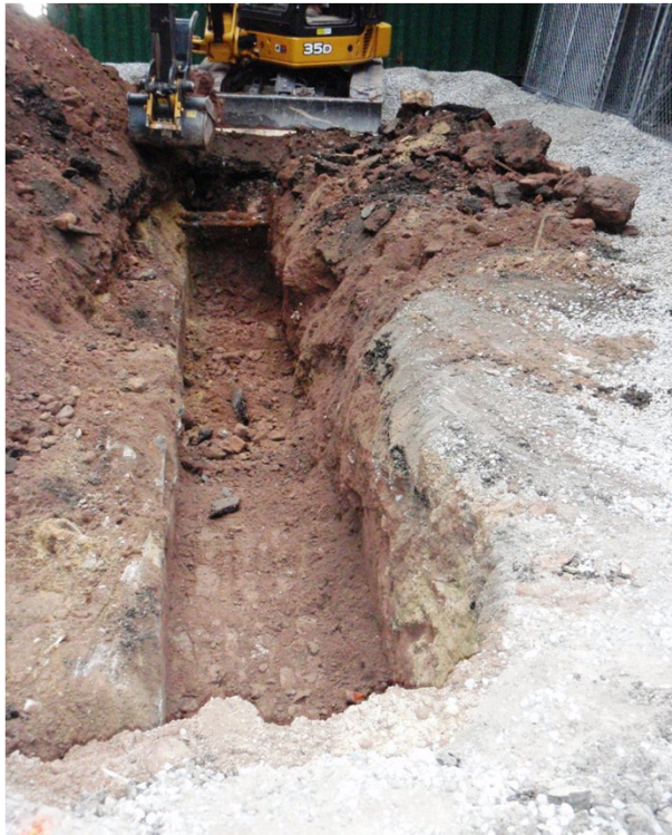
Photo 5: The test pit extended along the length of the western edge of the concrete vault. Facing south. 11 January 2012.
