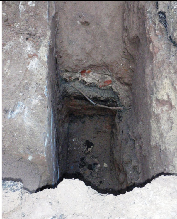
Photo 4: View of the southern sidewall at the location of SS-1. 11 January 2012.
