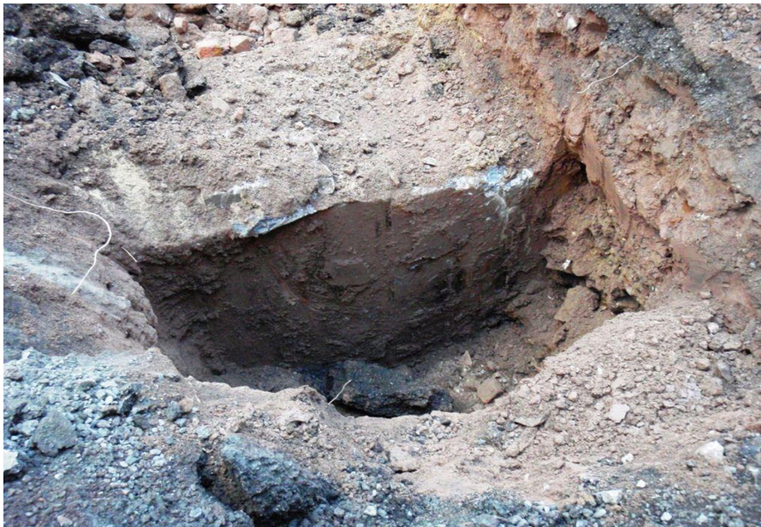
Photo 2: A concrete structure was encountered while performing test pitting to locate the suspected UST. Facing east. 11 January 2012.
