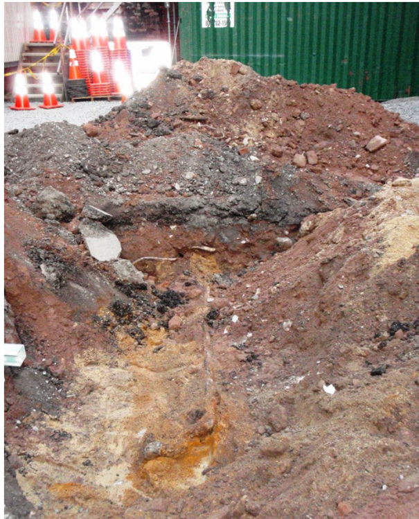
Photo 3: Piping connected to the concrete structure was identified. Facing south. 11 January 2012.
