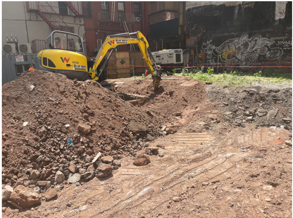
Photo 2: View of Urban removing concrete in the eastern part of WC05_0-5 (left) and the top of the UST concrete encasement (right).
