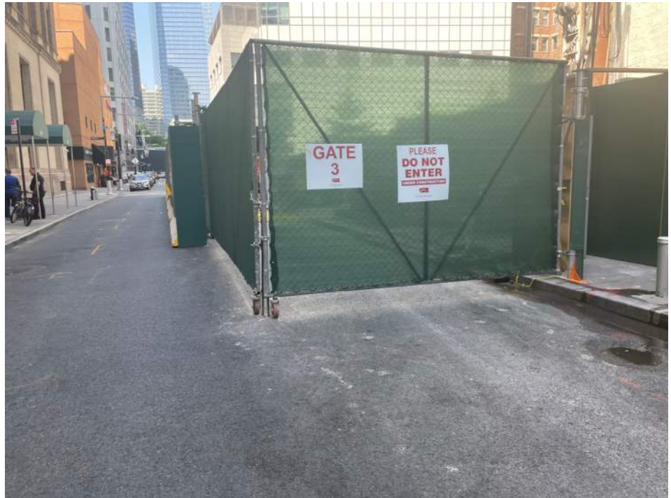
Photo 5: View of the entrance/exit of the site along Washington Street at the end of the work day (facing north).
