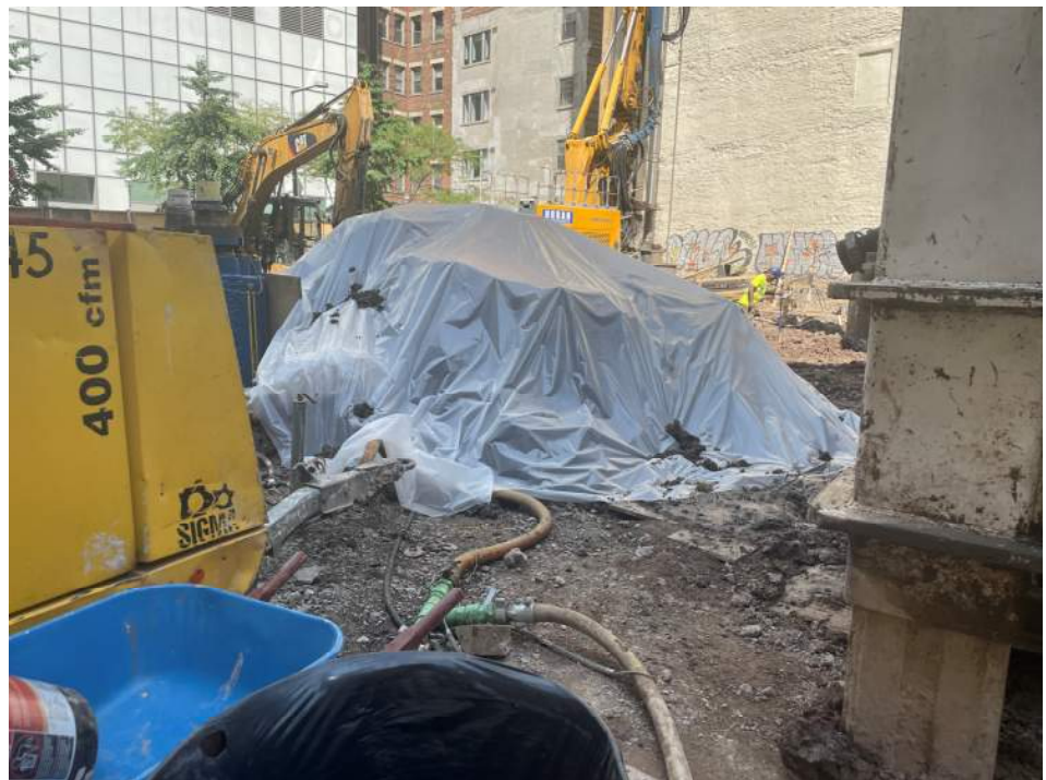
Photo 2: Stockpile covered with polyethylene sheeting at the end of the work day in the central part of waste characterization grid WC02 (facing northeast).
