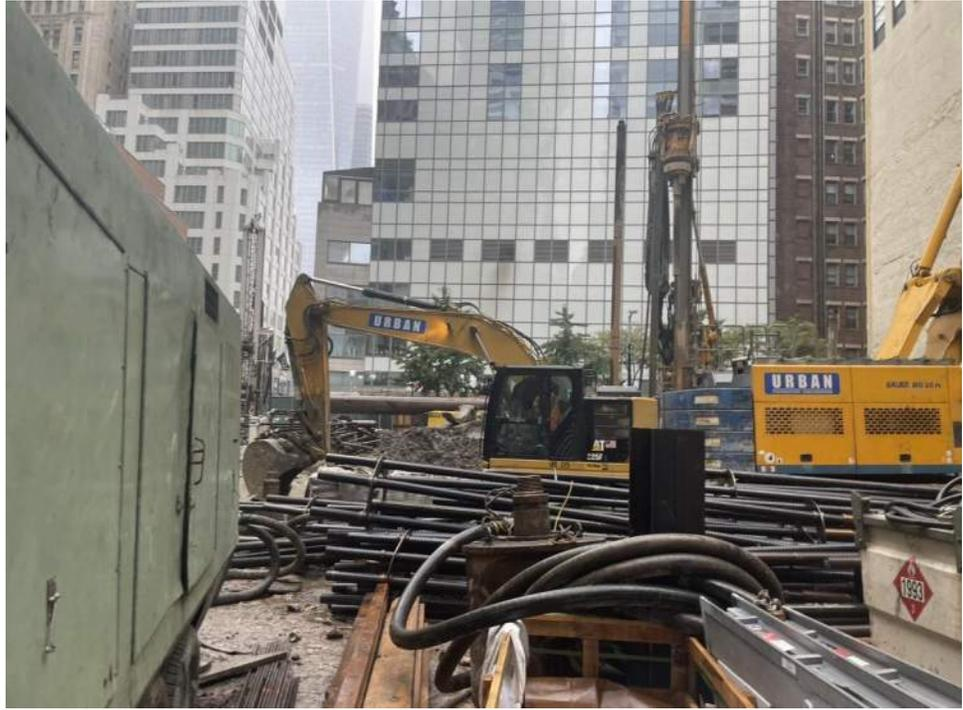
**Photo 2:** View of Urban replacing the geotextile fabric (facing northeast).
