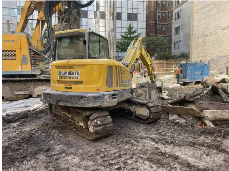
Photo 1: View of Urban excavating soil/fill in WC03 (facing northeast).
