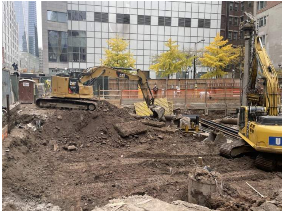
Photo 2: View of Urban excavating soil/fill in WC02_0-5 (facing north).
