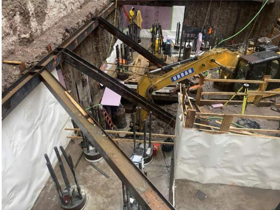
**Photo 2:** View of Urban loading a truck with soil/fill for off-site disposal (facing southeast).
