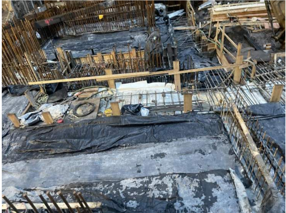
Photo 1: General view of the site (facing south).
