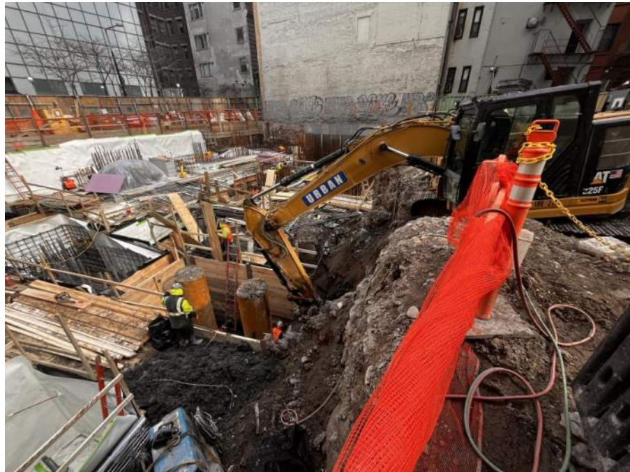
Photo 2: Urban excavating soil/fill in grid WC02 (facing east).
