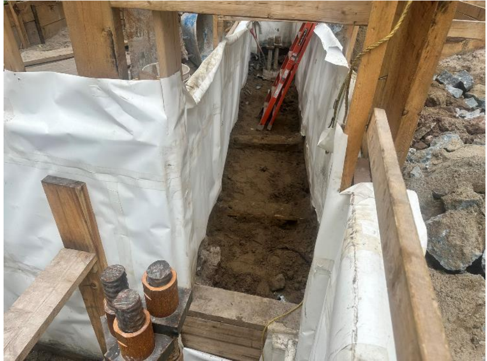
Photo 1: View of excavation area in the southern part of the site (facing south).
