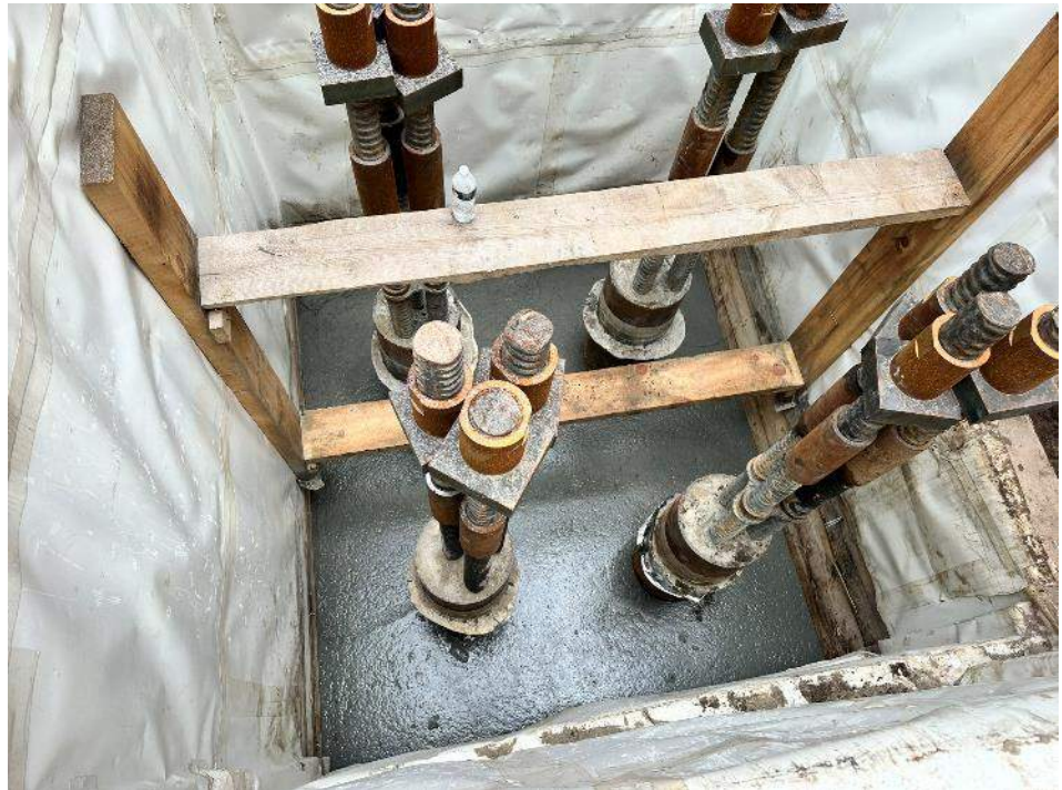
Photo 2: View of the poured concrete in the southern part of the site for waterproofing installation (facing east).
