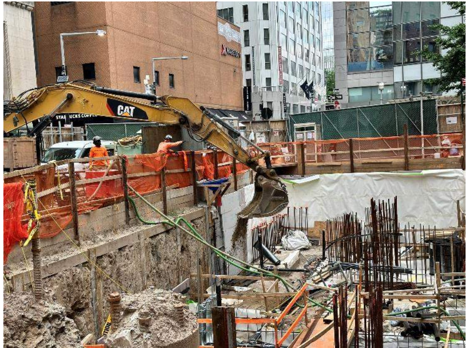
Photo 2: View of Urban backfilling in WC02 (facing northwest).
