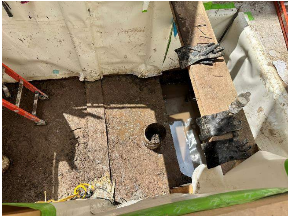
Photo 2: View of excavated area in the southwestern area of the site (facing south).
